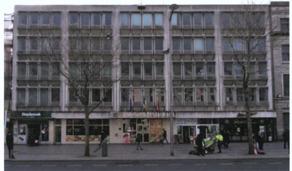
Plate 1: Front façade, number 45 O’Connell Street Upper
