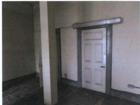
Plate 80: S-4 – View to south-west
