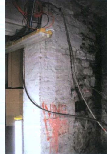
Plate 17: B-2 – View to north-west; mix of brick and Calp limestone
