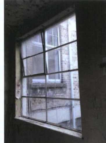
Plate 48: F-1 - View to north-east; steel pivot window
