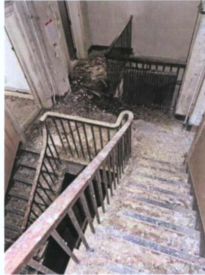
Plate 54: F-1 – View to south
