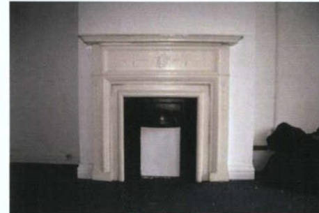
Plate 100: S-3 – Original cast-iron chimney piece to north
