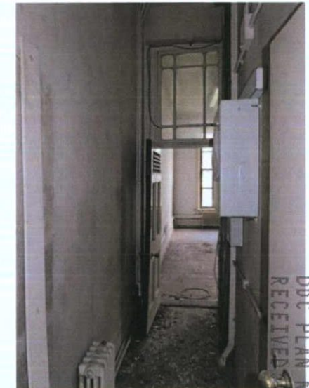
Plate 60: F-3 – View to east
