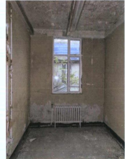
Plate 68: F-7 – View to west
