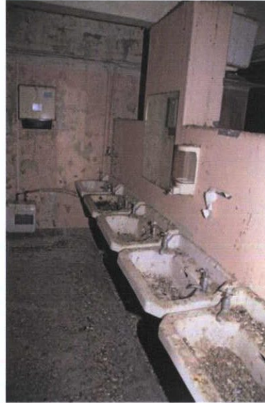
Plate 27: B-12 – View to west
