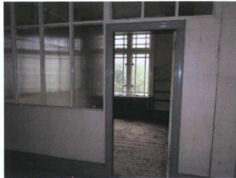
Plate 81: S-5 – Entrance to front room; non-original partition
