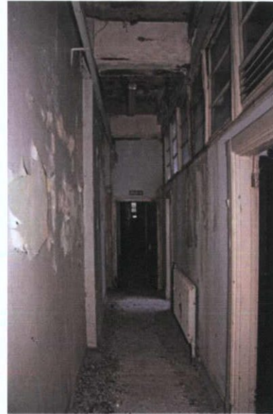
Plate 46: G-11 – View to west
