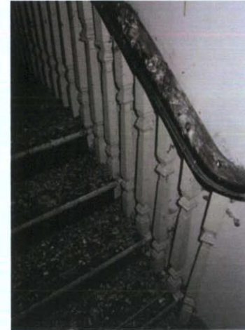
Plate 52: F-4 - Timber balustrade to staircase in main building; first floor staircase cut off from ground floor access
