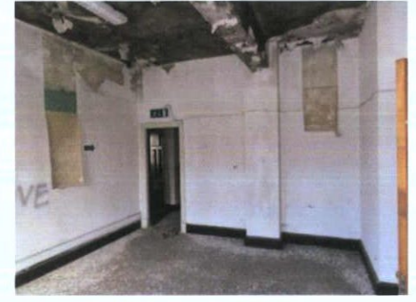
Plate 82: S-3 – View to east
