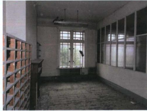
Plate 76: S-4 – View to east
