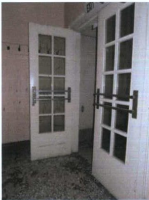
Plate 62: F-7 – View to south
