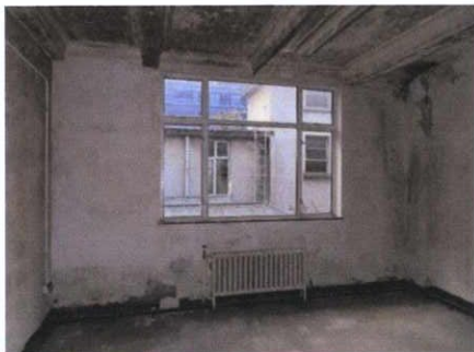
Plate 69: F-8 – View to west
