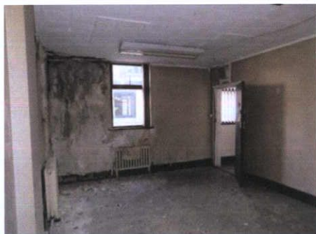
Plate 73: F-10 – View to east
