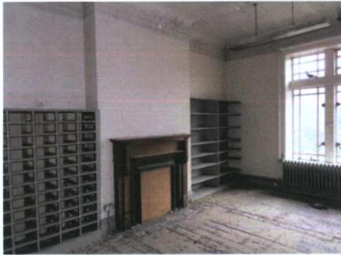
Plate 75: S-4 – View to north-west; original chimney piece
