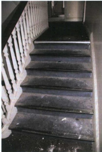
Plate 114: T-1 – View to east
