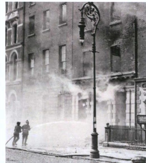
Figure 3: Fighting the fire at 44 Sackville Street Upper, July 1922
