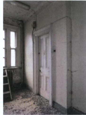
Plate 65: S-1 – Entrance to Room S-2
