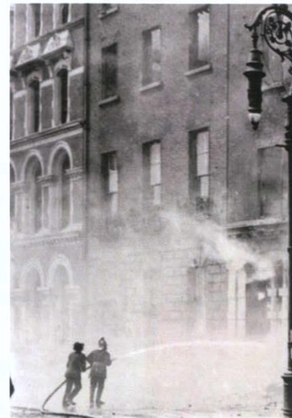
Figure 3: 45 O'Connell Street Upper gutted by fire
