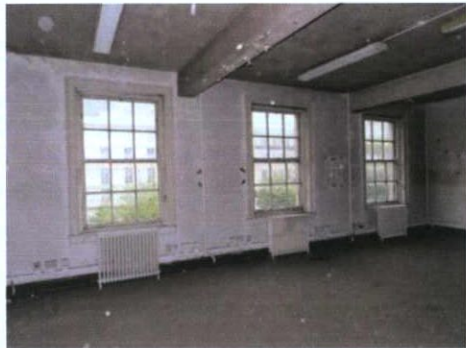
Plate 79: S-2 – View to south
