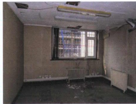
Plate 74: F-10 – View to west
