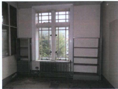
Plate 84: S-5 – View to east
