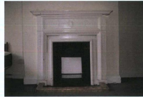
Plate 104: S-4 – Cast-iron chimney piece
