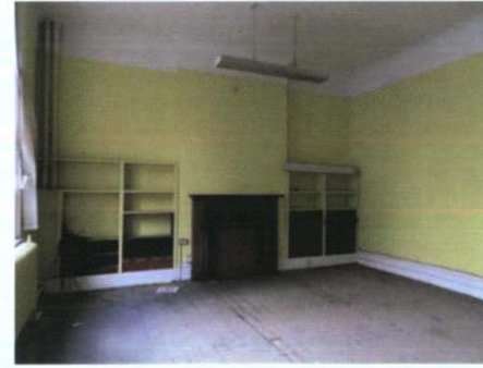
Plate 60: F-6 – View to north-east; original chimney piece
