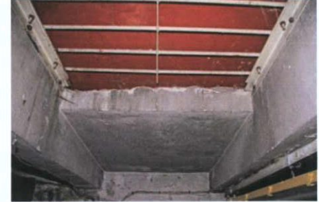
Plate 21: B-8 – View to ceiling intervention
