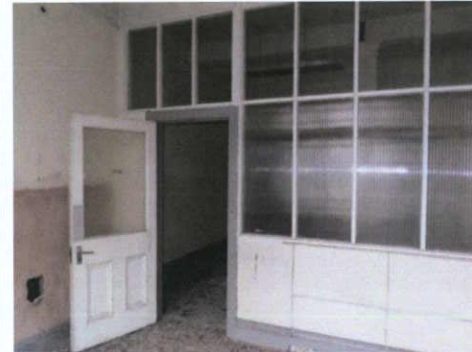
Plate 82: S-5 – View to south-west
