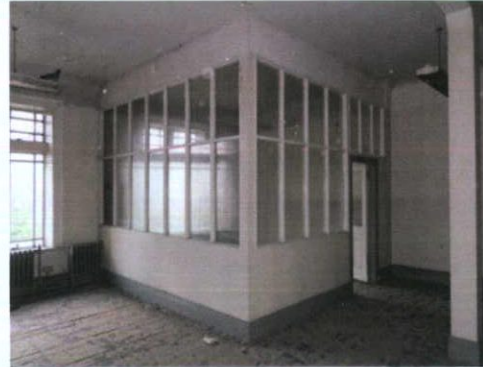
Plate 77: S-4 – View to south-east towards Room S-5; non-original subdivision of room
