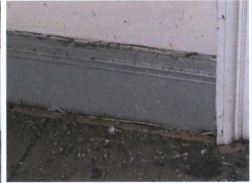
Plate 74: S-3 – Original skirting boards
