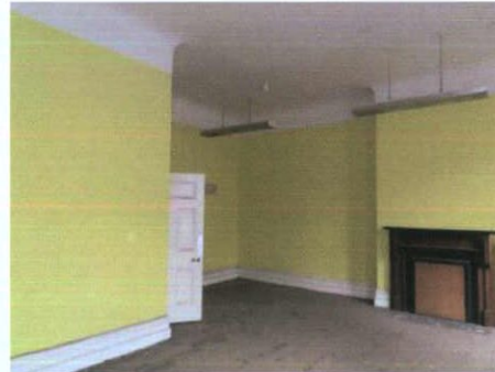
Plate 59: F-6 – View to north-west
