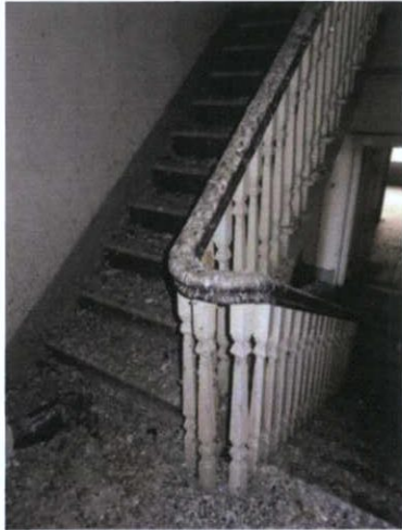
Plate 63: S-1 – View to east from half-landing
