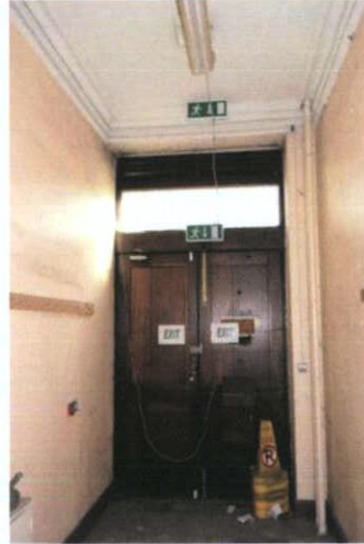
Plate 35: G-6 – View to east; non-original partition to north (left)
