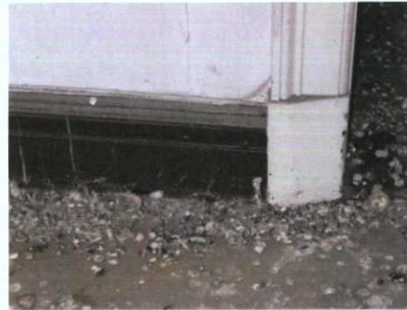
Plate 80: S-2 – Original skirting board
