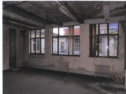
Plate 71: F-9 – View to west
