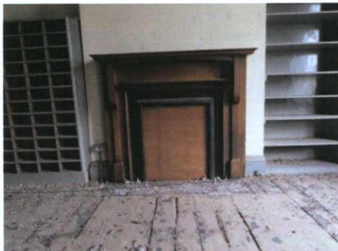
Plate 79: S-4 – Original timber chimney piece with cast-iron fire surround
