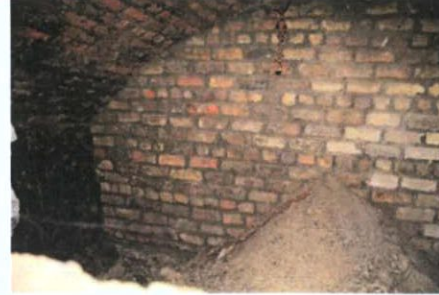
Plate 20: B-7 – View to east; brickwork rear of vault is later intervention
