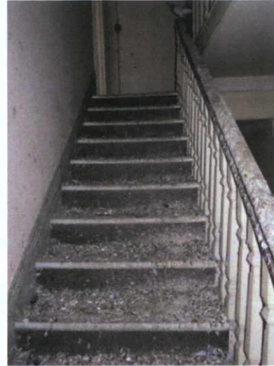
Plate 86: T-1 – View to east
