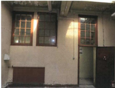
Plate 44: G-9 – View to north
