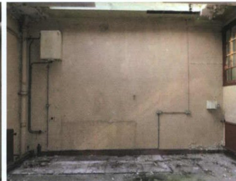
Plate 45: G-9 – View to west
