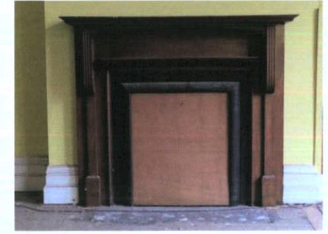
Plate 61: F-6 – Timber chimney piece with cast-iron insert
