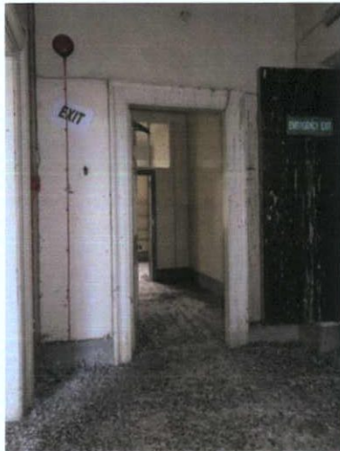
Plate 67: S-1 – View to east at first floor landing
