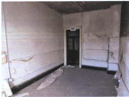
Plate 98: T-7 – View to east
