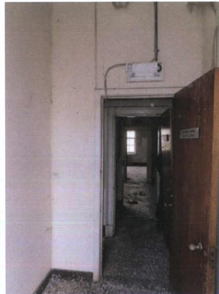
Plate 85: S-4 – View to east
