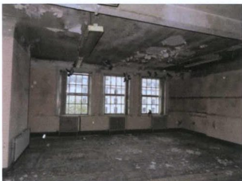
Plate 97: T-4 – View to east
