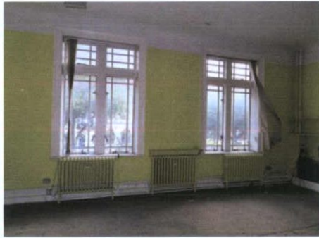
Plate 58: F-6 – View to east
