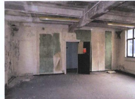
Plate 72: F-9 – View to south
