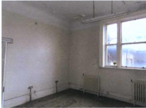
Plate 54: F-5 – View to south-west; Wyatt window
