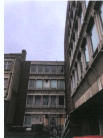
Plate 160: East side of car park — main building
