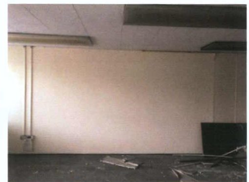
Plate 233: Room 2 — West wall
