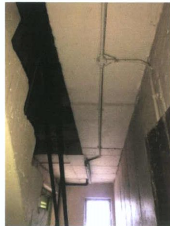
Plate 15: Ceiling of hallway
