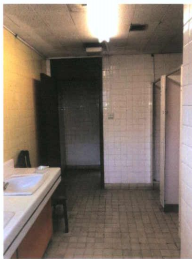
Plate 185: Exit from men's WC
