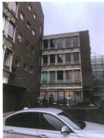
Plate 163: East side of car park — main building
