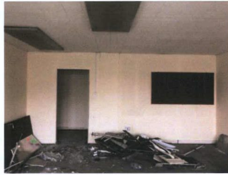
Plate 235: Room 2 — North wall
