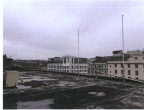
Plate 12: East roof — East 3
