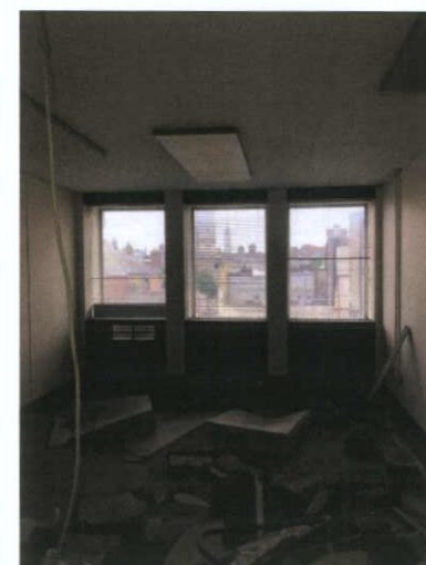
Plate 281: Room 15 — North wall
