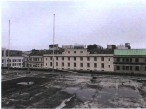
Plate 11: East roof — East 2
