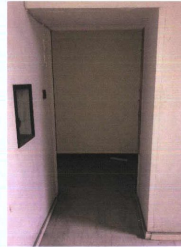
Plate 304: Entrance doorway onto level 3 from west stairwell
