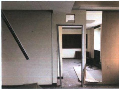
Plate 336: Room 1 — West wall
