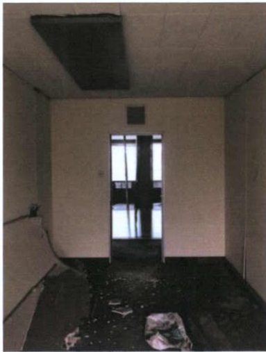
Plate 266: Room 11 — South wall
