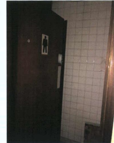
Plate 285: Male WC entrance from main hallway
