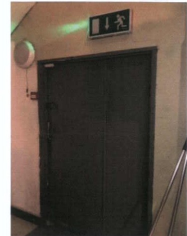
Plate 52: Emergency exit to car park
