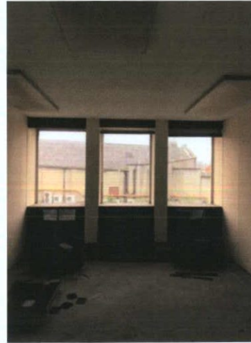
Plate 256: Room 9 — South wall
