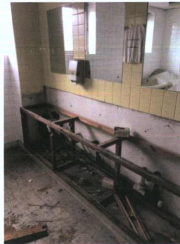
Plate 287: Male WC — West wall demolished wash hand basins
