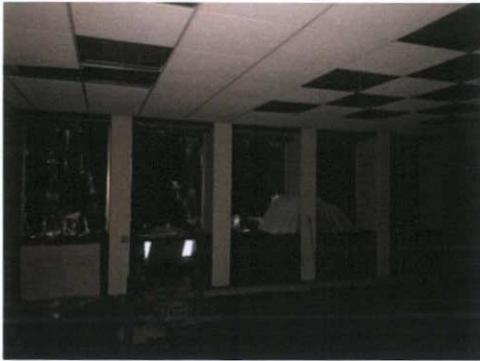
Plate 226: Room 1 — South wall
