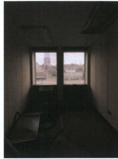
Plate 268: Room 12 — South wall
