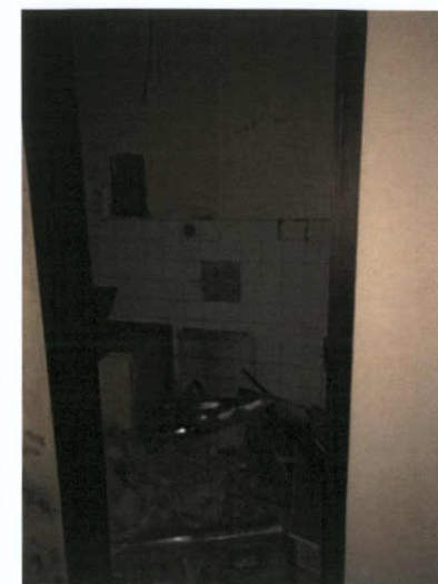
Plate 293: Doorway of cleaning closet
