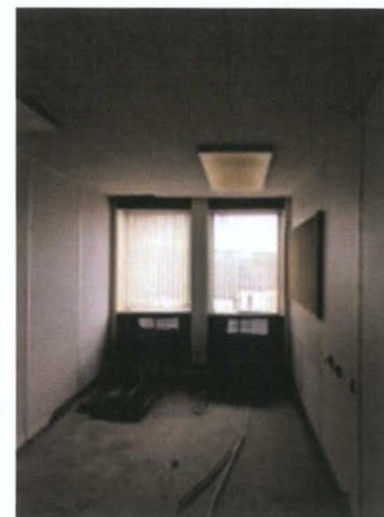
Plate 362: Room 7 — South wall
