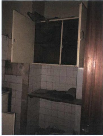
Plate 298: East wall of kitchenette
