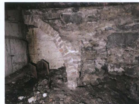
Plate 41: Vault and masonry in basement
