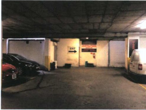
Plate 92: West wall at rear of car park
