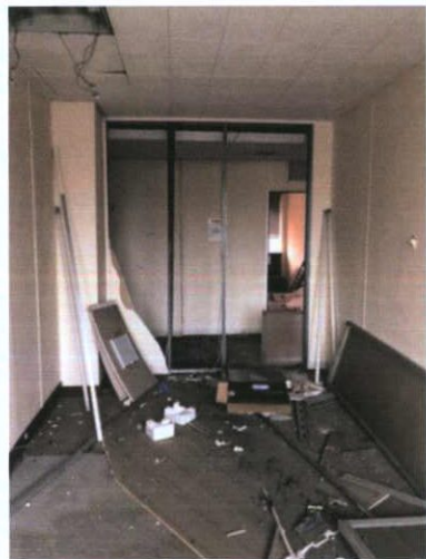
Plate 270: Room 12 — North wall
