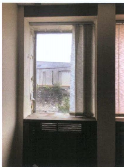
Plate 206: Window in office
