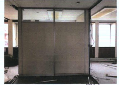
Plate 339: Room 2 — North wall
