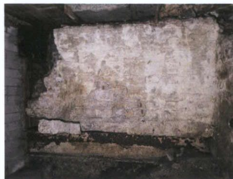
Plate 40: Limewashed wall in basement
