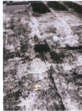
Plate 12: East roof — Drain
