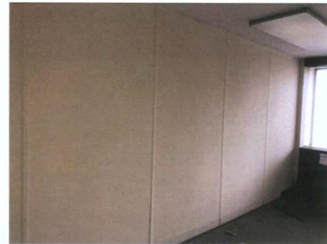
Plate 247: Room 7 — West wall
