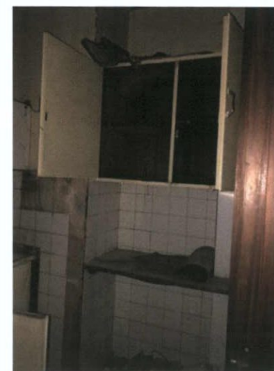
Plate 297: East wall of kitchenette
