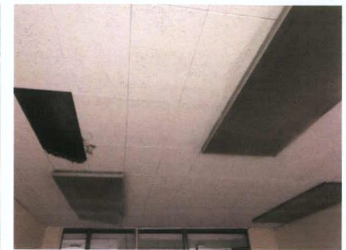
Plate 245: Room 6 — Suspended ceiling
