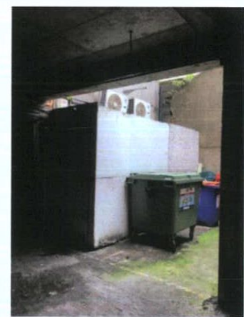
Plate 99: Waste area in south east corner
