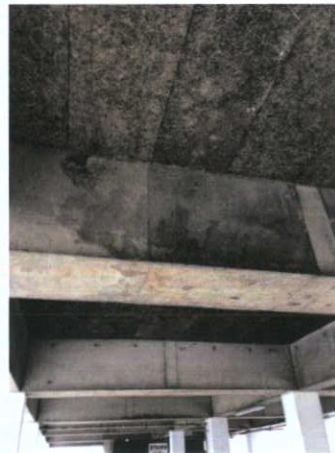
Plate 171: Car park ceiling
