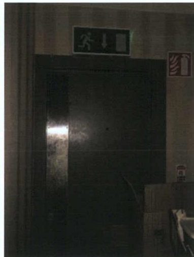
Plate 136: Fire exit door
