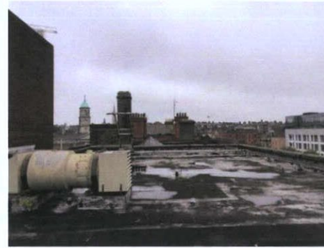
Plate 12: East roof — North
