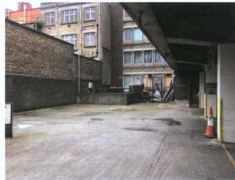
Plate 156: North boundary wall connecting to main building
