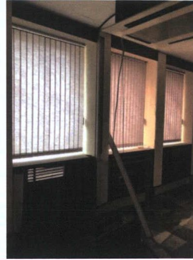
Plate 215: Windows on north wall with blind
