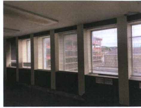
Plate 236: Room 3 — North wall
