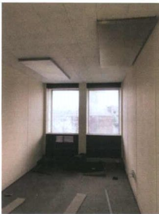
Plate 246: Room 7 — North wall
