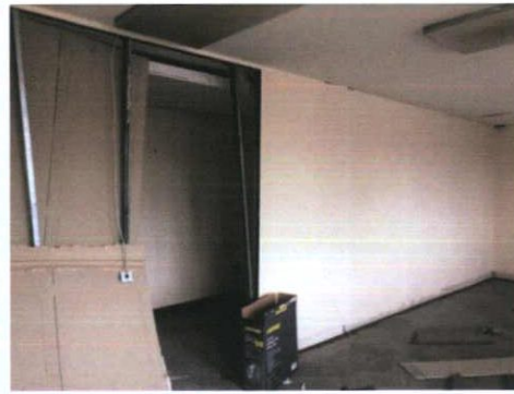
Plate 239: Room 3 — South wall
