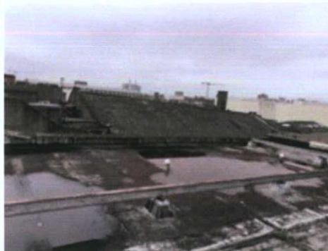
Plate 21: East roof — South 1
