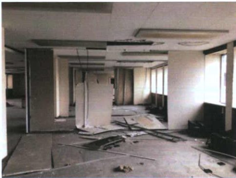
Plate 352: Room 5 — West wall
