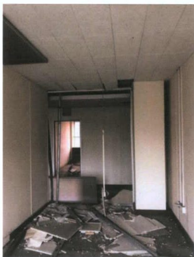
Plate 262: Room 10 — South wall
