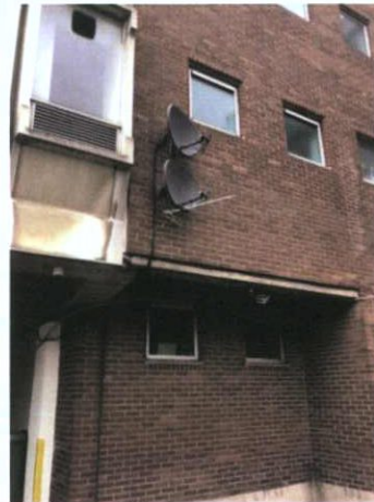
Plate 167: South west wall of west stair core
