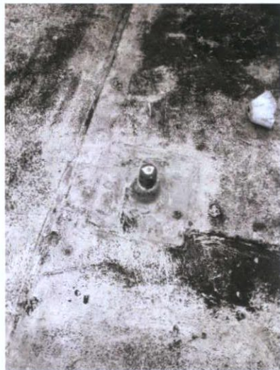
Plate 24: East roof — post for a fall arrest system wire
