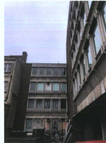
Plate 8: Rear of building view from car park — View to east
