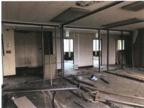
Plate 368: Rooms 8-12 — North wall
