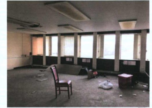
Plate 355: Room 6 — South wall
