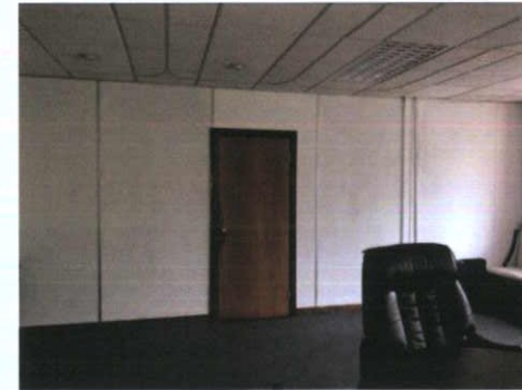
Plate 195: North wall of board room
