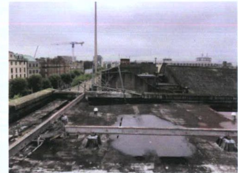
Plate 22: East roof — South 2
