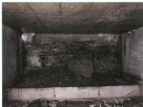
Plate 39: Limestone wall in basement
