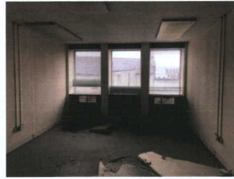
Plate 240: Room 5 — North wall
