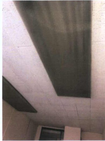
Plate 251: Room 7 — Ceiling detail
