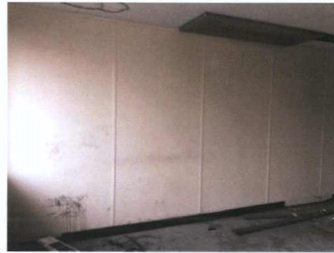
Plate 243: Room 6 — West wall
