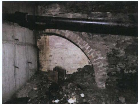
Plate 31: Rising walls and services in basement
