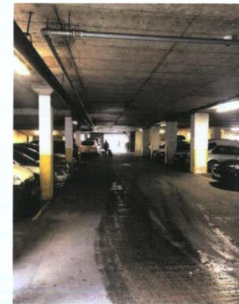
Plate 95: South corridor leading to exit on Moore Lane
