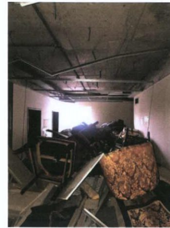
Plate 318: Lift lobby – North wall
