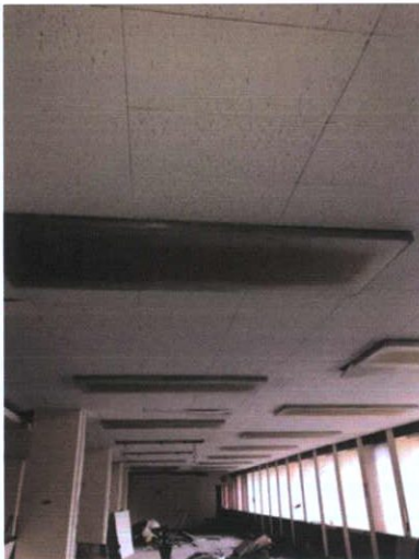
Plate 217: Typical suspended ceiling throughout floor
