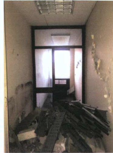
Plate 284: Room 16 — North wall — non accessible due to demolished materials
