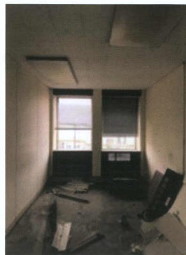
Plate 264: Room 11 — North wall
