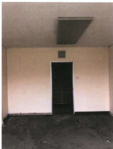
Plate 258: Room 9 — North wall
