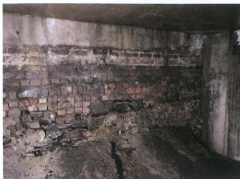
Plate 38: Brick and limestone wall in basement
