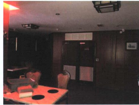
Plate 102: South wall — kitchen door
