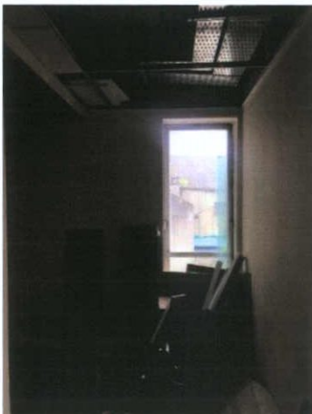
Plate 321: Corridor from lift lobby to main room
