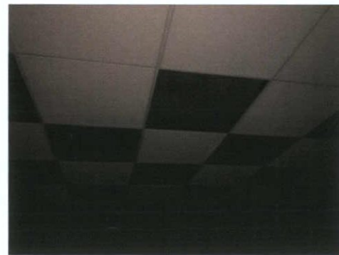
Plate 231: Ceiling panels removed
