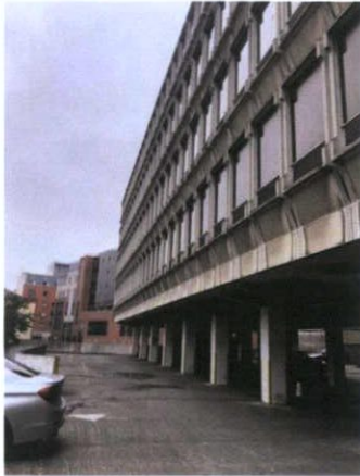
Plate 10: View from car park — View to west
