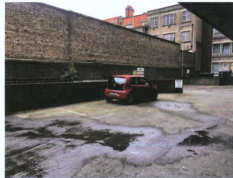
Plate 155: North boundary wall and entrance ramp
