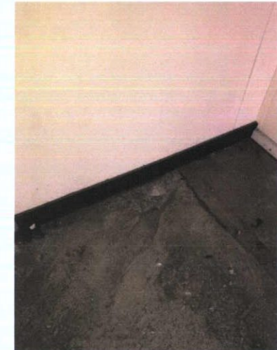
Plate 305: Carpet visible underneath metal stud partitions
