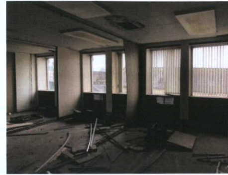
Plate 366: Rooms 8-12 — South wall
