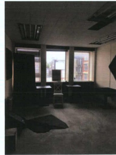
Plate 272: Room 13 — North wall
