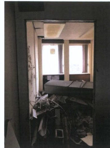
Plate 223: Inaccessible office to south of reception area
