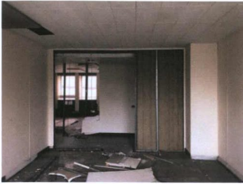
Plate 242: Room 6 — North wall
