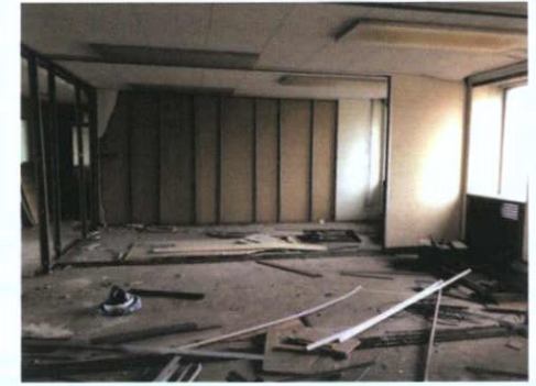
Plate 367: Rooms 8-12 — East wall
