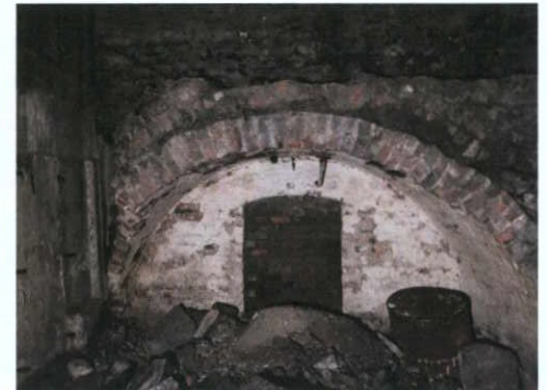
Plate 33: Broken end of brick vault
