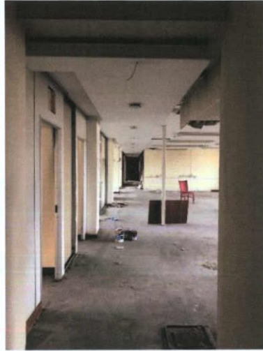
Plate 333: View from entrance to down main corridor
