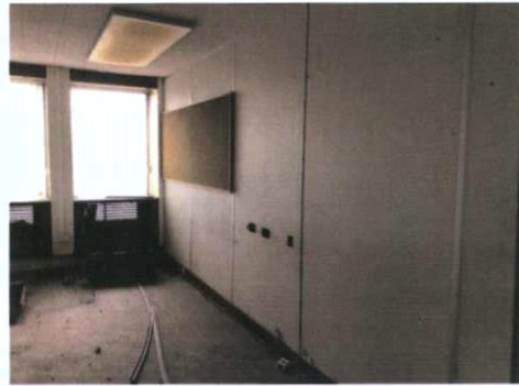
Plate 365: Room 7 — West wall
