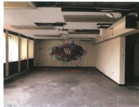
Plate 358: Room 6 — West wall
