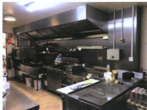
Plate 78: North wall of kitchen
