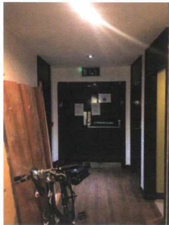
Plate 112: WC Hallways — fire exit leading to car park
