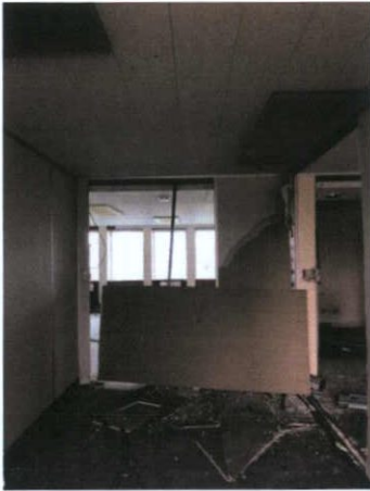
Plate 364: Room 7 — North wall
