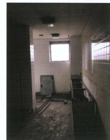
Plate 379: Men's WC wash area
