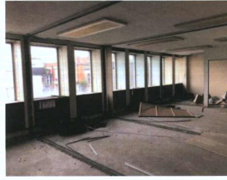
Plate 370: Rooms 13-16 — North wall
