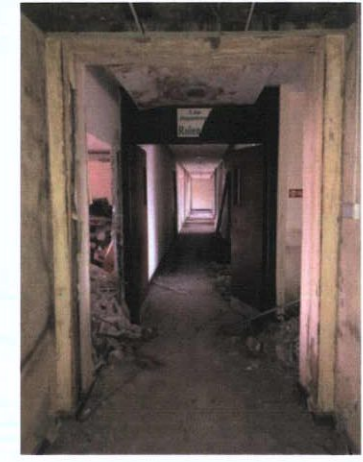
Plate 301: Main corridor facing west
