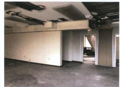
Plate 359: Room 6 — North wall
