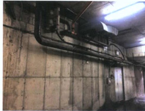
Plate 93: Building services on west wall
