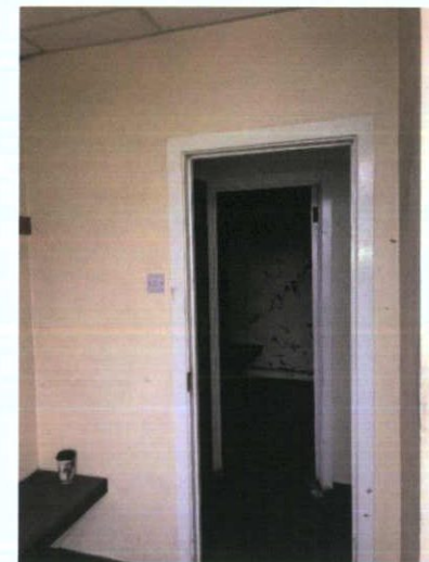
Plate 410: Room 3 — North Wall
