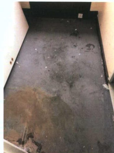
Plate 405: Room 1 — Concrete floor
