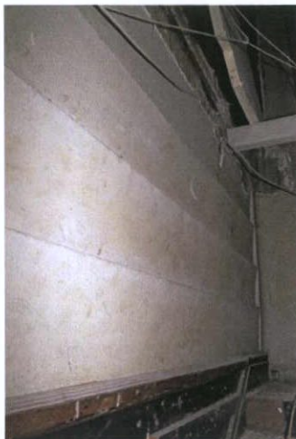
Plate 19: G-5 – Plaster to south wall arrow is NE
