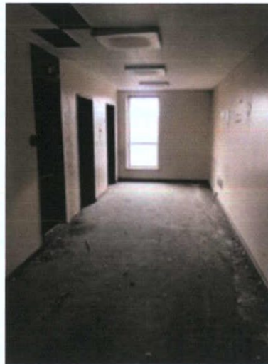
Plate 488: Lift lobby — North wall
