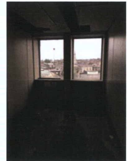
Plate 458: Room 13 — North wall
