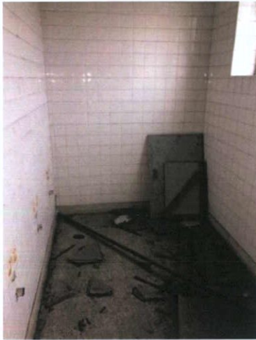
Plate 380: Men's WC urinal area
