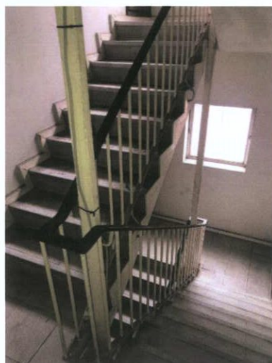
Plate 520: Typical stair flights and landings
