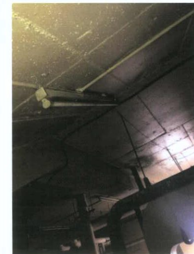
Plate 498: Plant room — Ceiling
