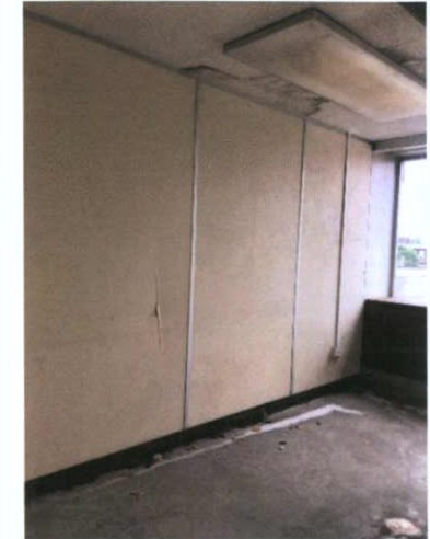
Plate 446: Room 11 — West wall
