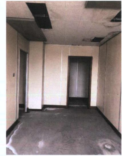
Plate 454: Room 12 — South wall
