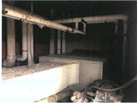
Plate 499: Plant room — South wall 1
