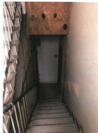
Plate 525: Stair down to level 1 landing
