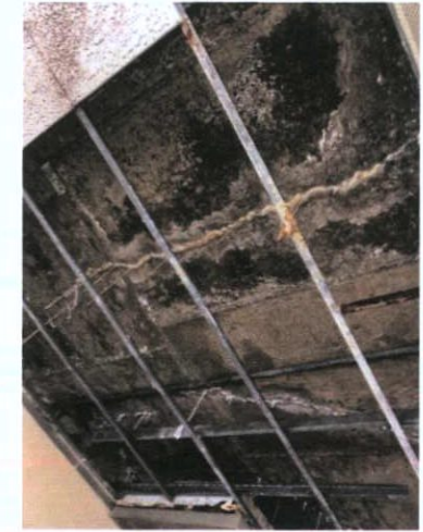
Plate 438: Room 9 — Suspended ceiling damage
