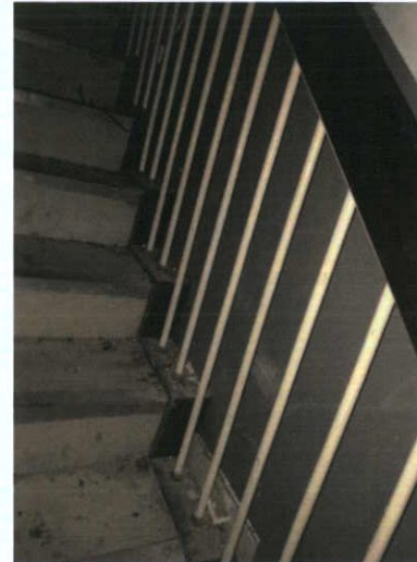
Plate 511: Stair baluster detail
