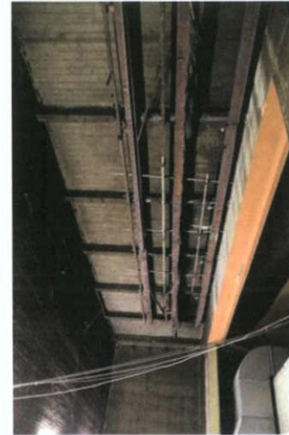
Plate 23: F-1 – View to north, ceiling over former stage
