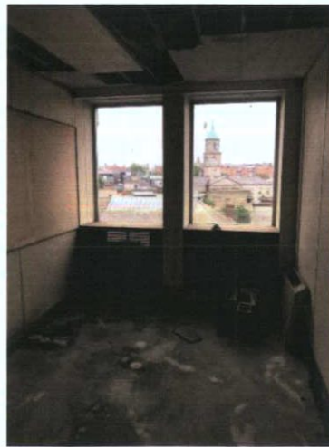
Plate 440: Room 10 — North wall
