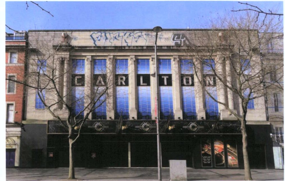
Plate 1: Front façade, Carlton Cinema, 52-54 O'Connell Street Upper
