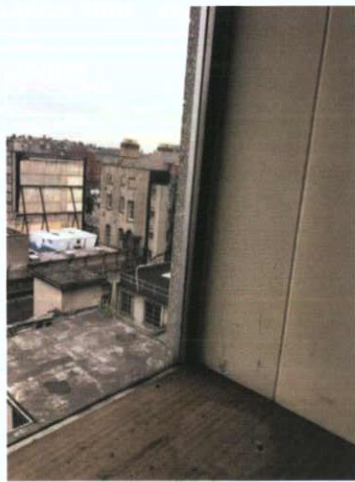
Plate 424: Room 7 — Window detail
