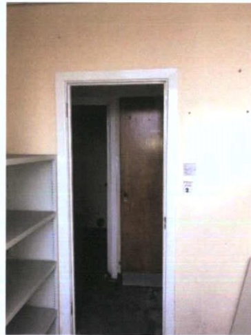
Plate 404: Room 1 — North wall
