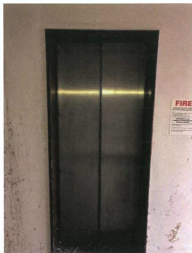
Plate 492: Lift lobby — Door 1
