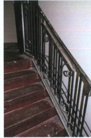
Plate 24: B-4 – View to north-east; original balustrade
