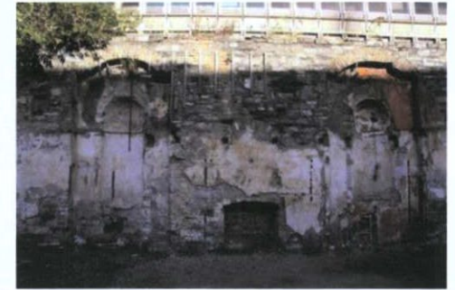
Plate 5: View to north; former chimney breast and flanking niches set into arches; formerly within Number 50
