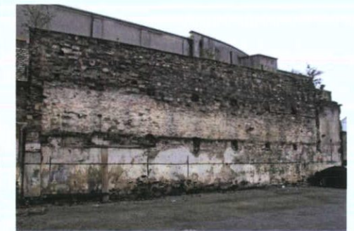
Plate 9: View to west; Calp limestone boundary wall
