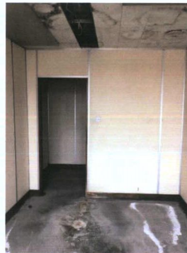
Plate 441: Room 10 — South wall
