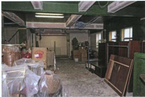
Plate 45: S-2 View to east
