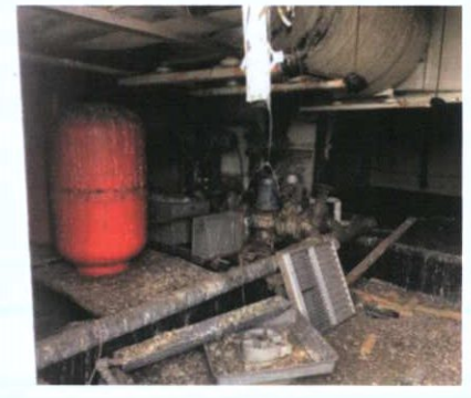
Plate 502: Plant room — North wall 2
