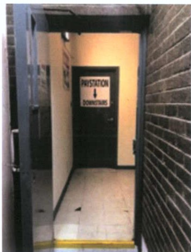
Plate 515: Access to stair at ground level
