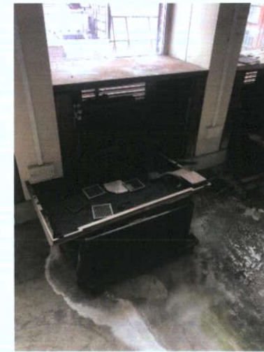
Plate 426: Room 7 — Ventilation units removed
