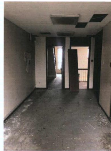
Plate 489: Lift lobby — South wall including east stairwell doorway and hallway to roofs
