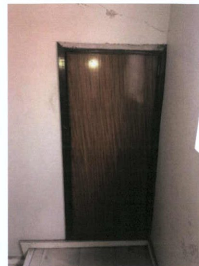
Plate 518: Access door to service riser
