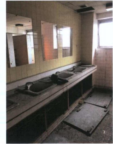
Plate 383: Women's WC wash area
