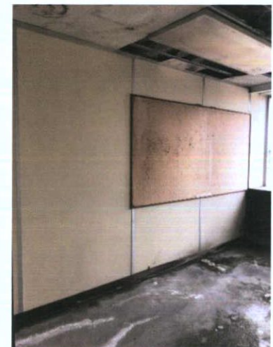
Plate 438: Room 9 — Suspended ceiling damage
