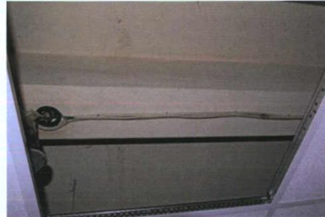
Plate 15: B-2 – Bressummers above false ceiling
