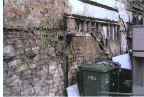
Plate 7: Red brick to north-east
