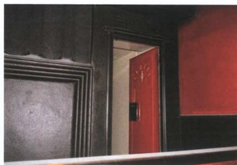
Plate 42: T-2 – Detail to doorway to south-east
