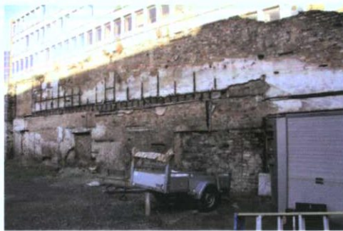
Plate 6: View to south-west; joist pockets in former party wall
