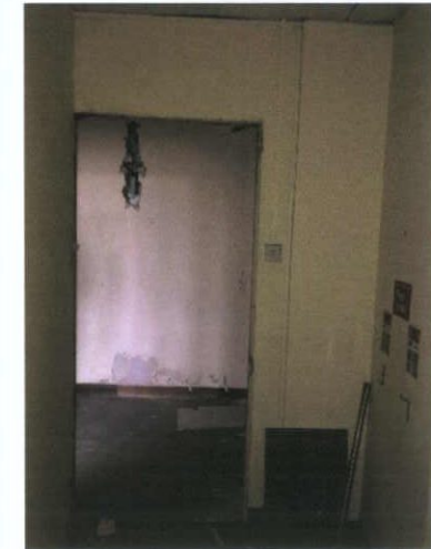
Plate 418: Room 6 — South wall
