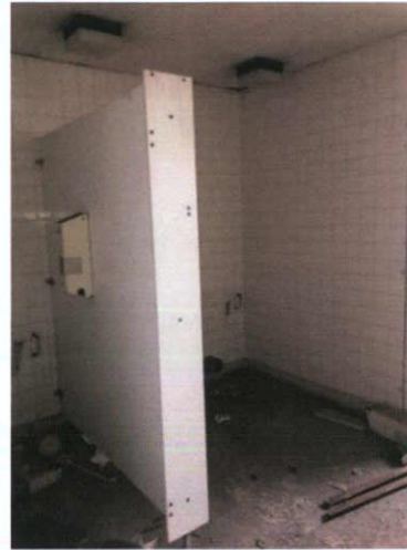
Plate 381: Men's WC cubicle area
