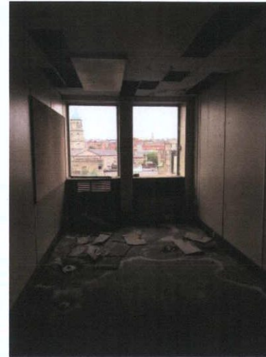
Plate 453: Room 12 — North wall
