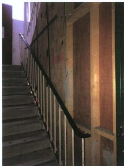
Plate 516: Stair wall to block upper levels
