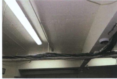
Plate 19: B-3 – Concrete structural bresssummers and cast concrete floor
