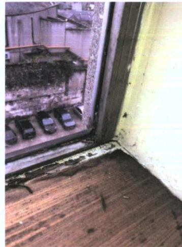
Plate 473: Room 16 — Window detail
