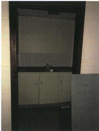
Plate 487: Kitchenette — North way / doorway
