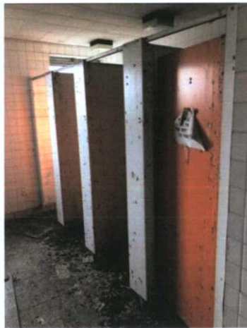
Plate 384: Women's WC cubicles
