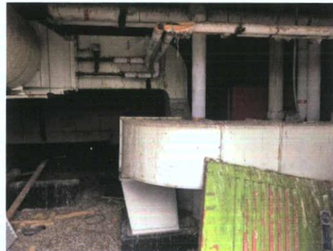
Plate 504: Plant room — East wall
