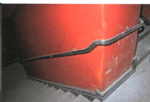
Plate 49: T-5 – Handrail on staircase
