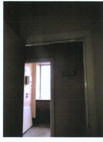
Plate 408: Room 2 — South wall
