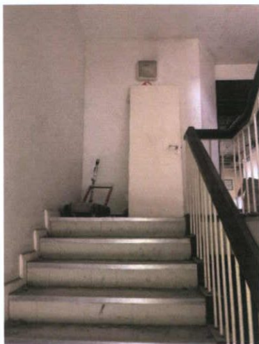
Plate 513: Fourth floor landing
