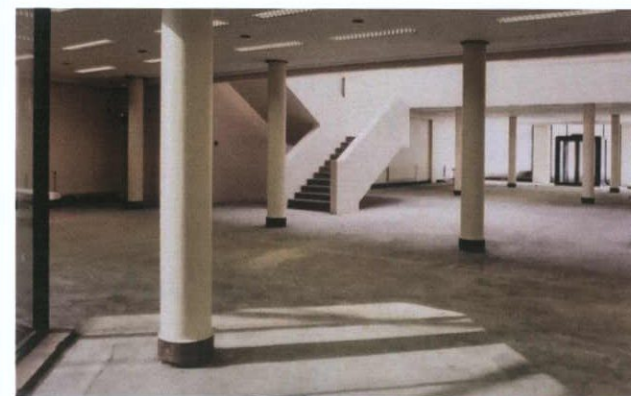
Figure 4: Interior of ground floor, 1988 (Irish Architectural Archive)
