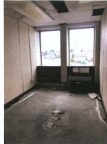
Plate 445: Room 11 — North wall
