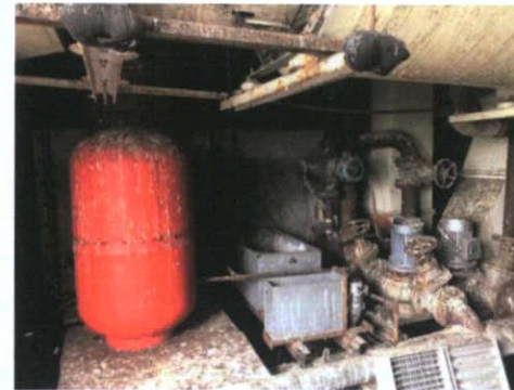
Plate 501: Plant room — North wall 1
