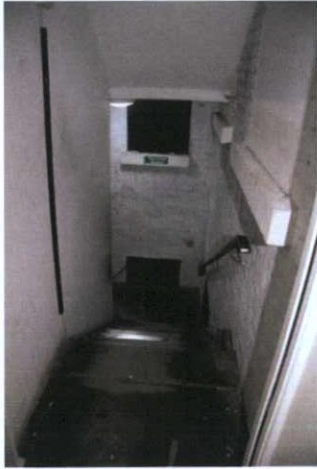
Plate 30: G-1 - View down stairway
