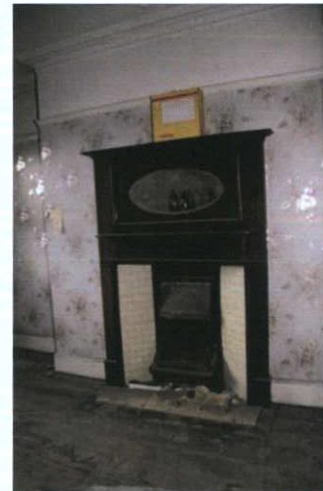
Plate 121: T-7 – View to north
