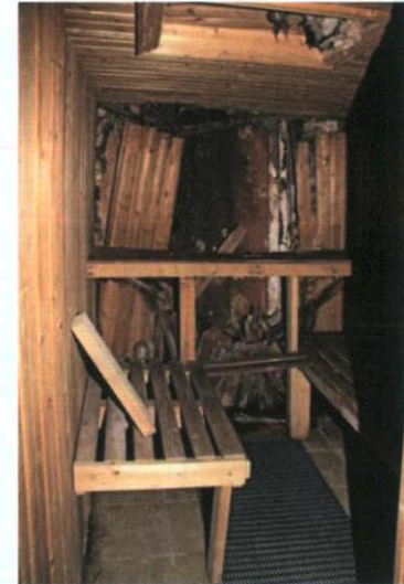
Plate 17: B-3 – View to east
