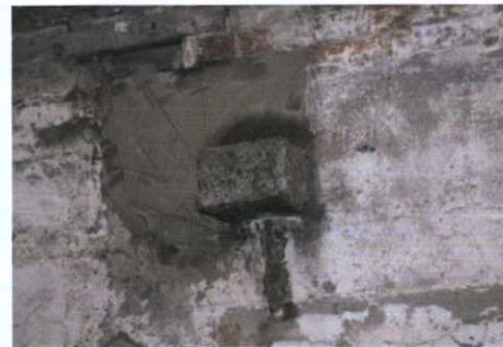
Plate 39: G-3: Granite corbel in southern wall
