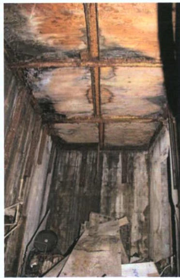
Plate 22: B-6 – Steel supports to ceiling
