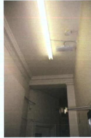
Plate 47: F-3 – Coving over central corridor
