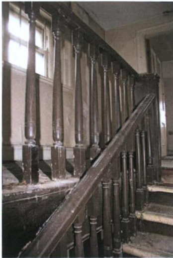
Plate 98: FO-1 – Detail to balustrade to fourth floor landing
