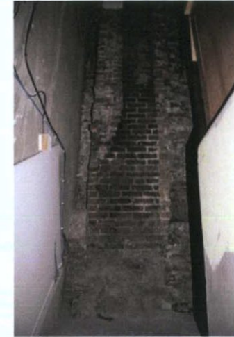
Plate 28: B-8 – View to south towards party wall
