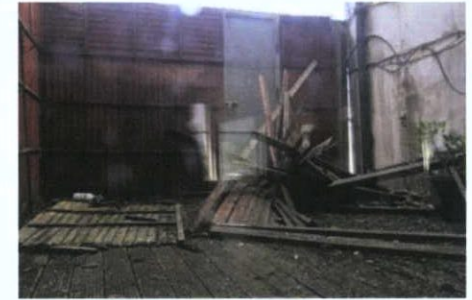
Plate 53: F-2 – View over rear extension from west window
