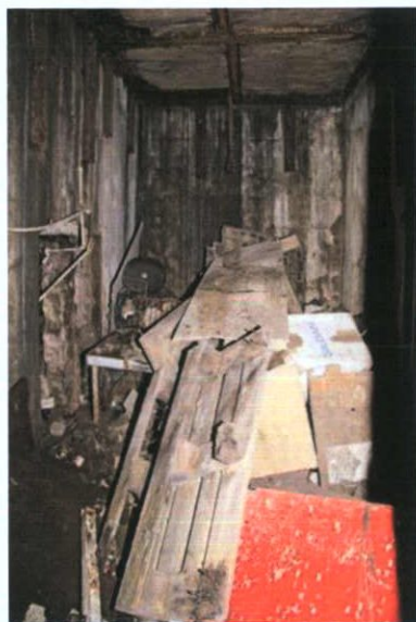
Plate 21: B-6 – View to south
