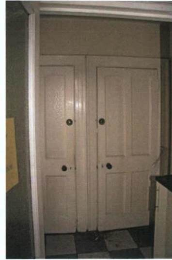
Plate 60: S-2 – View to west
