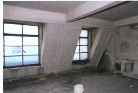
Plate 57: FO-2 – View to south-east
