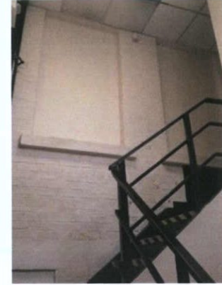
Plate 44: F-1 – Window at high level to east
