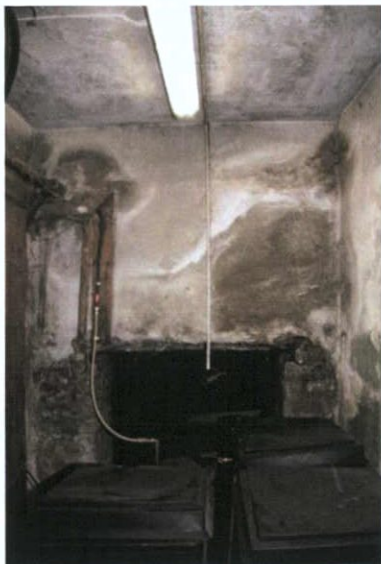
Plate 17: B-4 – View to east
