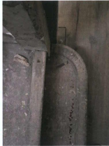
Plate 53: FO-1 – Curved timber step to half-landing
