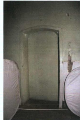
Plate 113: T-4 – View to south
