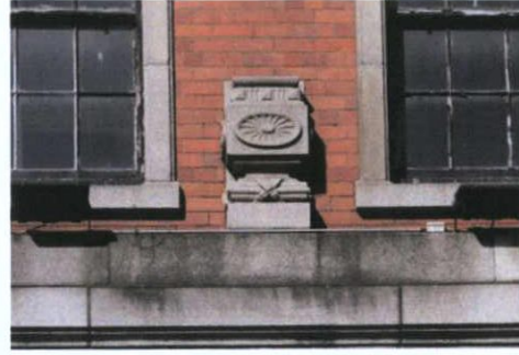
Plate 4: Limestone bracket
