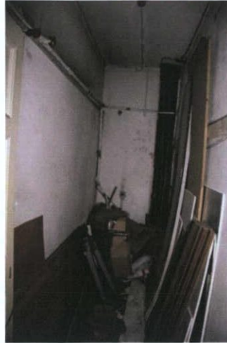
Plate 124: T-8 – View to north
