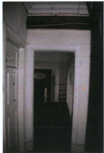
Plate 91: View into Room S-8 to north
