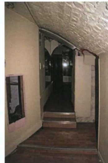
Plate 21: B-5 – View to east
