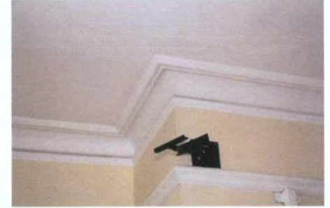
Plate 69: S-3 – Detail to coving to south chimney breast
