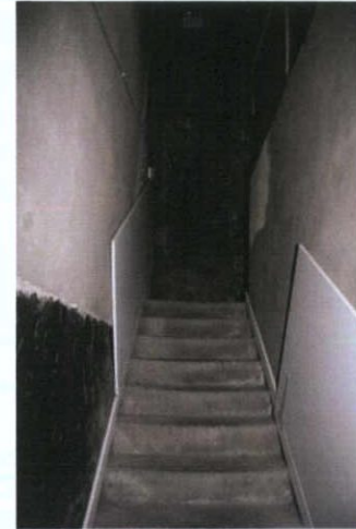
Plate 27: B-8 – View to south
