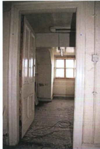
Plate 99: FO-1 – View to east into Room FO-5
