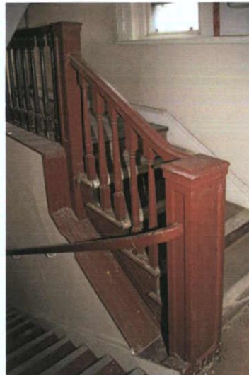
Plate 79: T-1 – View to north-west; original balustrade design resumes from third floor landing to fourth floor
