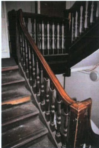
Plate 69: F-9 – View to south-west
