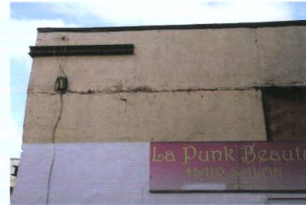
Plate 8: Former slit window, now blocked-up, noted to first floor to south elevation
