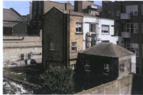
Plate 11: View of return and extension from south-west
