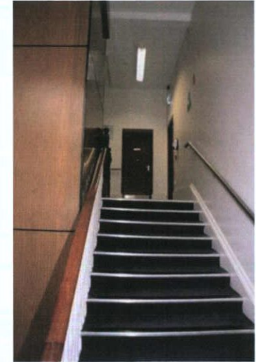
Plate 124: S-1 – View to east towards second floor landing
