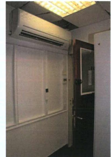
Plate 136: S-6 – View to north-west
