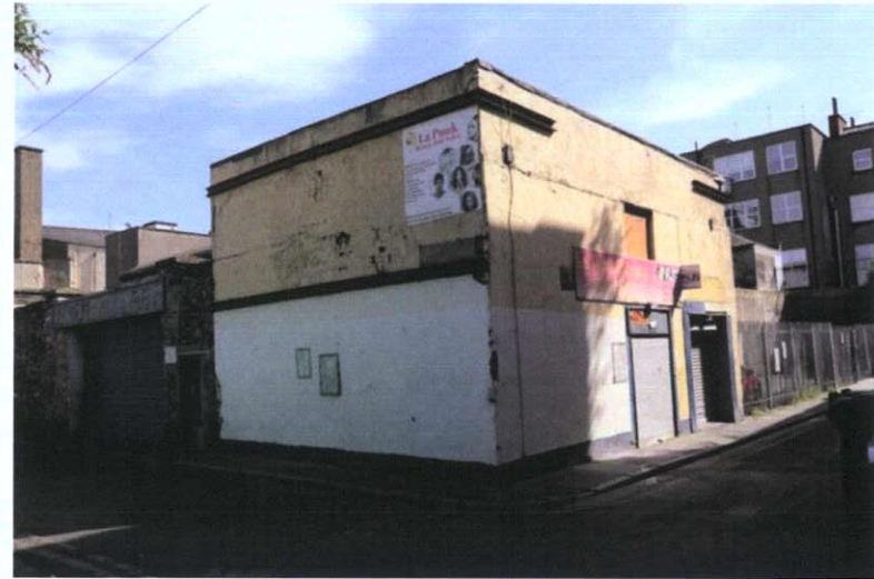
Plate 1: Exterior of 60A O'Connell Street Upper
