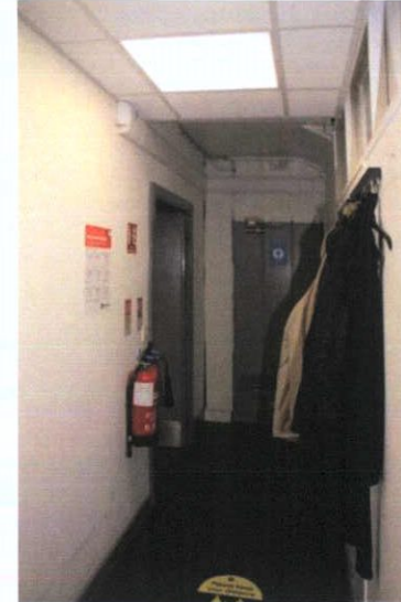
Plate 28: B-2 – View to east towards entrance to Room B-1
