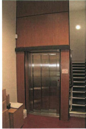
Plate 75: G-2 – View to west
