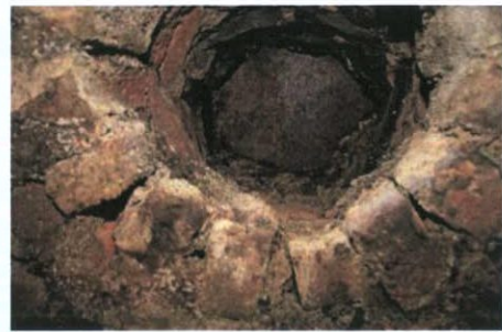
Plate 12: B-2 - Coal hole to soffit of vault
