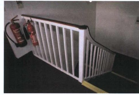
Plate 171: T-9 – Detail to balustrade
