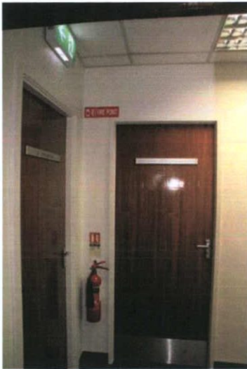
Plate 157: T-3 – View to east
