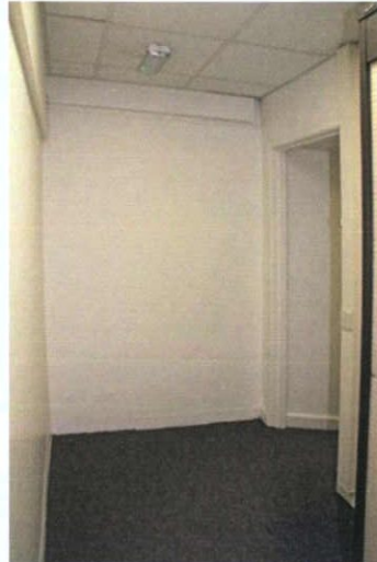
Plate 138: S-5 – View to east
