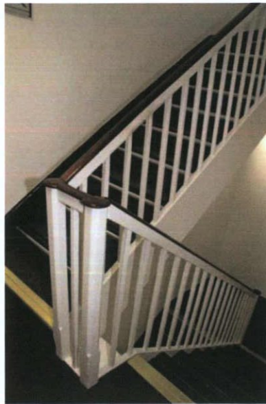
Plate 118: F-9 – View to north-west
