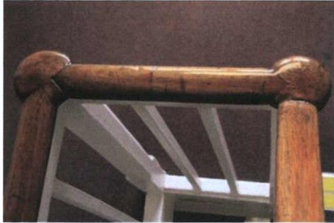
Plate 169: T-9 – Detail to balustrade
