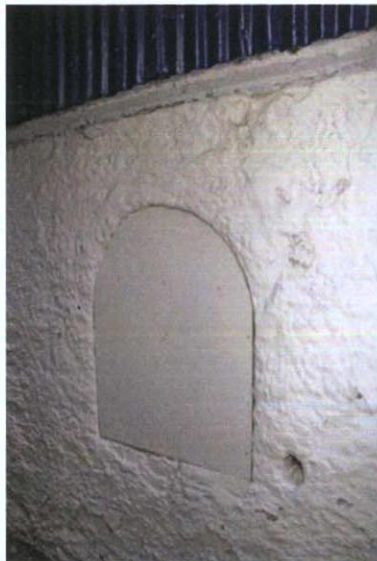
Plate 62: B-15 – Round-headed opening, now blind, to west
