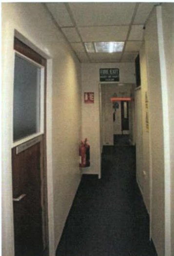
Plate 161: T-5 – View to south
