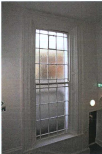
Plate 125: S-1 – View to west
