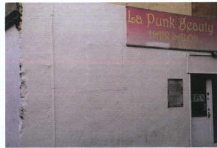
Plate 7: Ghost mark of former window opening
