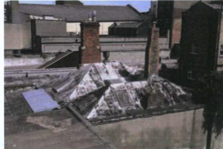
Plate 23: View to extension from south-west
