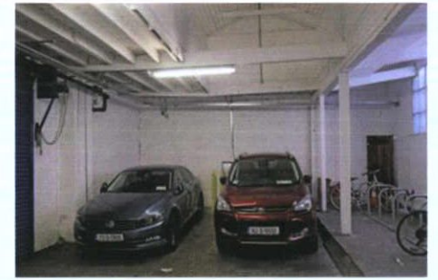
Plate 89: G-11 – View to north
