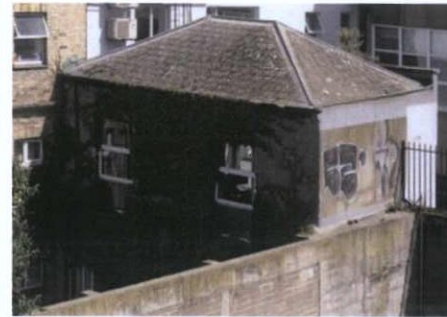
Plate 12: View of extension from south-west
