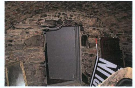
Plate 15: B-3 - View to west
