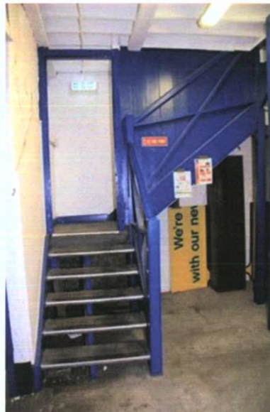
Plate 63: B-16 – View to west
