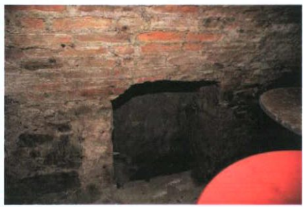
Plate 13: B-2 - View to north towards Room B-3
