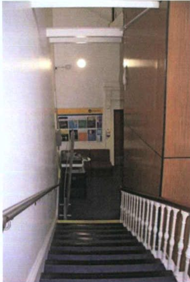
Plate 97: F-1 – View to east towards first floor
