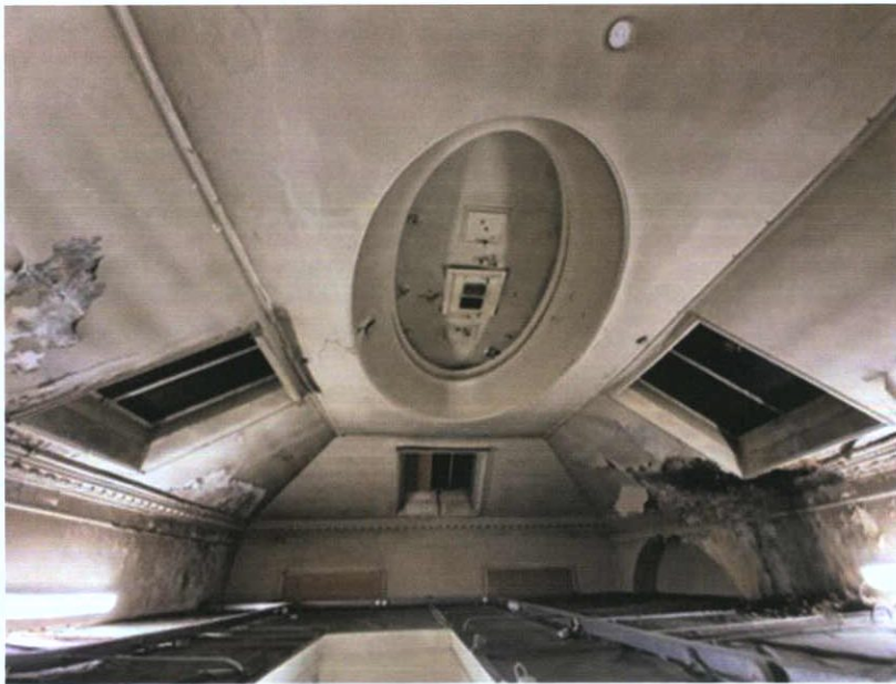
Plate 94: G-13 – Original ceiling over suspended ceiling in Reading Room
