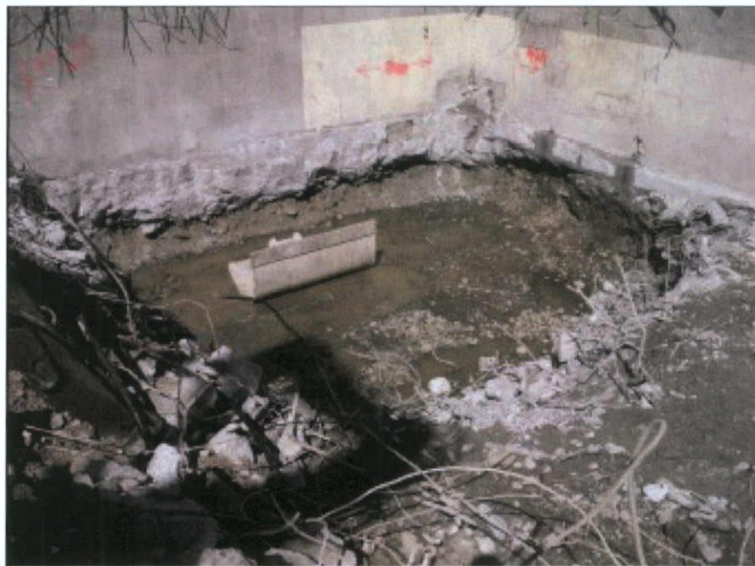
Figure 27 Trench 4, temporary crane base
