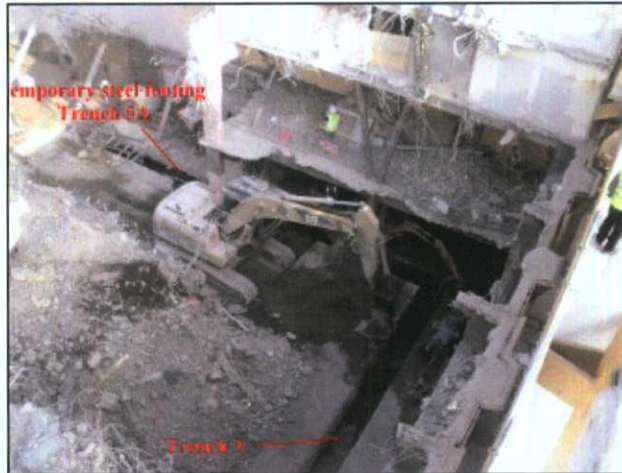
Figure 23 Overview of steel footing trench
