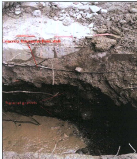
Figure 25 Trench B, concrete and natural gravels
