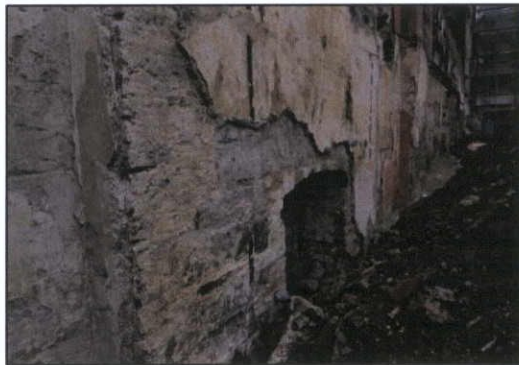
Figure 76 Projecting chimney breast
