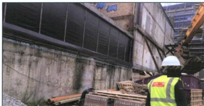
Figure 66 The south wall, west end
