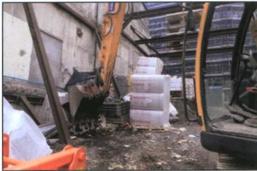
Figure 43 Trench 5, from the east
