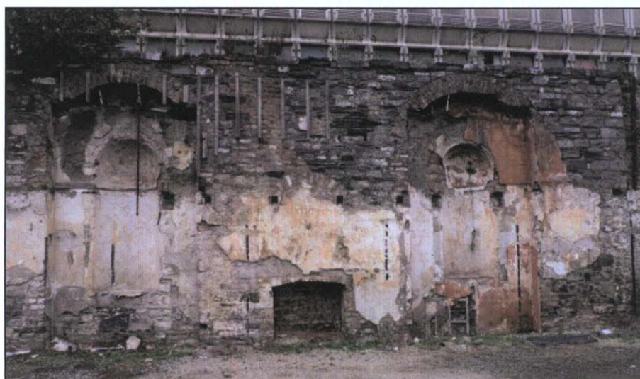
Figure 74 Building 2, from the south
