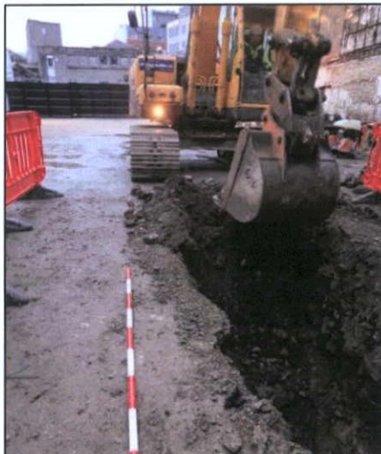
Figure 45 Trench 1, from the east
