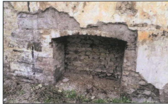
Figure 77 The fireplace in Room 2: type 3 brick
