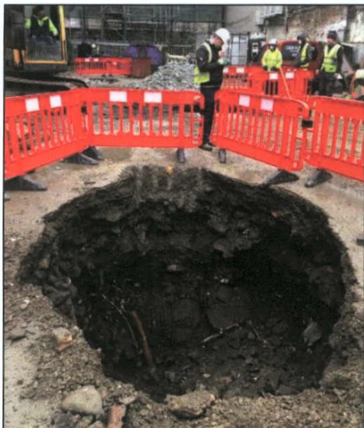
Figure 53 The expanding trench
