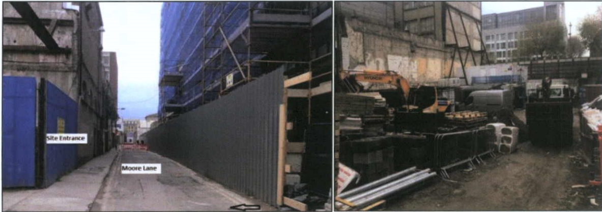
Figure 30 The site entrance (Site A) Figure 31 Site A, looking to the east
