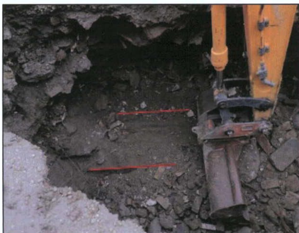
Figure 60 The structure from the north
