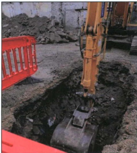
Figure 51 Trench 2 from the south
