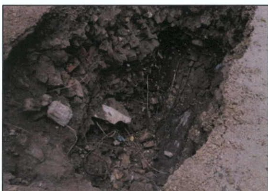
Figure 57 The floor abutting the wall foundation
