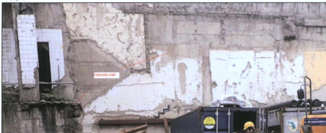
Figure 63 The north wall
