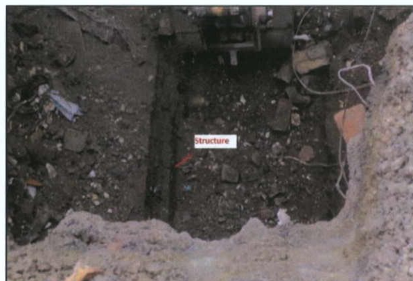
Figure 58 Foundation from the east
