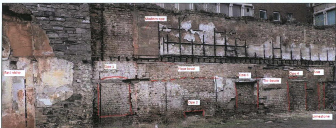
Figure 83 Building 3, from the west
