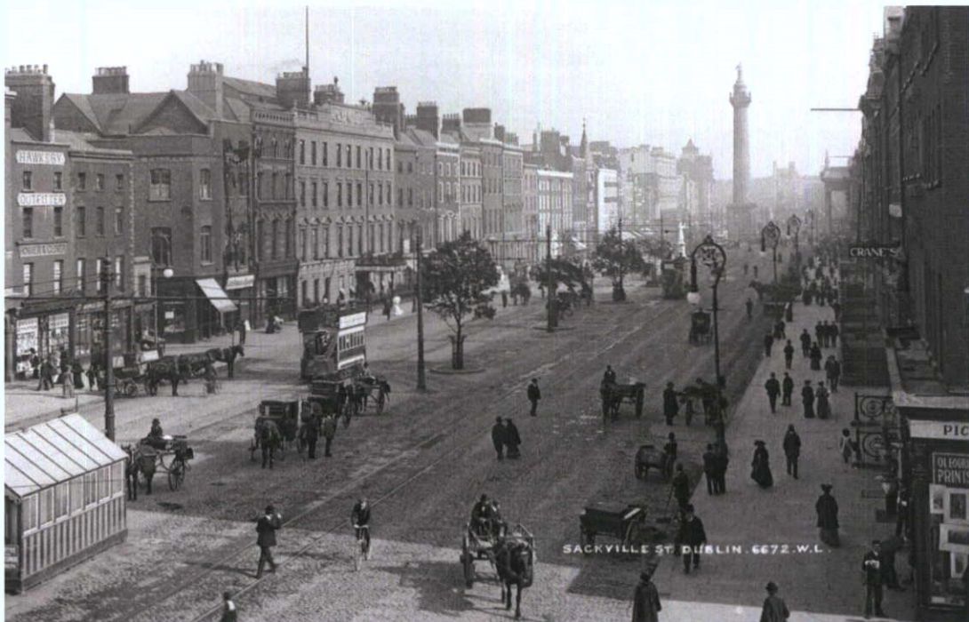
Figure 12.7: View of the north end of Sackville Street c. 1900. The Gresham Hotel is seen to the left.
