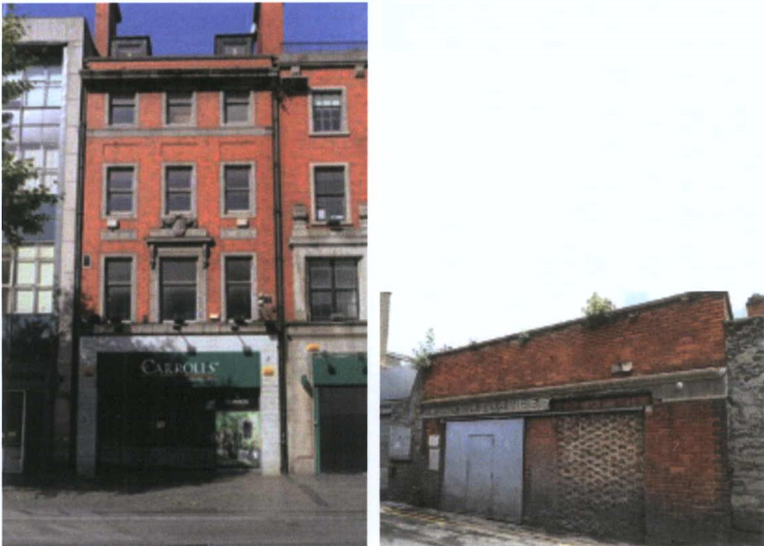
Plate 15.3.9 Front façade of No.58 O'Connell Street Upper and rear elevations on Moore Lane
