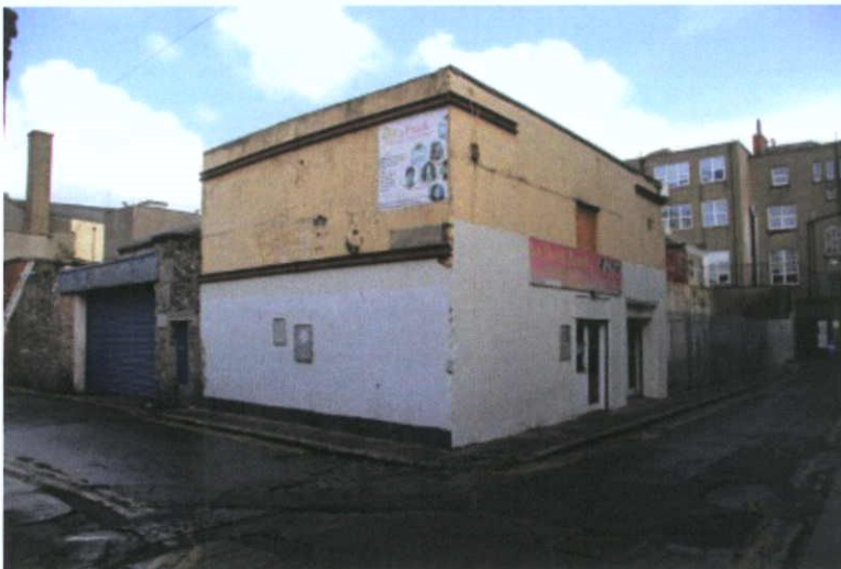
Plate 15.3.13 The corner sited No.60A O'Connell Street Upper, at the junction of Moore Lane and Henry Place.
