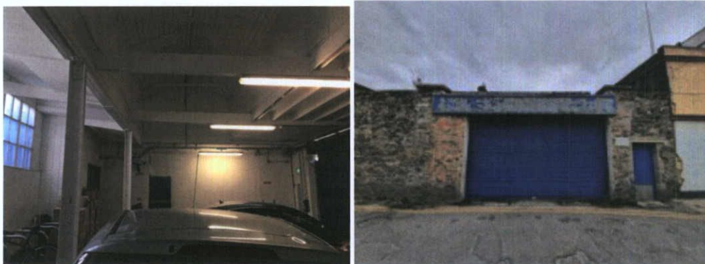
Plate 15.3.11 Interior and exterior of the car port
