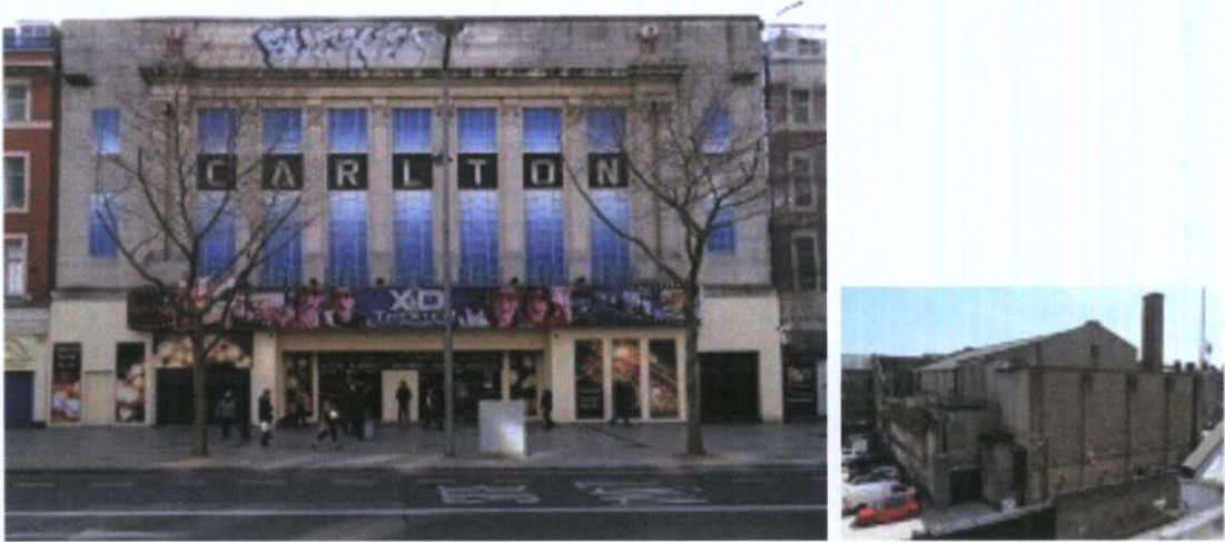
Plate 15.3.6 Front elevation of No.52-54 O'Connell Street Upper, the former Carlton Cinema and rear (upper) elevation on Moore Lane
