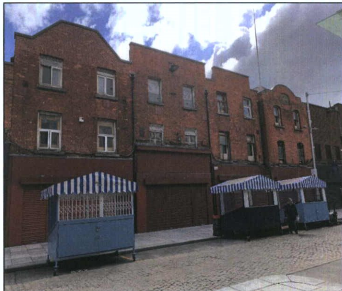
Figure 16.31: 14–17 Moore Street terrace, view southeast.
