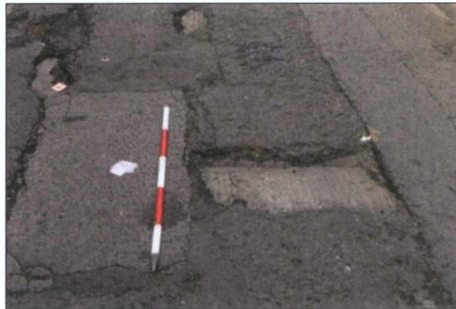
Figure 16.22: Concrete beneath tarmac surface on the Henry Place laneway
