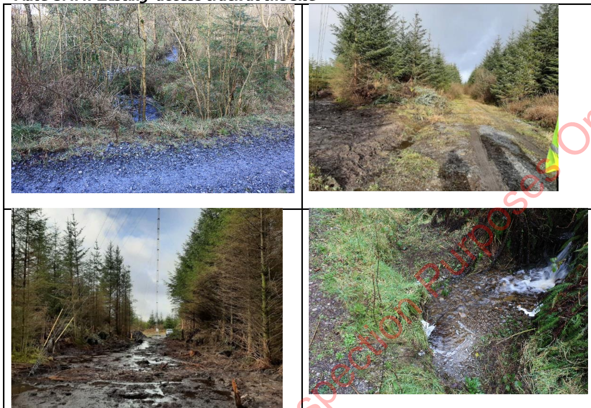
Plate 3.4.4: Existing access track at the Site
