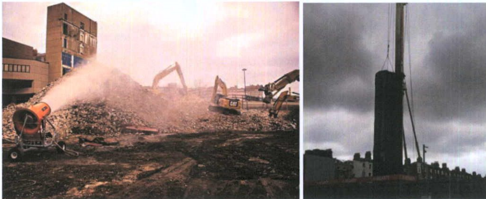
Figure 16 – Typical Dust Mitigation Measures
