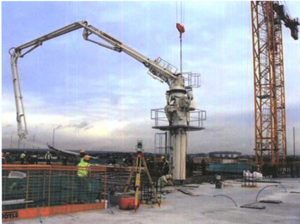
Figure 21 - Typical Concrete Placement
