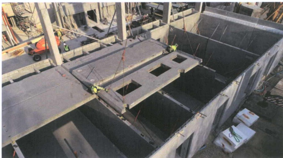
Figure 24. Typical Precast Concrete Construction
