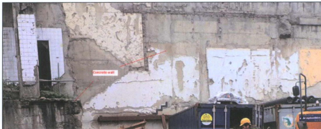
Figure 63 The north wall
