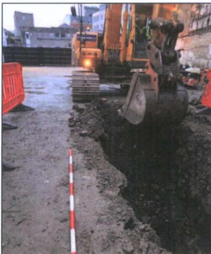
Figure 45 Trench 1, from the east
