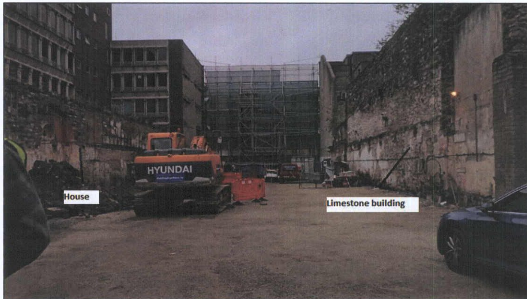
Figure 68 Site from the west
