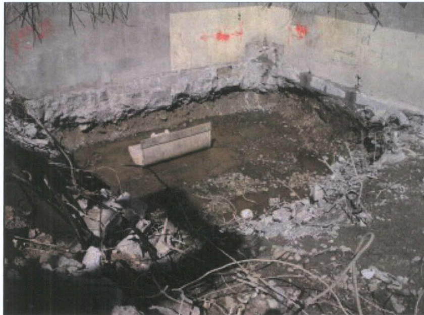
Figure 27 Trench 4, temporary crane base
