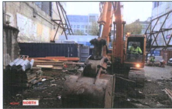
Trench 3, from the south Trench 4, from the west
