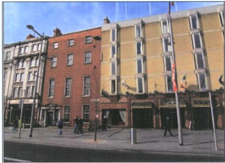
Figure 20 The Royal Dublin Hotel from the north pre demolition
