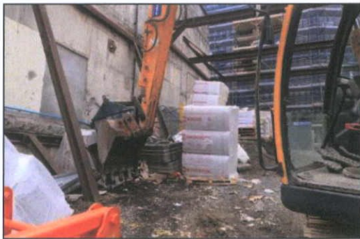
Figure 43 Trench 5, from the east
