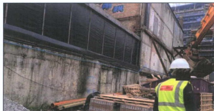
Figure 66 The south wall, west end
