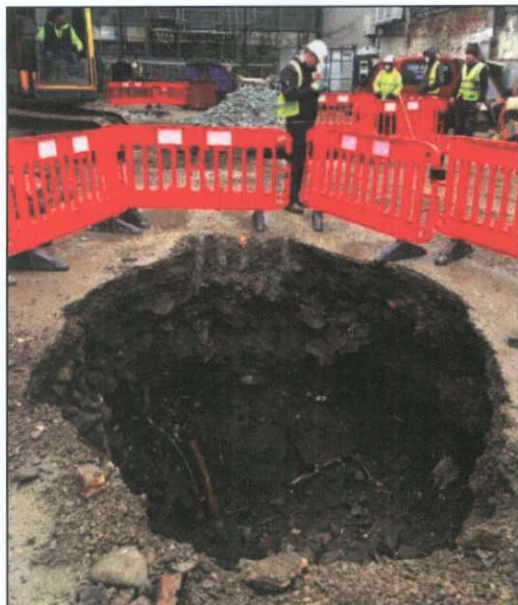
Figure 53 The expanding trench
