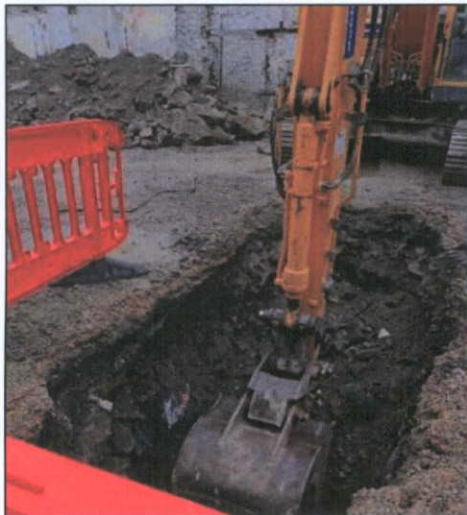
Figure 51 Trench 2 from the south
