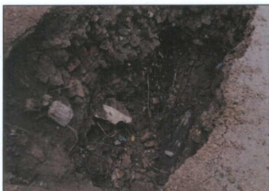
Figure 57 The floor abutting the wall foundation
