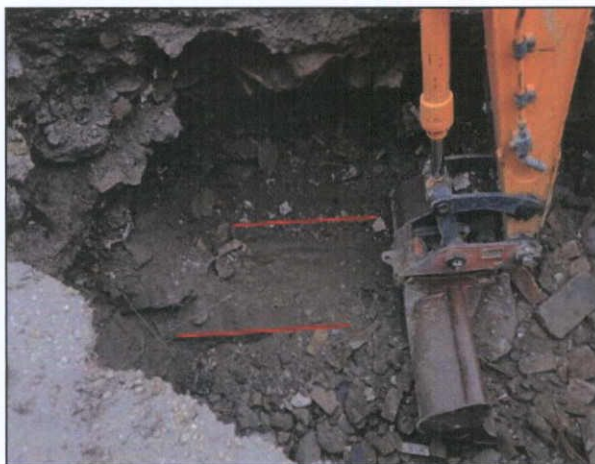
Figure 60 The structure from the north
