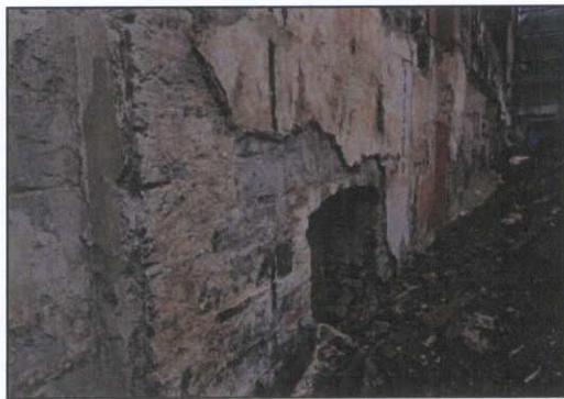
Figure 76 Projecting chimney breast
