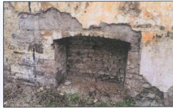
Figure 77 The fireplace in Room 2: type 3 brick
