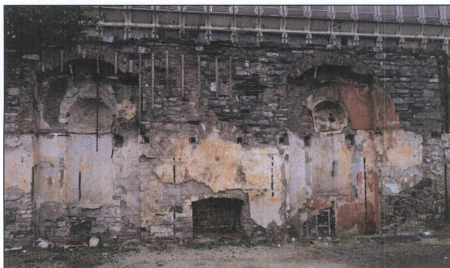
Figure 74 Building 2, from the south
