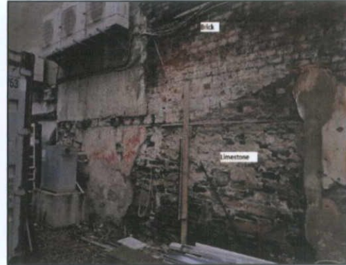
Figure 92 Section of the boundary wall
