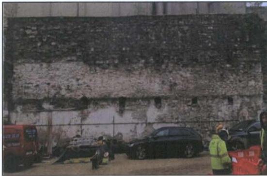
Figure 93 Building 4, from the north
