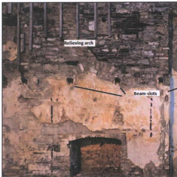
Figure 78 The relieving arch and beam-slots
