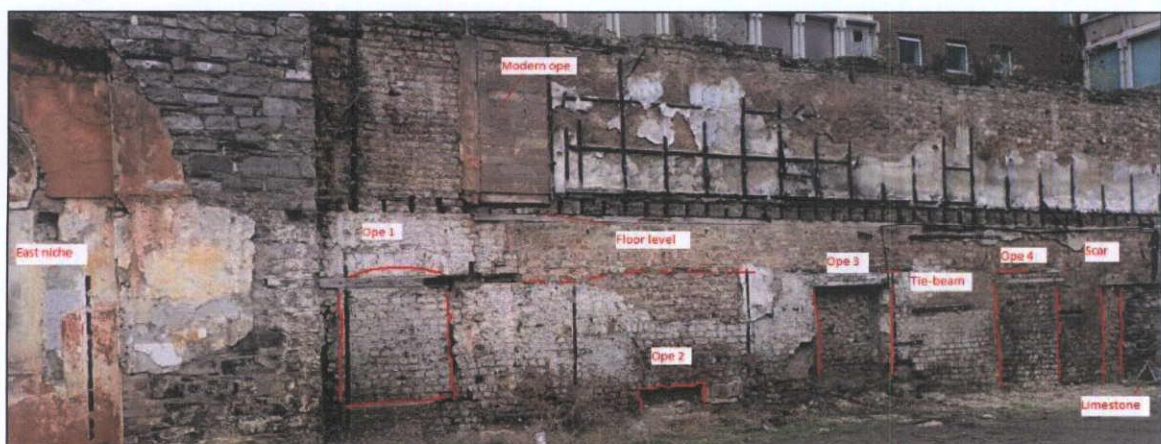
Figure 83 Building 3, from the west
