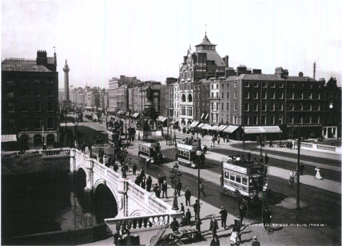
Figure 12.6: View of Sackville Street from the O'Connell Bridge c1910. The huge form of the Dublin Bread Company dominates the street.
