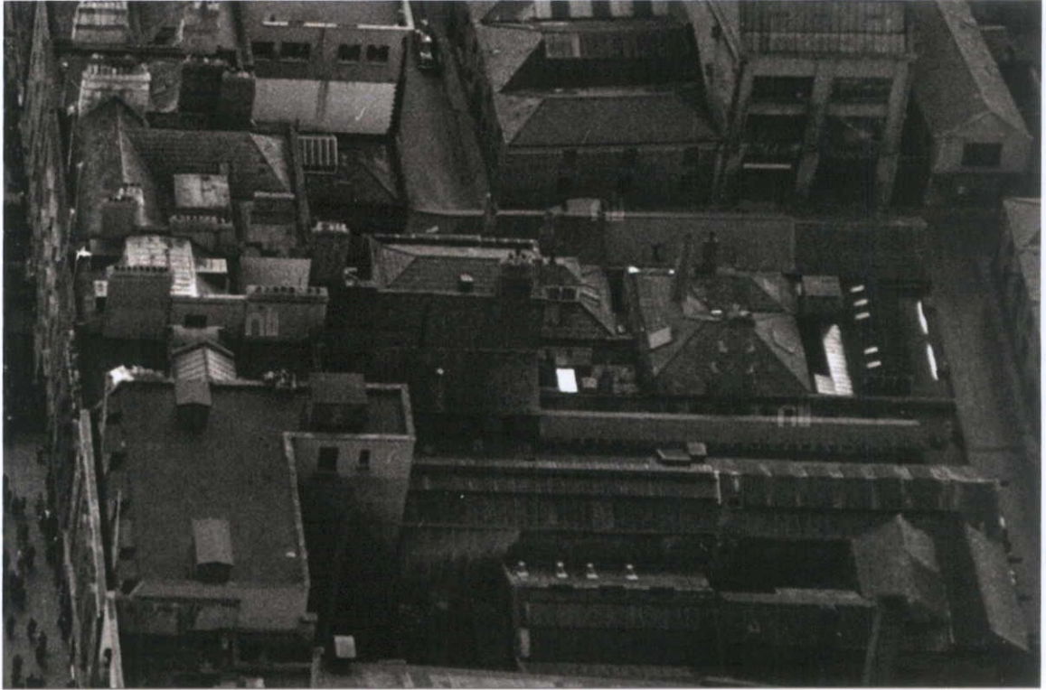
Figure 15.3.8: An aerial photograph of Site 2AB (in part), 1955 provides an interesting overview of the complex at the rear of No.59. The roof of reading room and the 'regency annex' is visible, with a lantern-roofed structure (since demolished) in the interstitial space. Source 'The Morgan Collection', National Library of Ireland.
