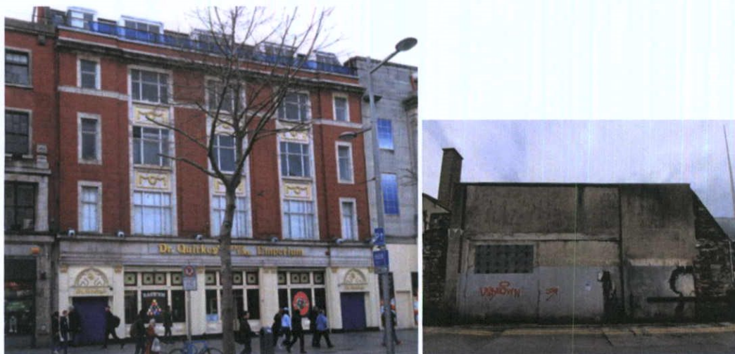
Plate 15.3.7 Front façade of No.55-56 O'Connell Street Upper and its mixed material rear elevation on Moore Lane
