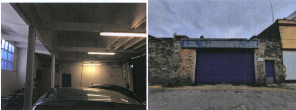
Plate 15.3.11 Interior and exterior of the car port
