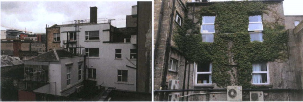
Plate 15.3.12 Left: Recency annex attached to the rear return of No.59 and right: western elevation of annex
