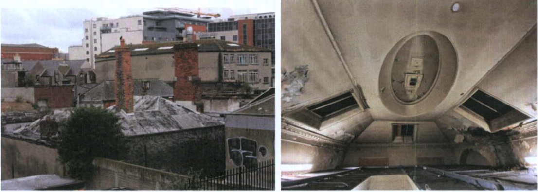
Plate 15.3.10 Roof and interior of rear of a former reading room pertaining to the Sackville Street Club
