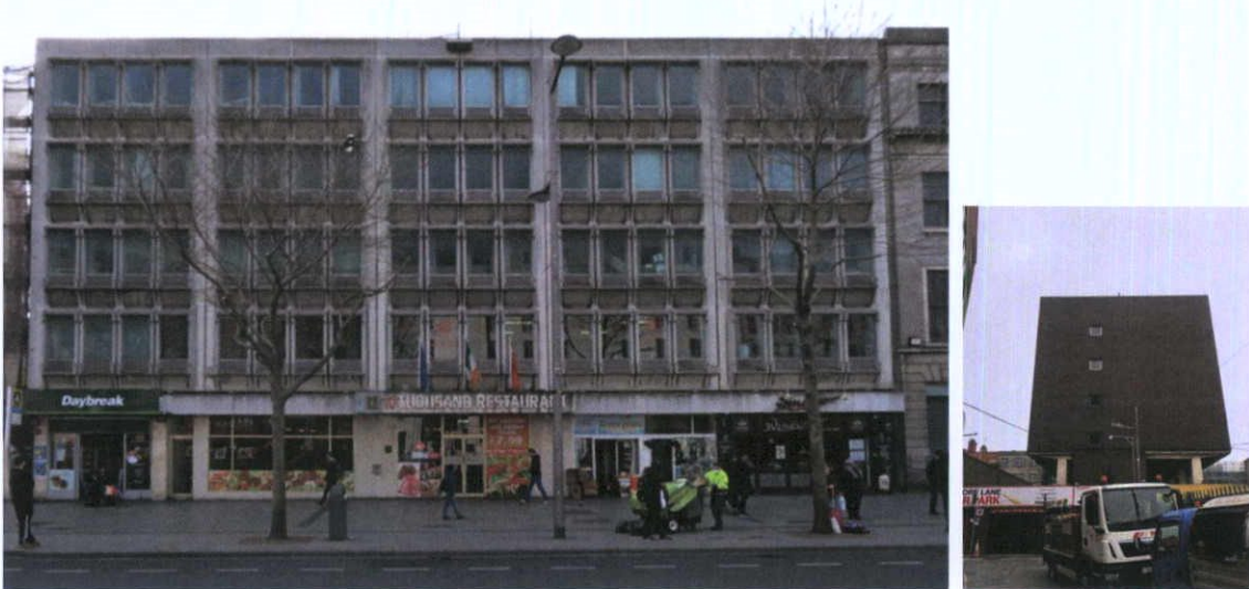
Plate 15.3.4 Front of No.46-49 O'Connell Street Upper and rear elevation on Moore Lane
