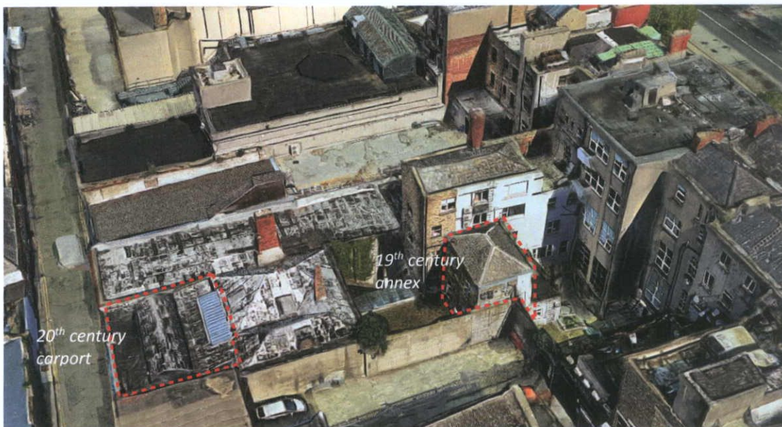
Plate 15.5.1 Identification of structures proposed for removal at the rear of No.59 O'Connell Street Upper; the 20 th century carport to the west and the 19 th century annex to the east.
