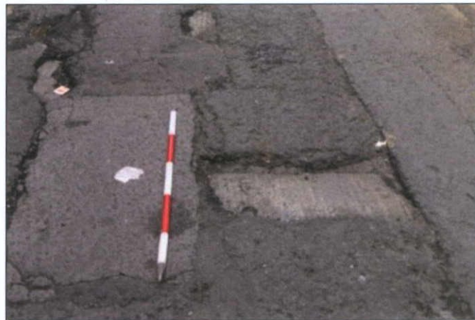
Figure 16.22: Concrete beneath tarmacadam surface on the Henry Place laneway
