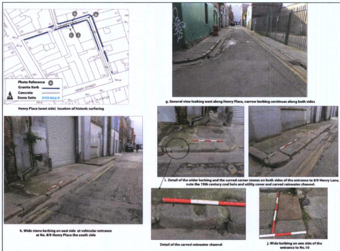
Figure 16.24: Henry Place (east-west running section) historic paving
