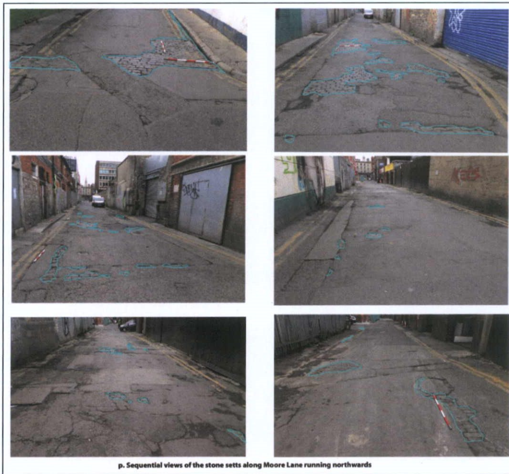
Figure 16.26: Moore Lane stone sett pavements beneath the tarmac surface
