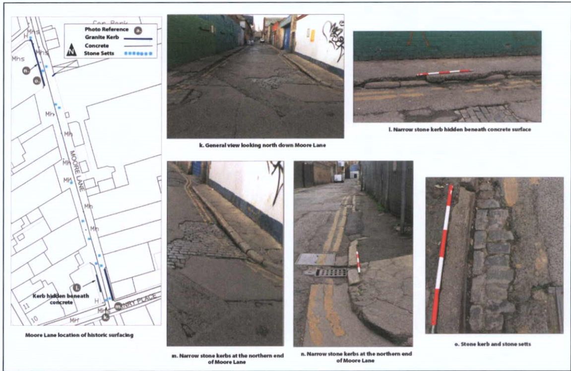
Figure 16.25: Moore Lane granite kerbing
