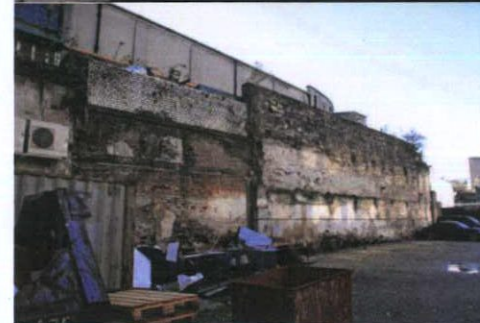
Indentations to southern boundary wall at No.51 suggesting a large-scale industrial type structure
