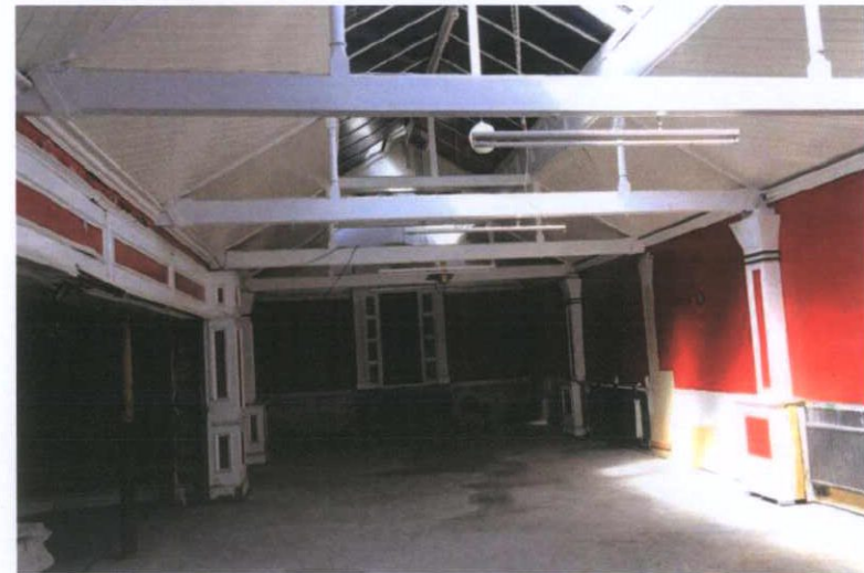
Link building between O'Connell Hall and main house
