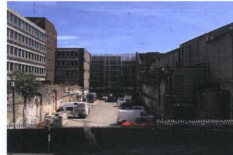
High level view of vacant site. Note niches and indentations in boundary walls. Front wall onto O'Connell Street and rear wall onto Moore Lane have been removed.
