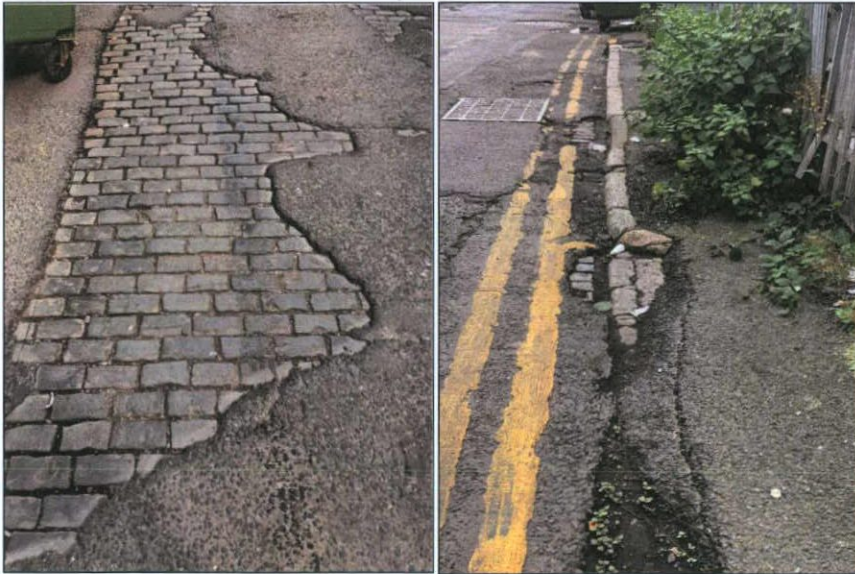
Plate 5 Relic street kerbs and paving
