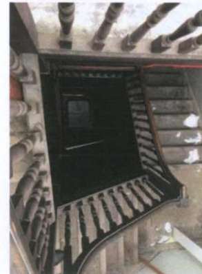
Staircase from 3rd floor level
