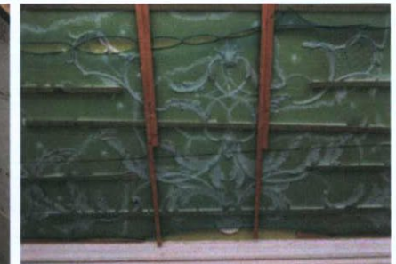
Sample of decorative plasterwork
