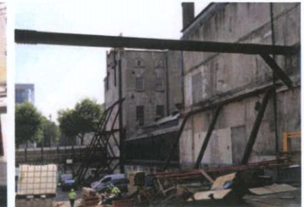
Interior of vacant site
