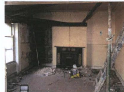
Upper floor, note structural propping
