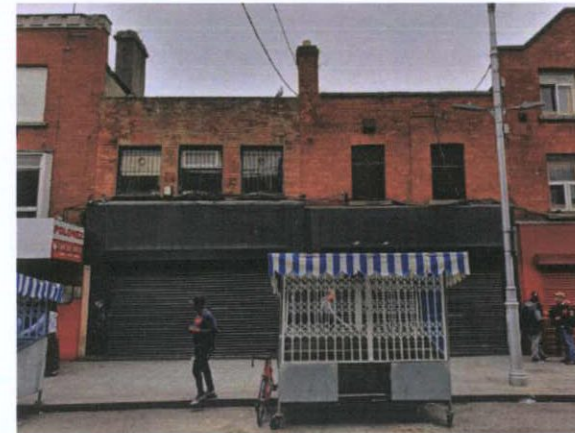
Front façade 19 Moore Street, left-hand-side
