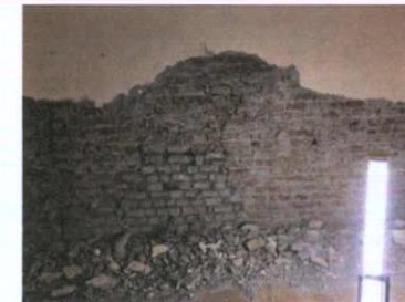
Creep hole at first floor level
