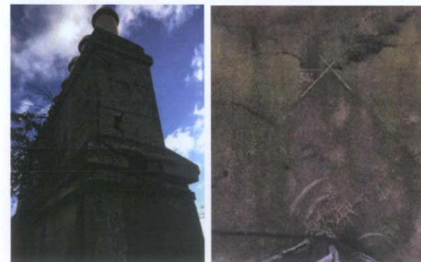
Early chimney with 18 th century brick found to front north-eastern stack
