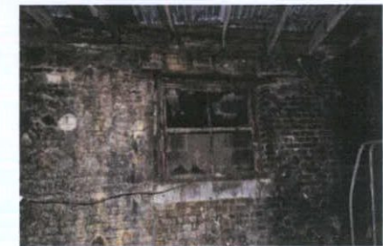
Sash window within modified structure
