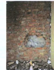
Creep hole at entrance level
