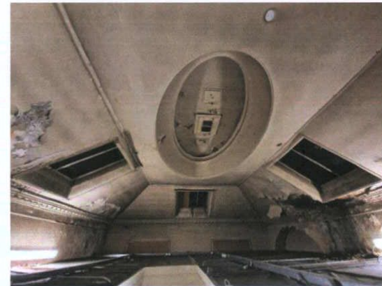
Ceiling of former reading room above contemporary partition walls
