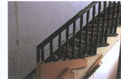
Detail of stair
