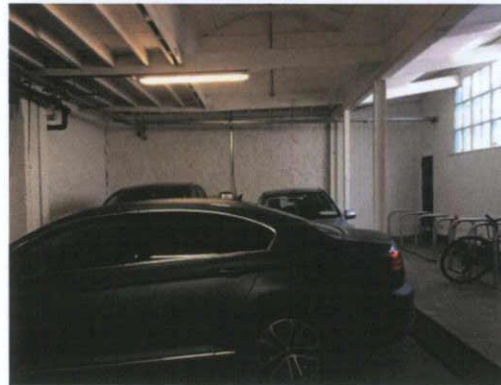
Interior of Car Port due north and south
