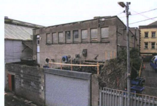
Rear elevation onto Moore Lane
