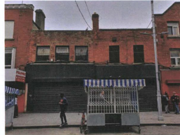
Front façade 18 Moore Street, right-hand-side
