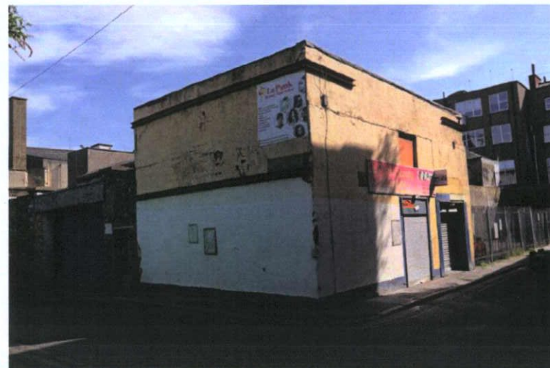
Exterior of 60a O'Connell Street at the junction of Henry Place and Moore Lane
