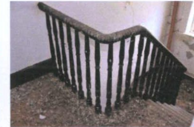
Turned balusters and timber handrail
