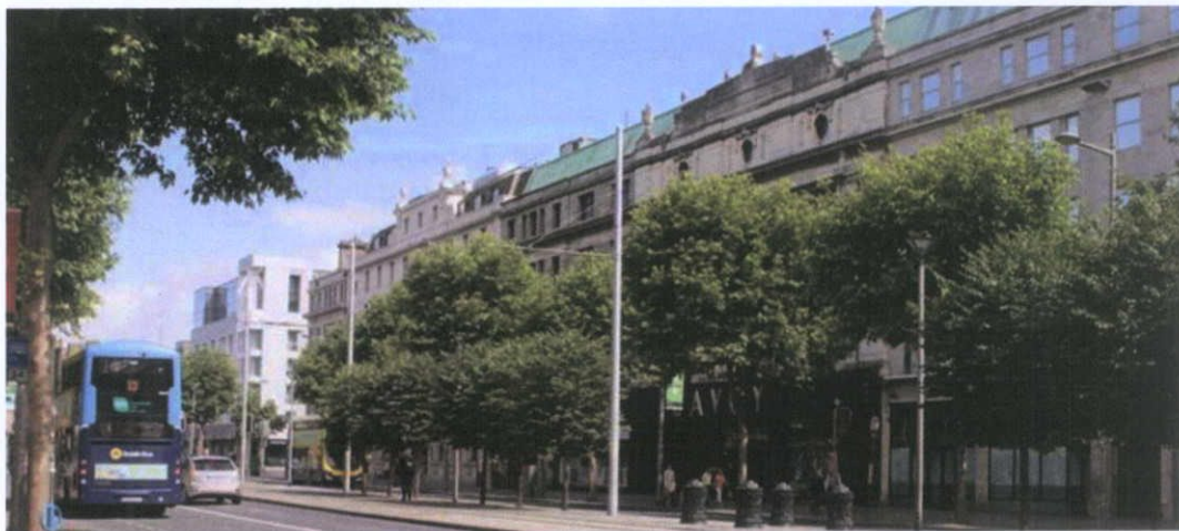
Figure 4.29 Views across of O'Connell Street Upper; Above: The Luas divides the street and planting obscures much of the architecture of the street including on the west side, No.42 - the only near-complete, original house on Sackville Mall. Below: Trees obscuring the Gresham Hotel on the east side.
