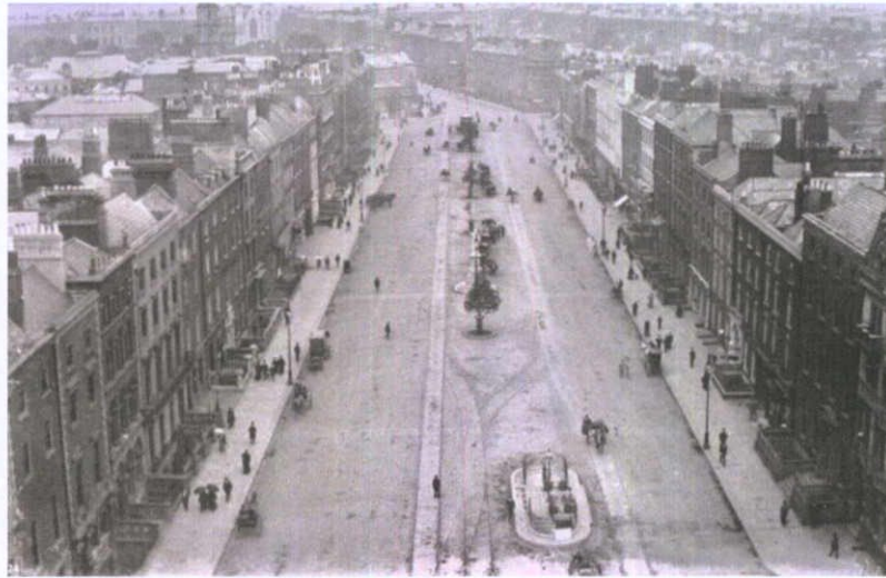
Figure 3.12 O'Connell Street Upper in the late-nineteenth century; the majority of the areas are still extant. (IAA)
