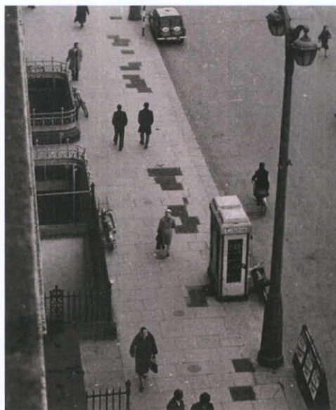
Figure 3.13 A number of so-called coal-stoppers are visible along the pavement, giving access to the vaults under the pavement, (1962). (Courtesy of Dublin City Library and Archive)
