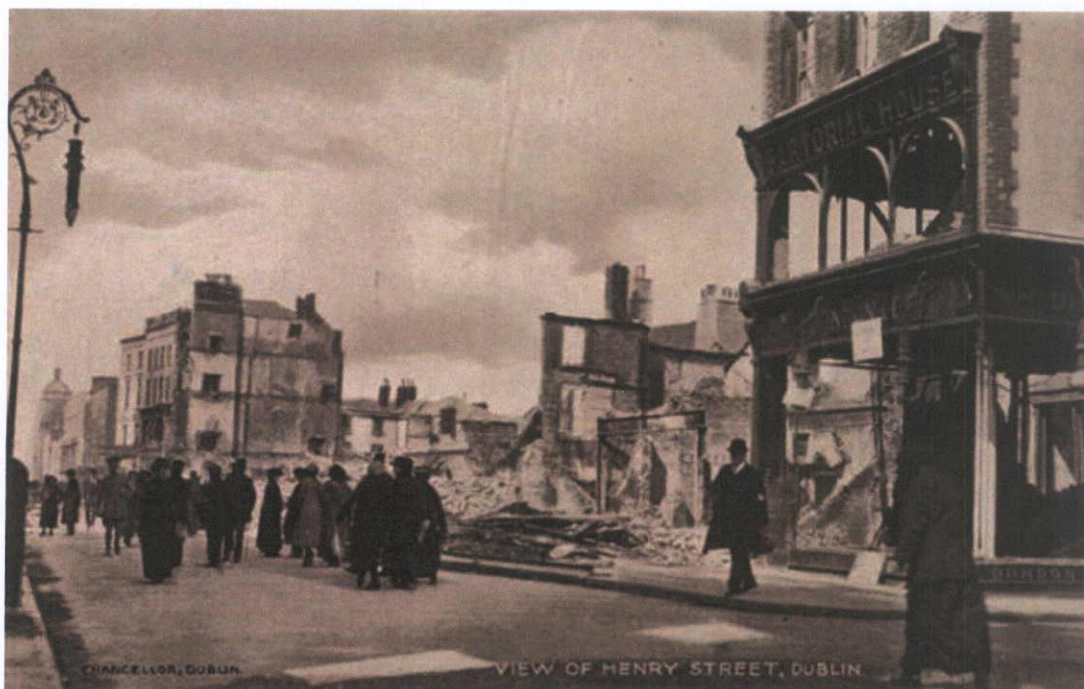
Figure 7.6 Henry Street looking west, aftermath of the Easter Rising. Note the shell of the building on the right. This plot had been rebuilt to create the new typology with large first floor display windows before 1916. (Courtesy of Dublin City Library and Archive)
