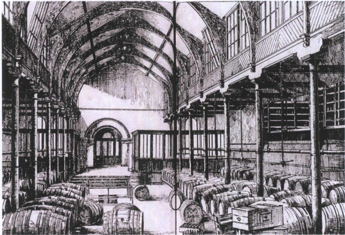
Figure 4.14 Gilbey's warehouse (Dublin Builder 1864).
