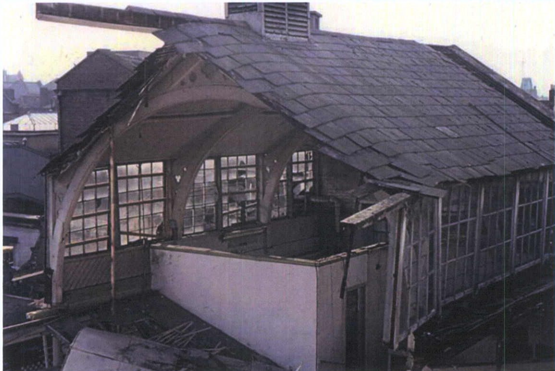
Figure 4.15 Gilbey's Warehouse during demolition 1972. (Courtesy of Dublin City Library and Archive)
