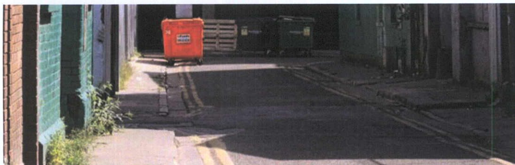
Figure 9.17 Henry Place some surviving sections of pavement. A section on the right has larger width granite kerbstones. 2020
