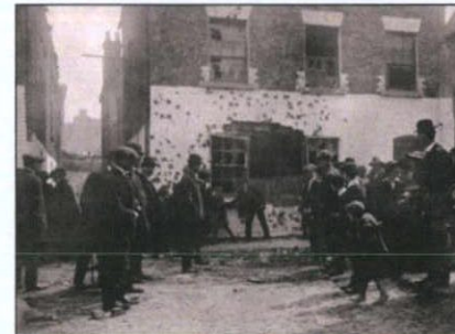
P 24 Unknown Building 1916, thought to be on the site of 10 Henry Place, depicting significant damage from fire on the front.
