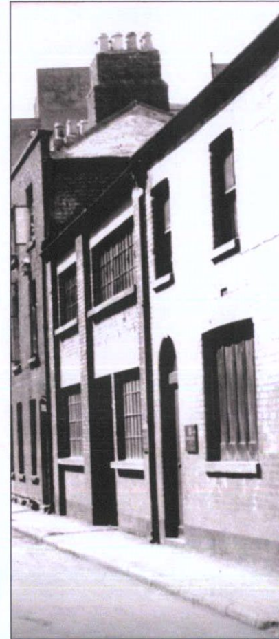
P 21 Eastern façade of 6-8 Henry Place, 1952, depicting lower floor and arched headed doorway which survives, though blocked up. Source: Military Archives.
