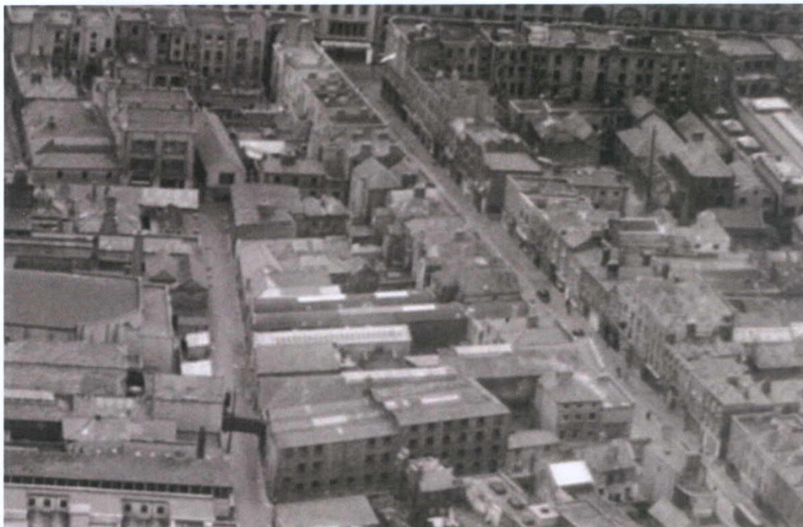
Figure 8.11 Looking south over Moore Street on the right and Moore Lane to the left, 1949. (Britain from Above ref. XAW027121)
