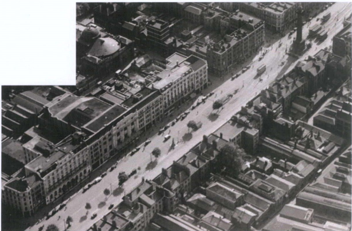
Figure 9.11 1933: The trees are on O'Connell Street Upper only. There appears to have been some recent replacements. Note also the sole, overgrown surviving tree in a garden on the west side. (Britain from Above, photograph ref XPW043448).
