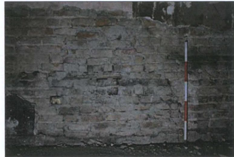
P 14 Infilled opening recorded in 10 Moore Street, Extract: Myles Report.
