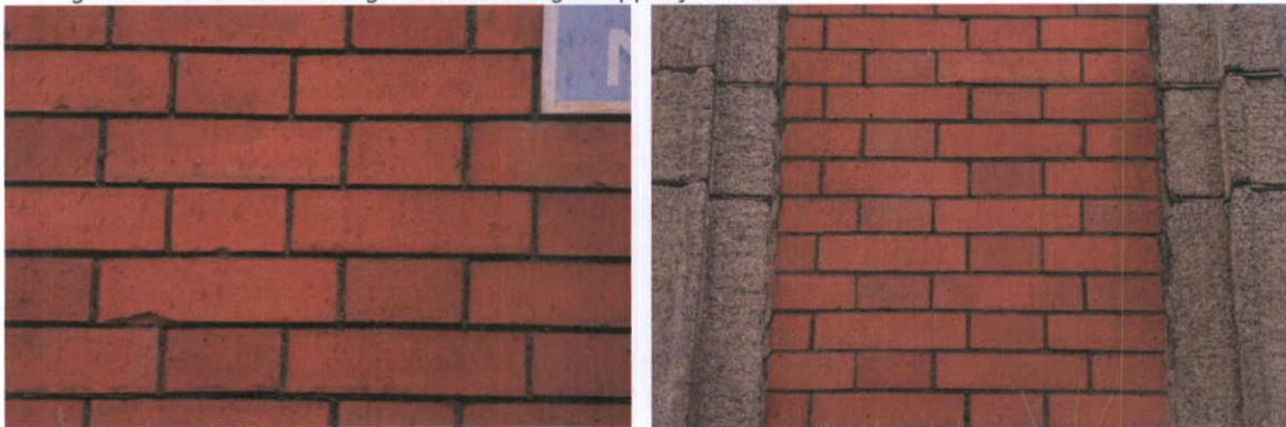
Fig.4.5.3: Detail of the c.1917-1920 brickwork at 41 Henry Street.
