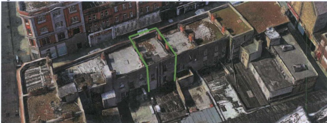
Fig.4.8.3: GoogleMaps view of the roof and rear elevation of No.4 Moore Street.
