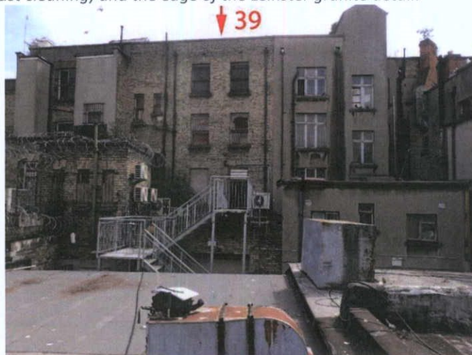
Fig.4.3.4: No.39 Henry Street forms part of a terrace using identical yellow stock brick, and all buildings appear to have been built at the same time.
