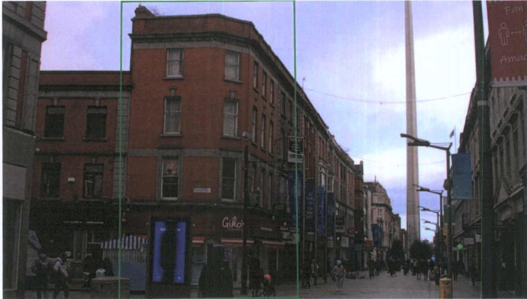
Fig.4.5.1: The brickwork on the soiled façade of No.40 Henry Street consists of well-fired machine-cut red clay brick with weatherstruck Portland Cement-based pointing mortars. Leinster granite was used for architectural detailing. The work probably dates to c.1917-1920.
