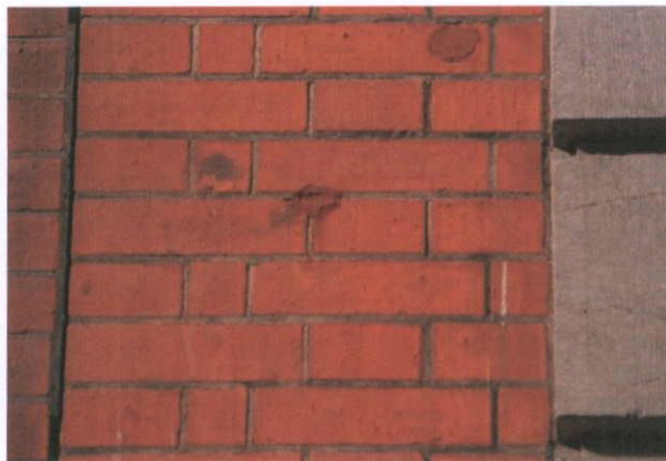
Fig.4.2.2: The brickwork and limestone detailing on the façade of 38 Henry Street has been cleaned and small 'plastic' mortar repairs (appearing dark red) seen.
