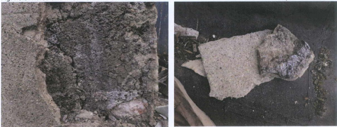
Fig.4.8.6: Concrete fabric beneath the Portland Cement render coat.
