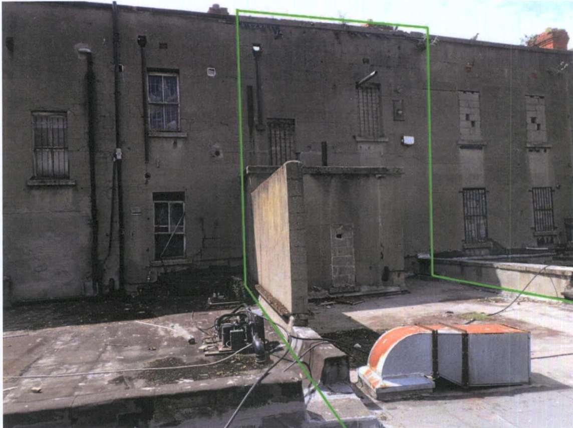
Fig.4.9.4: The rear elevation of No.5 Moore Street, built c.1917. Note that the colour and composition of the Portland Cement render and the configuration of the openings of Nos.5 and 4 matches; while the neighbouring No.6 Moore Street (right of image) was built using a slightly different Portland Cement render mix and with a different window arrangement.
