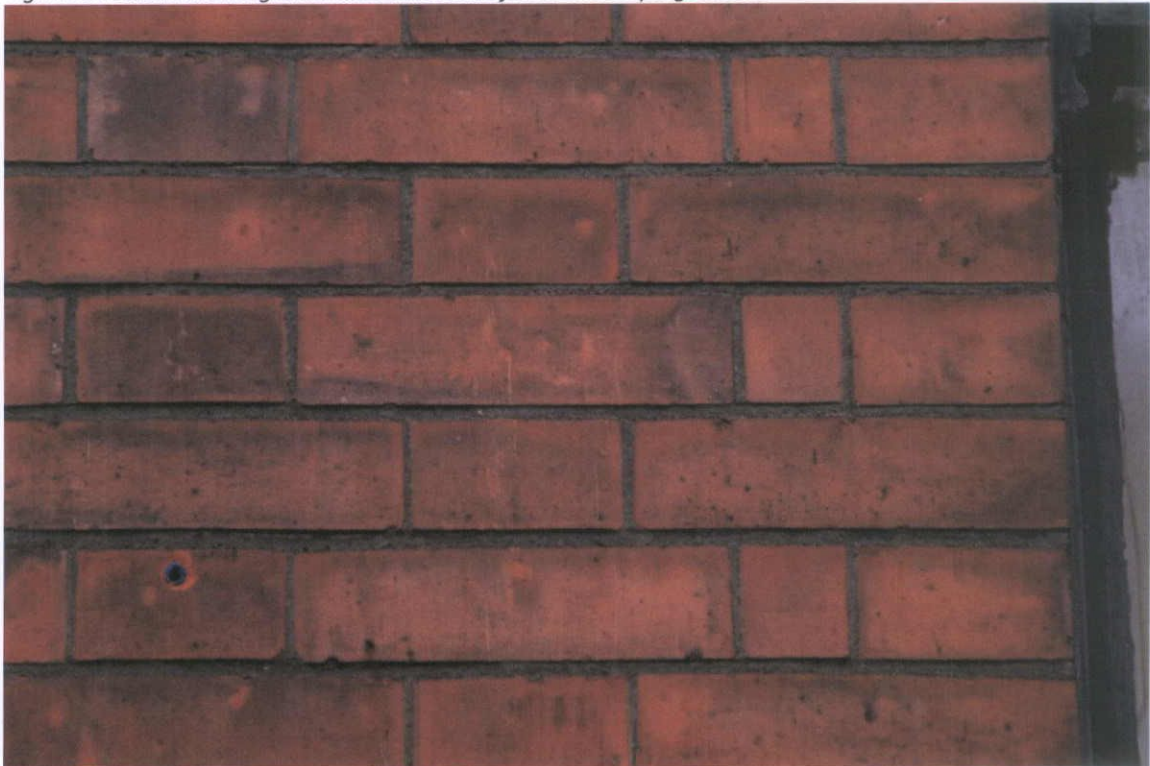
Fig.4.7.4: The soiled brickwork is machine-cut kiln-fired, consistent with c.1917 work.
