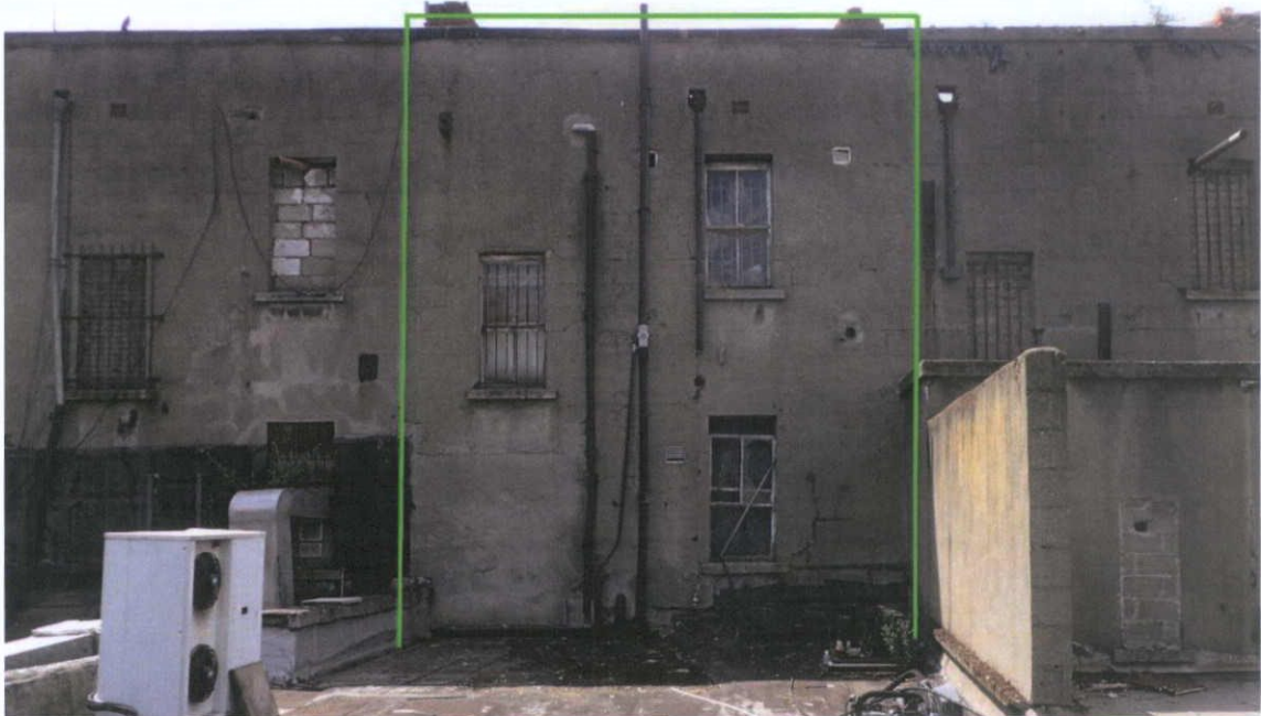
Fig.4.8.4: Note the rendered rear of No.4 mirrors the treatment of No.3 and 5.
