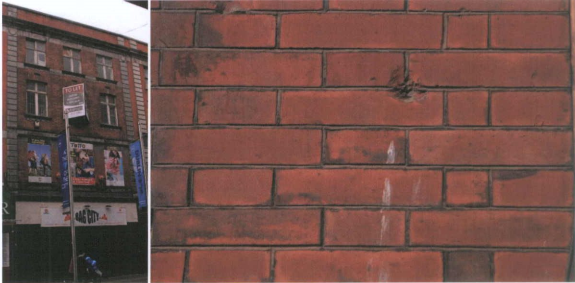
Fig.4.4.1: The brickwork on the soiled façade of No.40 Henry Street consists of well-fired machine-cut red clay brick with weatherstruck Portland Cement-based pointing mortars. Leinster granite was used for architectural detailing. The work probably dates to c.1917-1920.
