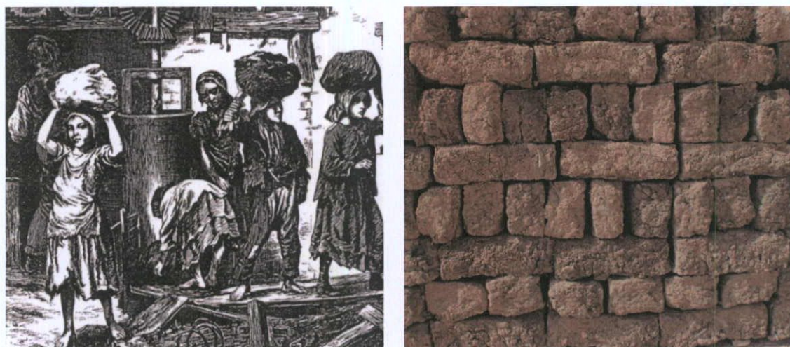
Fig.3.4: 'The Brick Children' from 'The Graphic', Saturday 27 May 1871, with a pug mill in the background; and a detail showing hand-made bricks which had been laid out to dry and then stacked.
