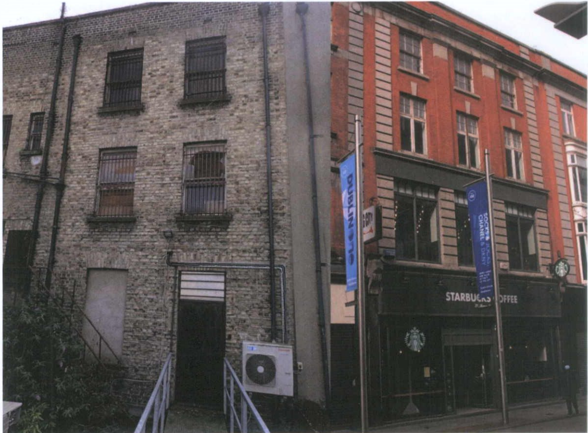
Fig.4.3.1: General views of the rear elevation (note rebuilt parapet) and façade of 39 Henry Street. The rear elevation brickwork matches that of No.38 and is contemporary with same.
