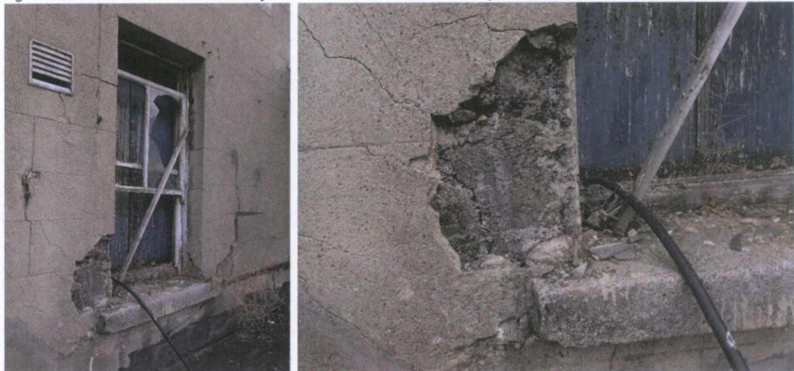
Fig.4.8.5: Ruled and lined Portland Cement render over a concrete structure. Rear elevation, No.4 Moore St.
