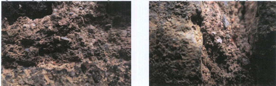
Fig.4.2.6: Crushed brick in the bedding mortars at the rear of No.38 Henry Street.
