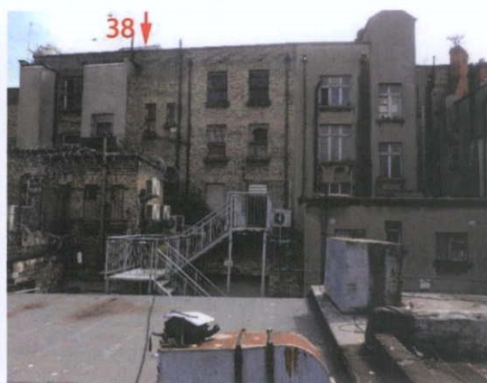
Fig.4.2.3: No.38 Henry Street forming part of a terrace using identical c.1920 yellow stock brick.
