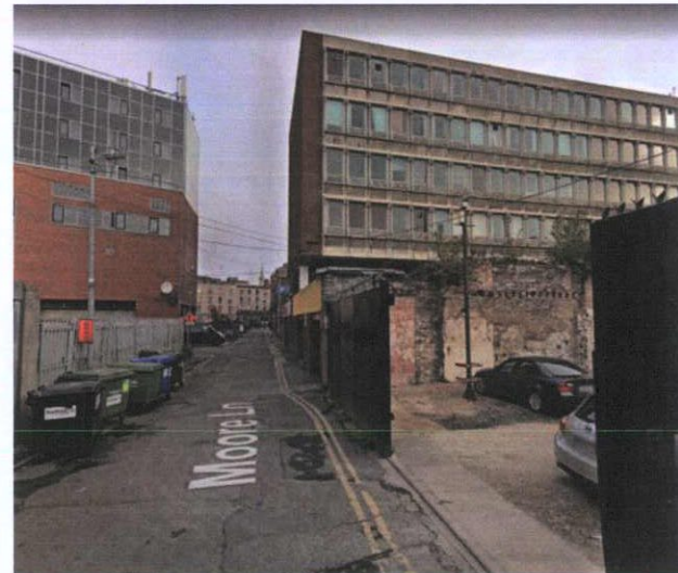
P 44 Moore Lane, midway point, facing north towards Parnell Street, 2020, Source: Google
