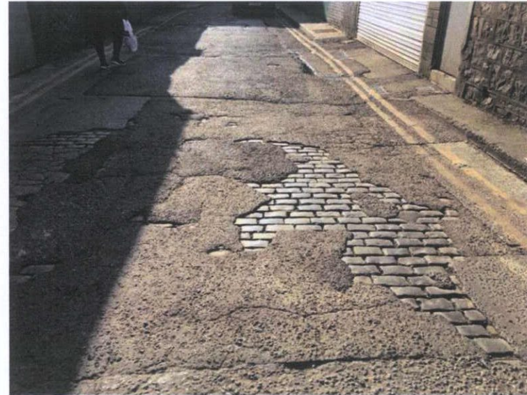
P 39 Original setts on Moore Lane visible under modern road surface.
