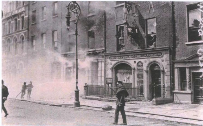
P 51 43 and 44 Sackville Street following the fire.
