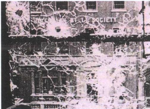
P 55 Shattered window at the Sackville Club, 59 O'Connell Street Upper (Source: George Morrison)
