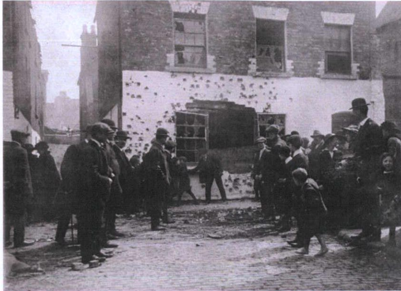
P 35 'Unknown building' damaged in 1916, thought be 10 Henry Place, at the junction of Moore Lane and Henry Place. Property Loss Archives describes the front of 10 Henry Place blown in by shell fire.
