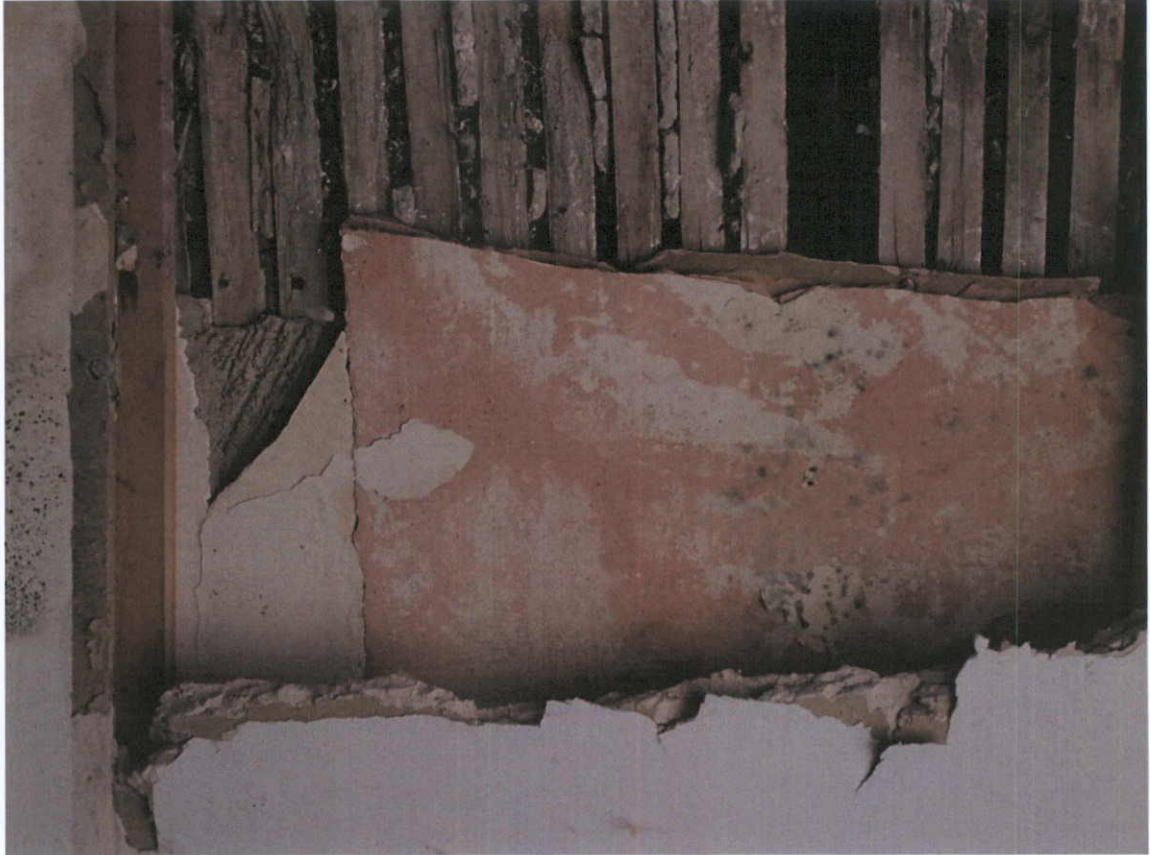
Fig.4.12.6: Lime lath-and-plaster ceiling surviving at the first floor of Nos.8-9 Moore Street (concealed behind poorly-applied later ceiling plaster layers).
