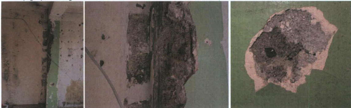
Fig.5.8.4: The party wall (left) and inner face of the west wall (right) are of concrete.
