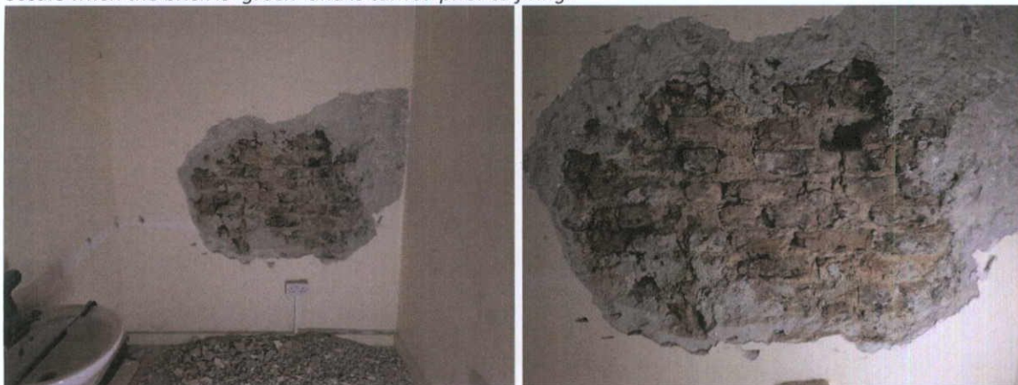
Fig.5.3.5: Internal party wall at upper floor level showing hand-made brick bedded in a lime bedding mortar.
