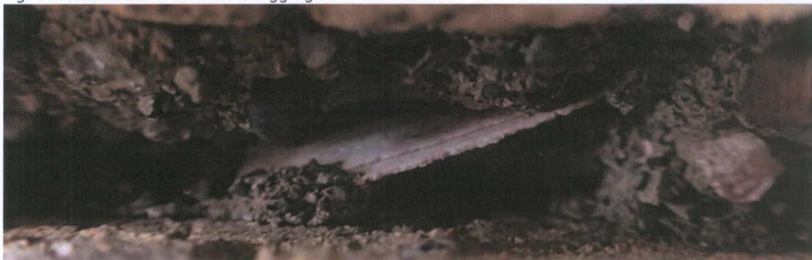
Fig. 4.17.6: Shell used as porous calcareous aggregate in the mortar.
