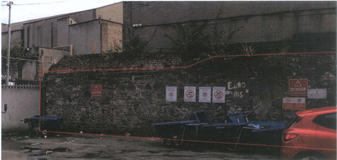
Fig.6.4.5: The eastern section of the wall consists of hewn Calp limestone masonry bonded in a lime-based mortar.
