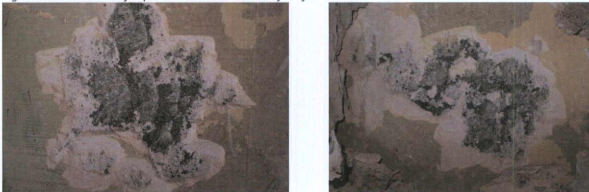
Fig. 4.17.13: Cement used to plaster the inside of the north wall at first floor level.
