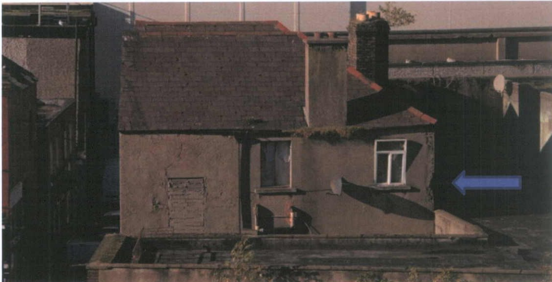
Fig.5.1.5: The rear of No.10 Moore Street is rendered. The north side (arrowed) was opened up.
