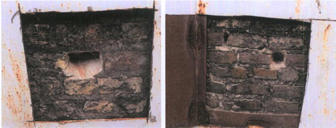
Fig.4.16.3: Nineteenth century yellow stock brick, first floor level, west elevation.
