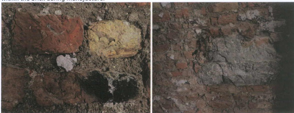
Fig.5.3.9: Late eighteenth/early nineteenth century brickwork, ground floor, south wall, with concrete infill.
