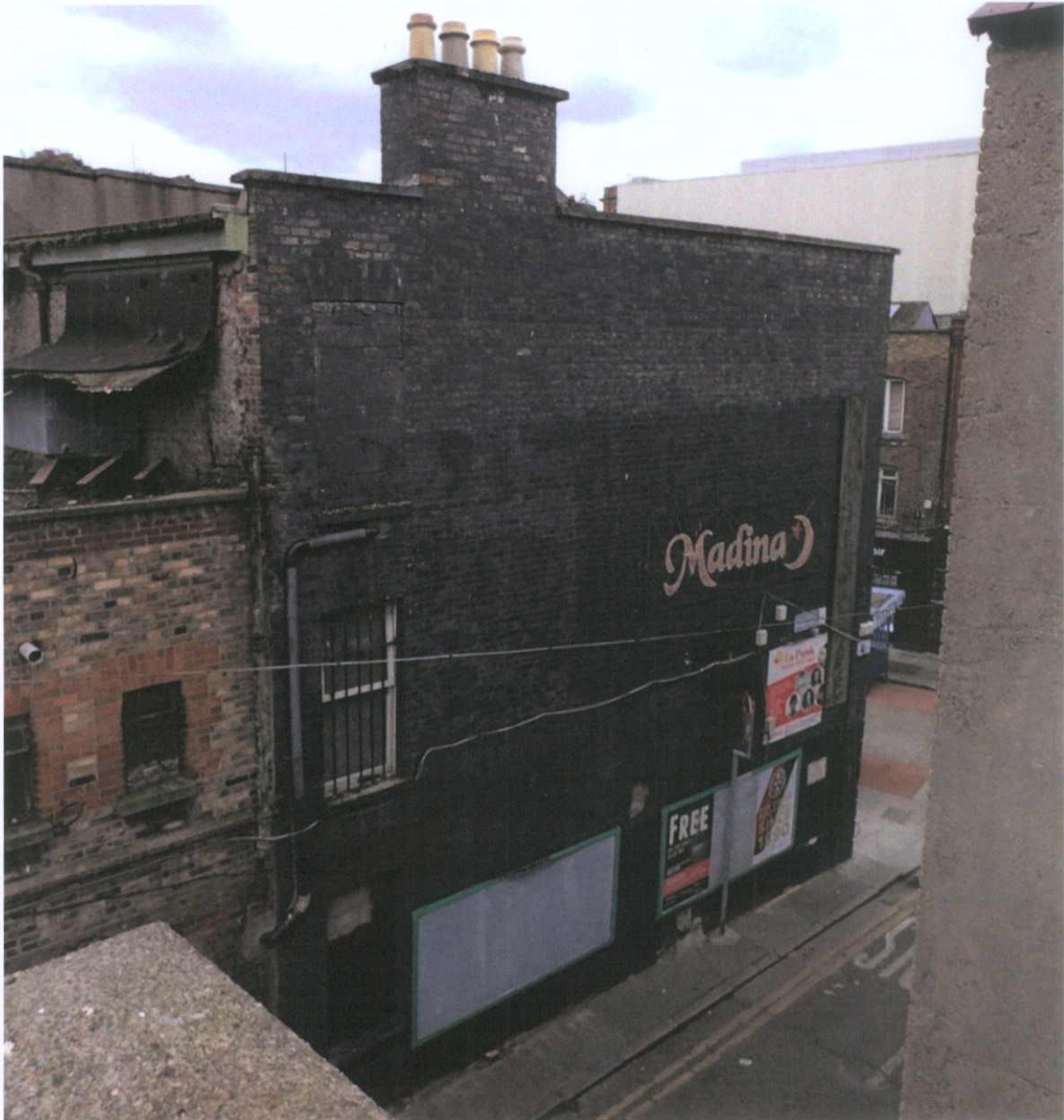
Fig.4.12.4: View of the painted north wall of No.9 Moore Street.
