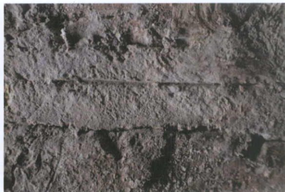
Fig.5.1.12: Lined mortar joint on the brick party wall between No.10 and 11 Moore Street, with traces of the animal hairs from the haired lime plaster adhering to the joint (right). This finish is also found on the eighteenth century internal walls of No.42 O'Connell Street.
