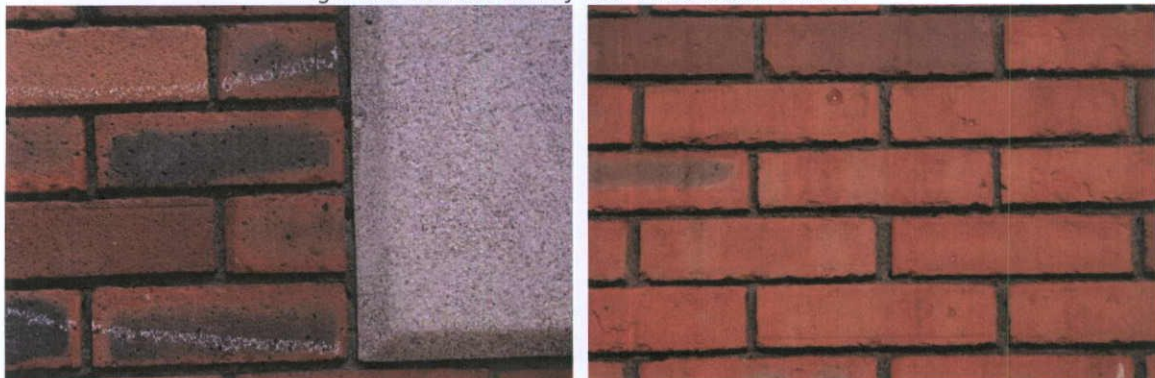
Fig.8.3.2: Detail of the brickwork and cast stone quoins.
