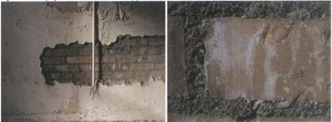
Fig.6.1.8: The north wall (party wall with No.22) consists of kiln-fired extruded machine-cut yellow stock brick. Similar brick is found in the link building between 42 O'Connell Street and O'Connell Hall.
