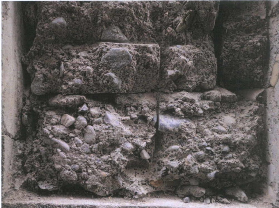
Fig.4.16.14: 1959 concrete repair, east elevation, ground floor level.
