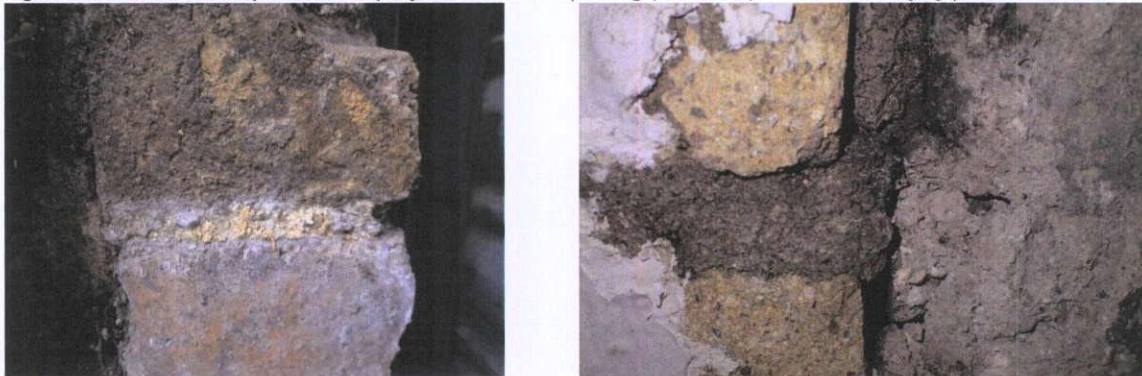
Fig.5.6.8: Detail of yellow stock brick from the inner face of the south wall bedded in a lime-rich mortar; and the inner face of the east wall showing coarse yellow brick bedded in a cement mortar (right).
