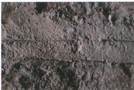
Fig.5.1.12: Lined mortar joint on the brick party wall between No.10 and 11 Moore Street, with traces of the animal hairs from the haired lime plaster adhering to the joint (right). This finish is also found on the eighteenth century internal walls of No.42 O'Connell Street.
