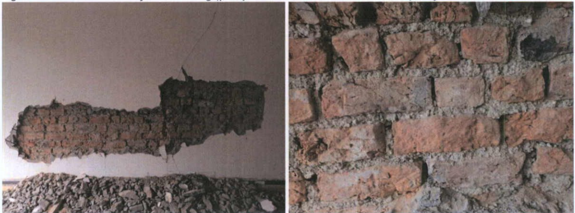
Fig.6.1.4: The party wall between Nos.20 and 21 is of hand-made clamp-fired brick laid in deep lime mortar joints.
