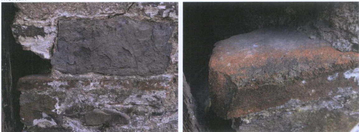
Fig.6.4.6: Ceramic tile used within the masonry.
