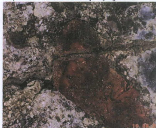
Fig. 4.17.9: Crushed brick in the mortar.
