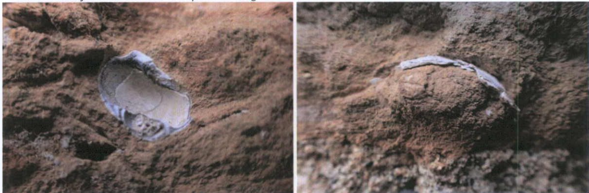
Fig.5.1.8: Detail of brick from the north elevation of No.10 Moore Street showing examples of shell inclusions in the fired clay matrix.
