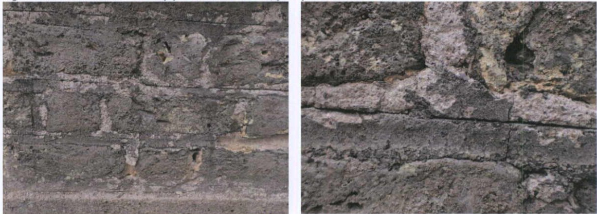
Fig.4.16.4: 'Pennystruck' lime pointing mortars, first floor level, south elevation.
