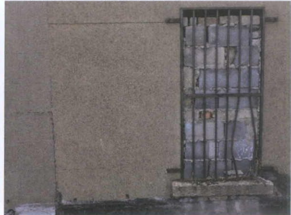
Fig.4.10.3: The rear elevation has a Portland Cement render which has weathered differently to its neighbor, indicating that the cement binders are slightly different in composition.
