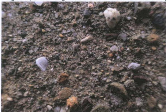
Fig.4.10.3: Detail of the aggregate standing proud of the surface of the render at the rear of No.6 Moore Street consisting of rounded natural aggregate and shell.
