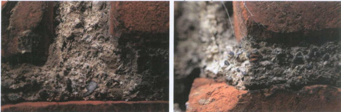
Fig.5.5.5: The lime-based bedding mortar contains sub-rounded to sub-angular aggregate, fine lime lumps and partially slaked limestone and some crushed brick.
