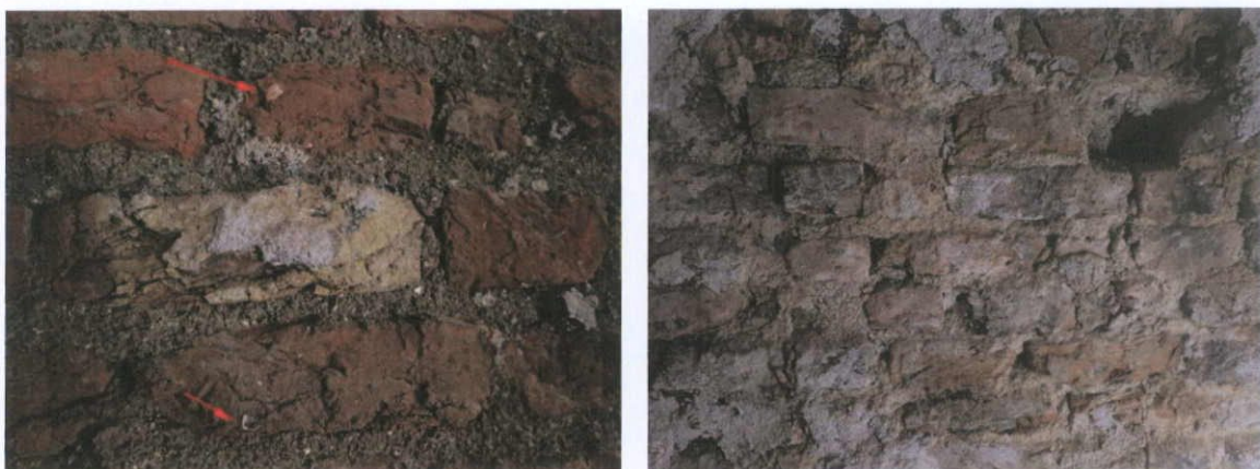
Fig.5.3.2: 13 Moore Street, Ground Floor, Rear Room, north face of south wall (party wall with No.12). Detail of handmade brickwork from the internal party wall between Nos.13 & 12 Moore Street with burnt shell inclusions (arrowed) within the fired clay matrix (left). The original brick at first floor level (right) is also hand-made and of varying dimensions and qualities, laid in deep lime mortar joints. These are ‘place’ bricks intended to be coated with a lime plaster.
