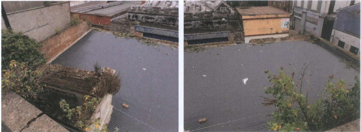
Fig.5.6.3: View of the roof from the west, with the inner leaf of yellow stock brick from the now lost first floor level visible at the wall tops.
