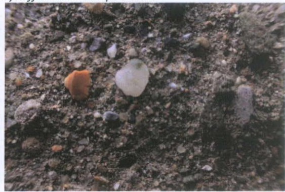
Fig.4.10.3: Detail of the aggregate standing proud of the surface of the render at the rear of No.6 Moore Street consisting of rounded natural aggregate and shell.
