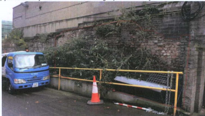
Fig.8.4.10: The western section of the wall is composed of red and yellow place brick, and appears to represent internal lining.
