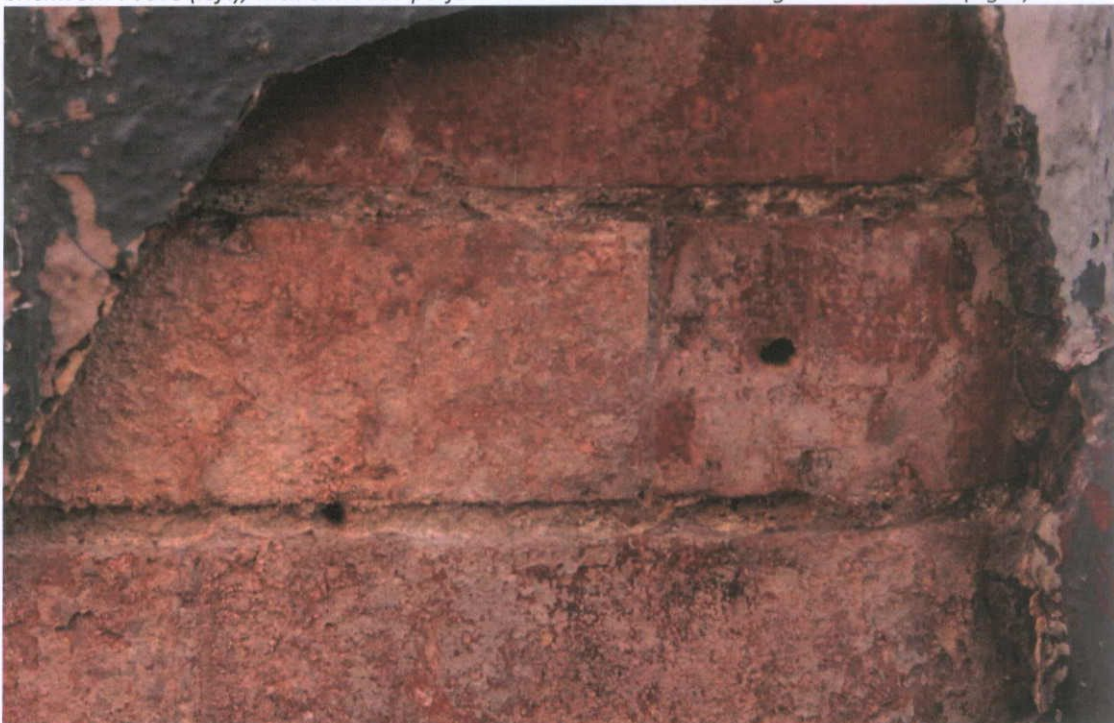
Fig.4.14.4: Detail of the curved brickwork at the north-east corner of the building.
