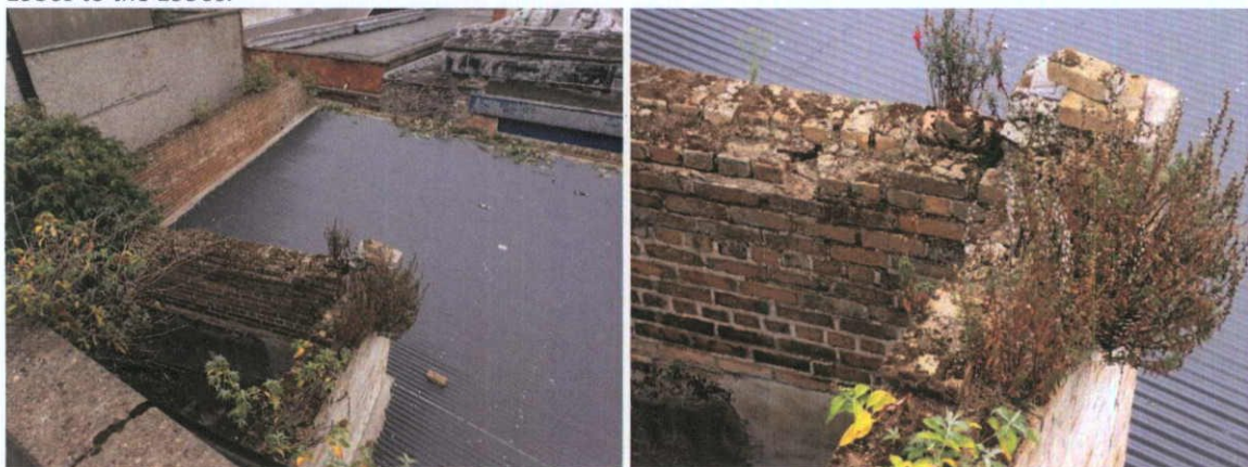
Fig.5.2.2: Yellow stock brick sampled from the rear return of No.12 Moore Street.
