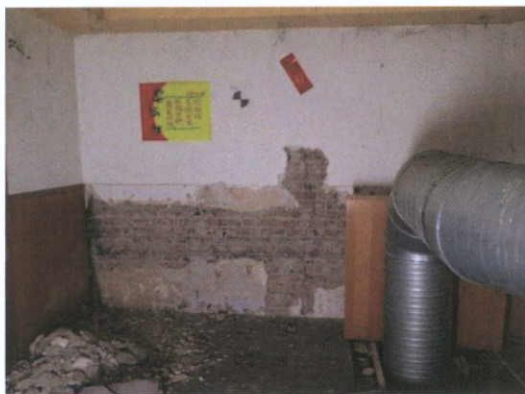
Fig.5.1.10: The party wall between Nos.10 and 11 Moore Street contains early brickwork with lime mortars struck in the same style as the internal walls of the mid-eighteenth century No.42 O'Connell Street.
