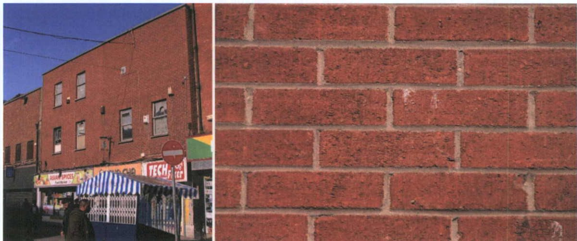
Fig.5.2.1: The façade of 11-12 Moore Street was built of machine-cut textured brick bedding in Portland Cement and finished with a 'bucket handle' joint, this finish is common from the late 1950s-1980s. The brick is widely used in the twentieth century, and this type of textured brick could date from anywhere from the 1930s to the 1990s.
