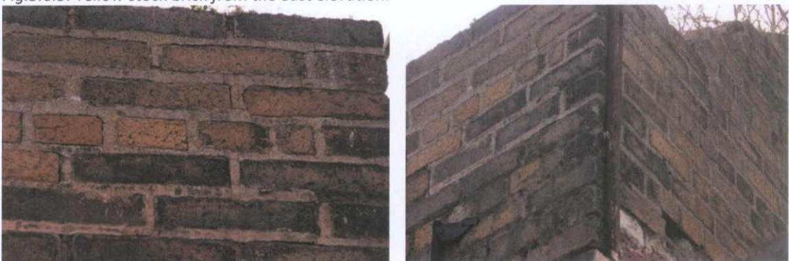
Fig.5.6.6: The yellow stock brick was used for the east (left) and north (right) elevations.
