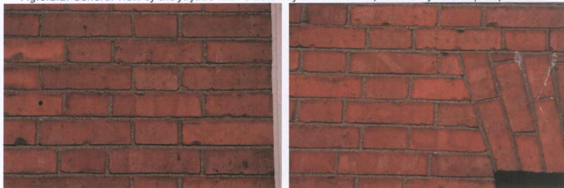
Fig.6.1.2: Detail of the brickwork at the façade, showing 'kiss marks' from the firing process.
