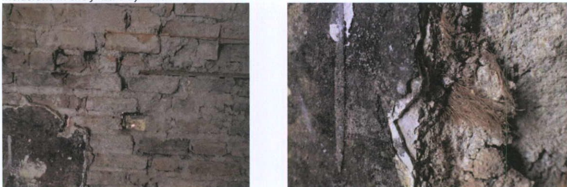
Fig.5.1.9: Internal face of the wall show in Fig.5.1.6 with a change in both brick and mortar at the 'creephole' (left); while the surviving wall plaster has early haired lime plaster layers surviving beneath twentieth century surface finishes (right).
