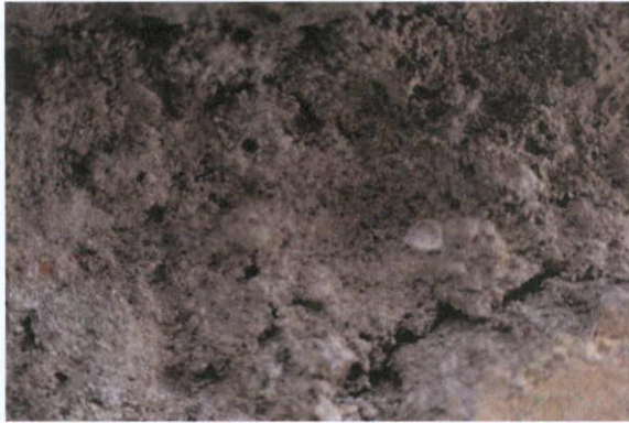
Fig.4.16.10: Cementitious bedding mortar seen externally at the north end of the east elevation.
