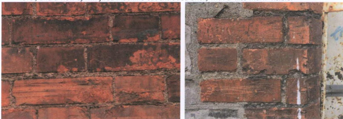
Fig.5.5.4: The brickwork was laid in a lime-based mortar finished flush.
