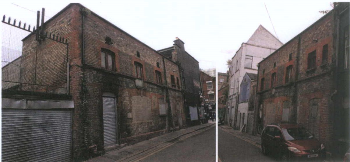
Fig.4.17.1: General view of Nos.11-13 Henry Place.
