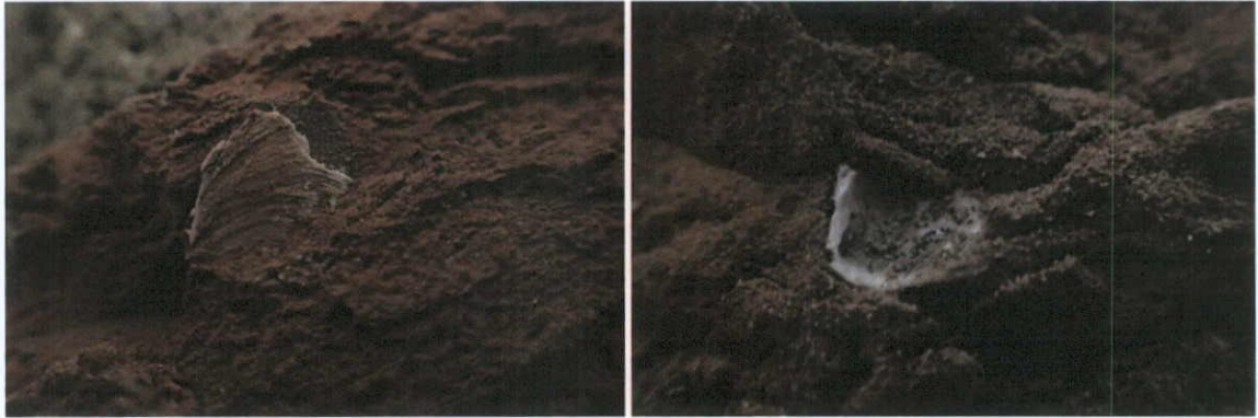
Fig.5.3.3: 13 Moore Street, Ground Floor: Detail of burnt shell inclusions in the brick.
