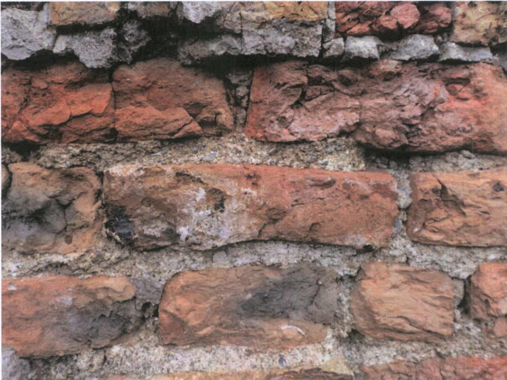
Fig.5.1.7: Detail of north elevation of No.10 Moore Street. The exposed brickwork consists of hand-made clamp-fired bricks showing a lack of sorting of the raw clay material, characteristic moulding and shaping defects, and both underfired and over-fired examples of brick. The bricks do not conform to standard imperial sizing.
