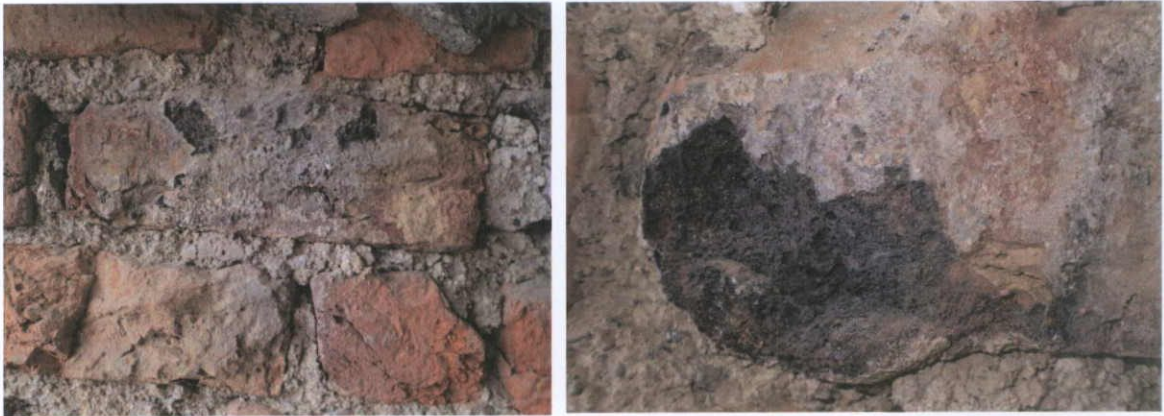
Fig.6.1.7: Many of the bricks were unevenly fired, with sections over-fired and partially vitrified.
