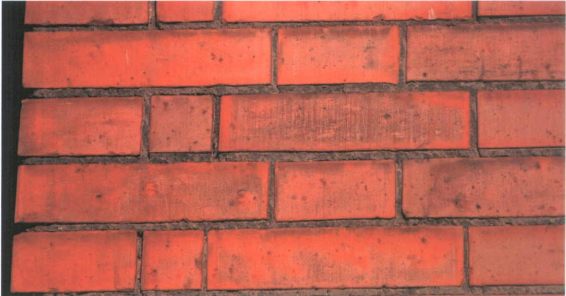
Fig.4.10.2: Machine-cut brick with subtle surface colour variations are characteristic of this brick.
