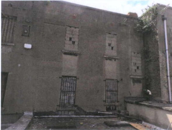
Fig.4.10.3: The rear elevation has a Portland Cement render which has weathered differently to its neighbor, indicating that the cement binders are slightly different in composition.
