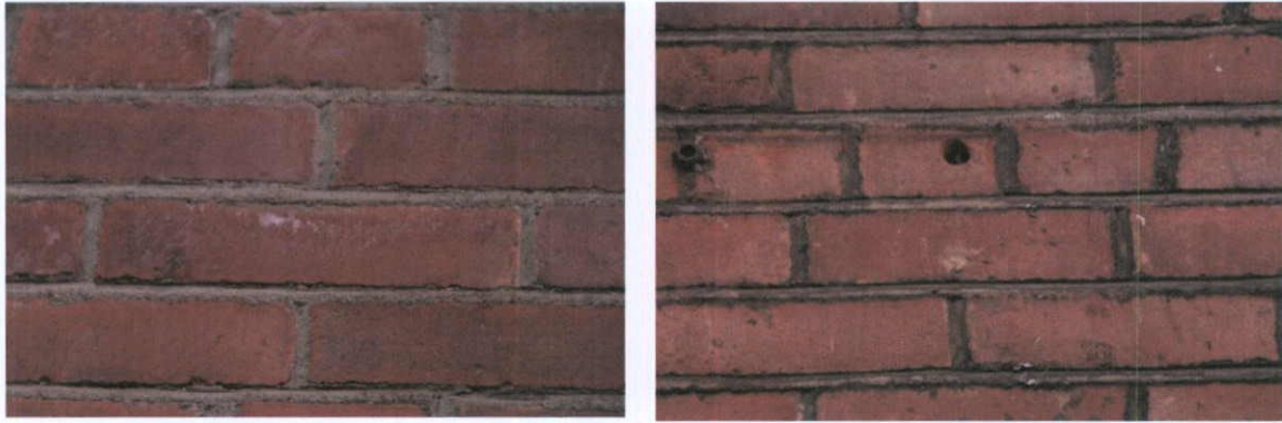
Fig.4.14.5: The brick at first floor level is remarkably free from airborne particulate soiling (which is commonly found on building surfaces which have not been previously cleaned in Dublin City). Some soiling is found on the weatherstruck joints – suggesting that the brickwork was either cleaned (or possibly built) not too long before the Air Pollution Act 1987.
