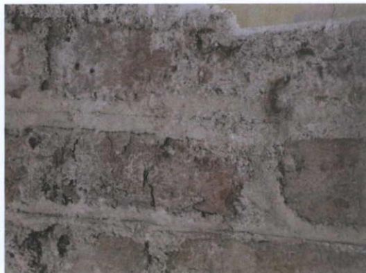
Fig.5.1.10: The party wall between Nos.10 and 11 Moore Street contains early brickwork with lime mortars struck in the same style as the internal walls of the mid-eighteenth century No.42 O'Connell Street.
