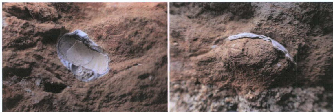
Fig.9.1.2: 'Shell brick' is found at a number of buildings on Moore Street including No.10 Moore
