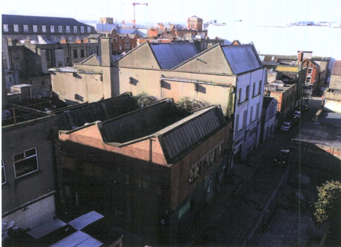
Fig.4.14.1: General view of the building showing a rendered and painted ground floor level, with a brick first floor rising to a sawtooth roof.
