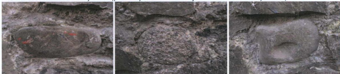
Fig.6.4.3: Rounded cobble-sized limestone is also found in the wall fabric.
