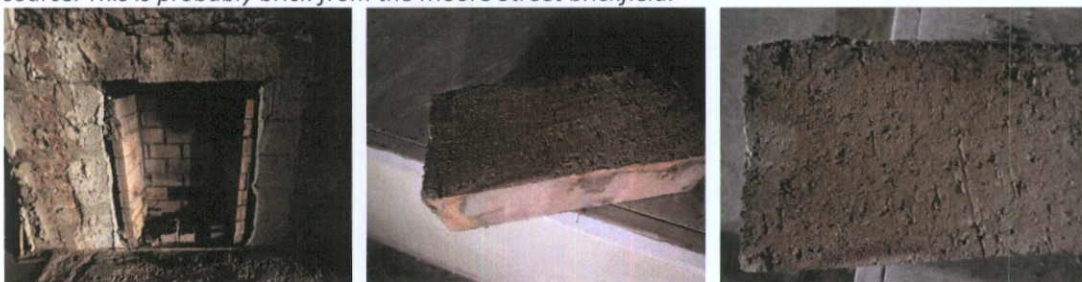
Fig.4.3.11: Wire-cut firebrick at ground floor level, north wall, rear (west) room.
