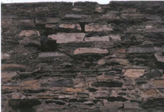
Fig.5.3.28: Calp limestone masonry.
