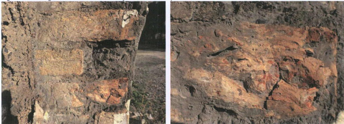
Fig.5.3.5: Detail of yellow stock brick in the chimney stack. The brick retains sedimentary structures indicating hand-made work; but has less inclusions and defects than the brick used for form the joist holes.
