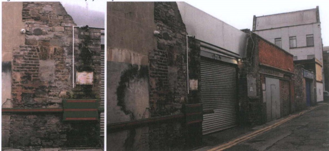
Fig.5.4.2: Calp masonry fabric at the rear of the building with a brick window, and a granite cill.
