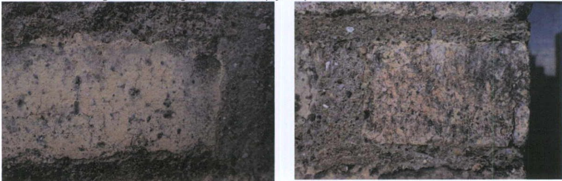
Fig.5.2.11: Detail of 1920s yellow stock brick in cementitious mortar.
