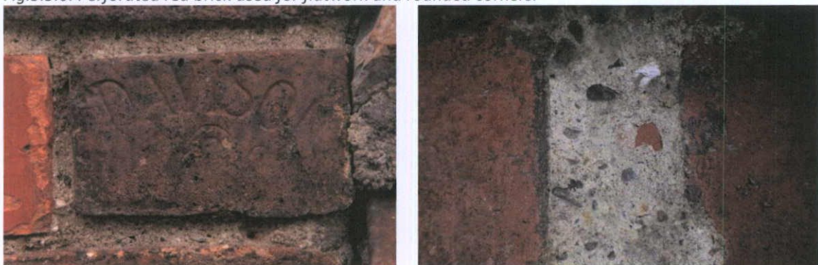
Fig.5.5.7: Brick stamped 'Davison' (left) and detail of the mortar mix containing poorly sorted sub-angular limestone as well as crushed red and yellow brick pozzolan. Charles Davison's Ewloe Barn Brick and Tile Works were active from 1933 to 1951 at Buckley in Flintshire, Wales 2 .
