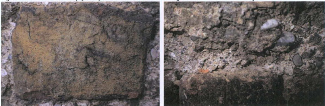
Fig.4.4.6: Clamp-fired yellow stock brick showing shrinkage cracks and over-burnt edges; laid in a coarse-grained lime mortar of rounded limestone pebbles with angular chert and quartzite and crushed brick pozzolan added.
