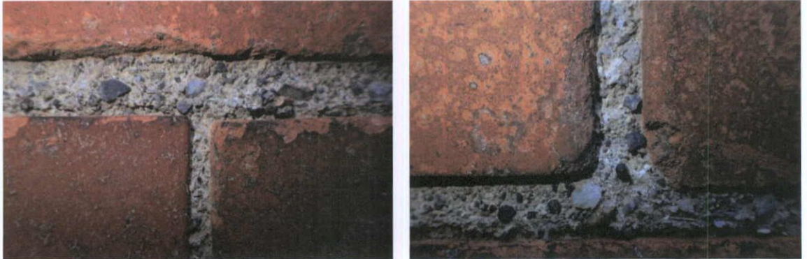
Fig.5.1.5: Coarse-grained lime-cement mortar, c.1920s.
