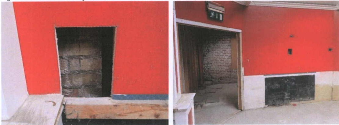
Fig.4.4.2: The brickwork is covered by modern plasterboard.
