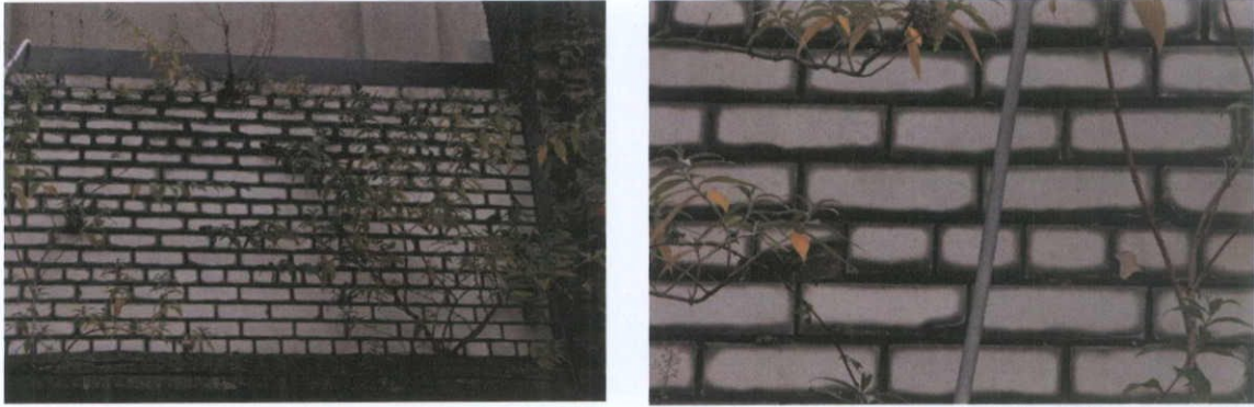
Fig.5.3.24: White glazed 'encaustic' brick which became popular towards the end of the 19 th and early 20 th century for bathrooms, kitchens, high traffic areas and some rear elevations.
