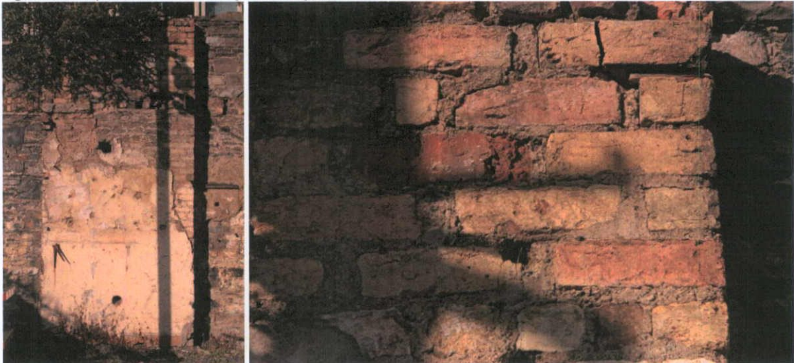
Fig.5.3.4: Fine-grained brick was used for the chimney stack.
