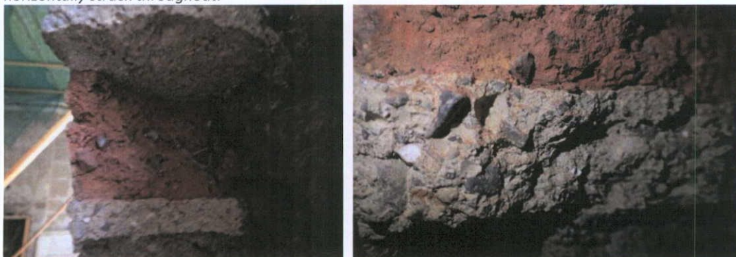
Fig.4.3.10: The large aggregate in the coarse-grained bedding mortars is similar in shape, dimension and mineralogical composition to the stone inclusions seen in the handmade bricks – suggesting a similar source. This is probably brick from the Moore Street brickfield.
