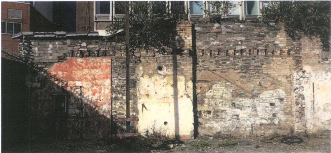
Fig.5.3.1: General view of Building A
