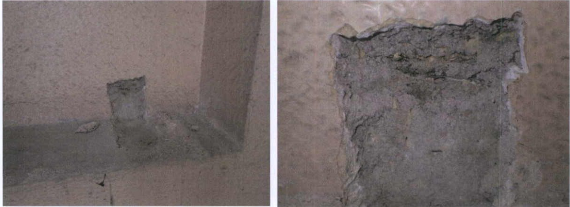
Fig.5.2.16: 1920s yellow stock brick in cementitious mortar exposed in the party walls of the south wall at ground floor level.
