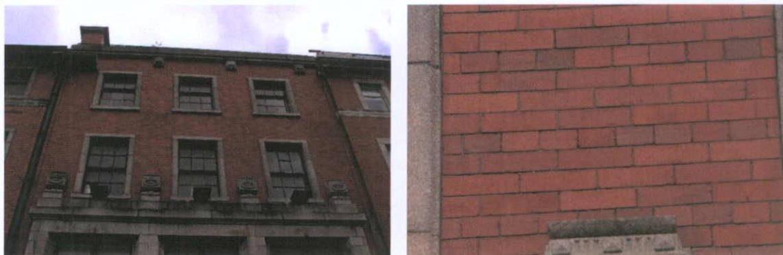
Fig.5.4.1: Brickwork at the façade of 57 O’Connell Street.
