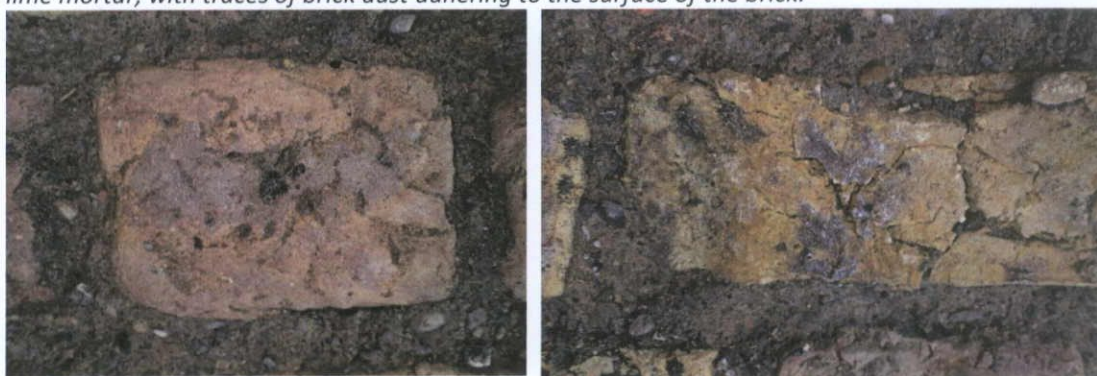
Fig.5.2.5: Stretcher and header views of yellow-pink stock brick with shrinkage cracks laid in coarse-grained pozzolanic lime mortar.
