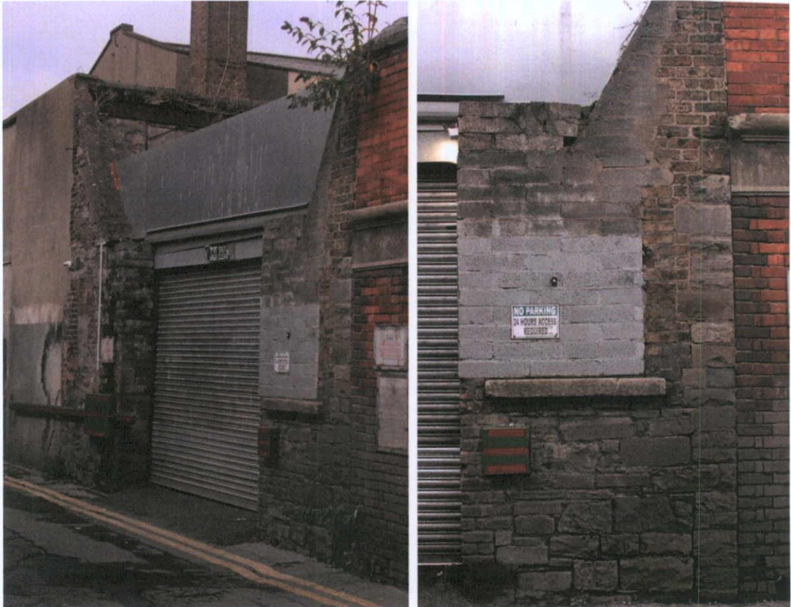
Fig.5.4.3: Detail of coursed hewn Calp masonry and brick fabric.
