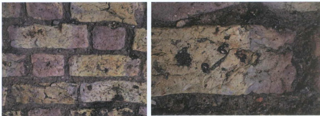
Fig.5.2.4: Detail of yellow-pink clamp-fired stock brick from the basement vaults set in saturated pozzolanic lime mortar; with traces of brick dust adhering to the surface of the brick.
