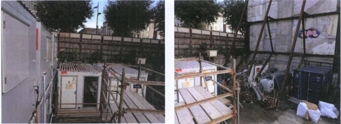
Fig.4.2.2: Reinforced concrete on the east (left) and south (right) boundaries.
