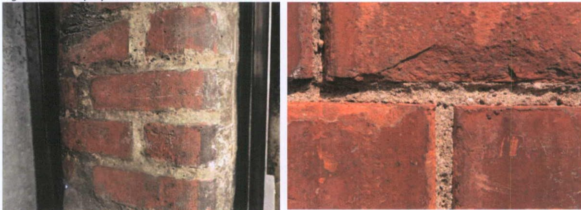
Fig.5.5.6: Perforated red brick used for flatwork and rounded corners.
