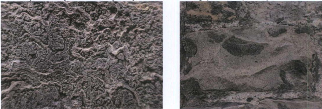
Fig.5.6.7: Black gypsum soiling crusts on the surface of the mortar and stone.
