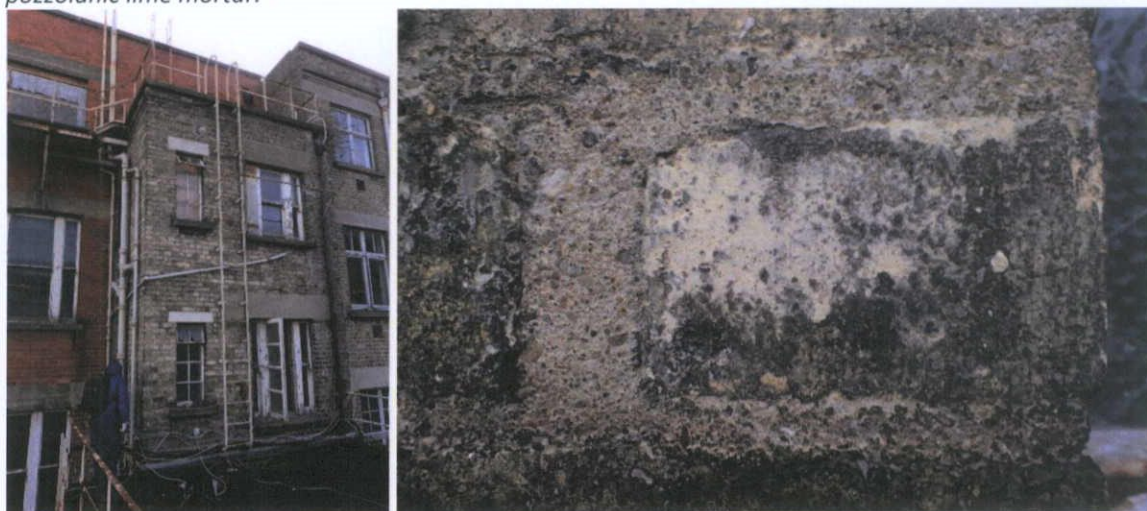
Fig.5.2.6: The return is made from c.1920s yellow stock brick in a lime-cement mortar, with concrete lintels above the openings and forming the parapet coping.
