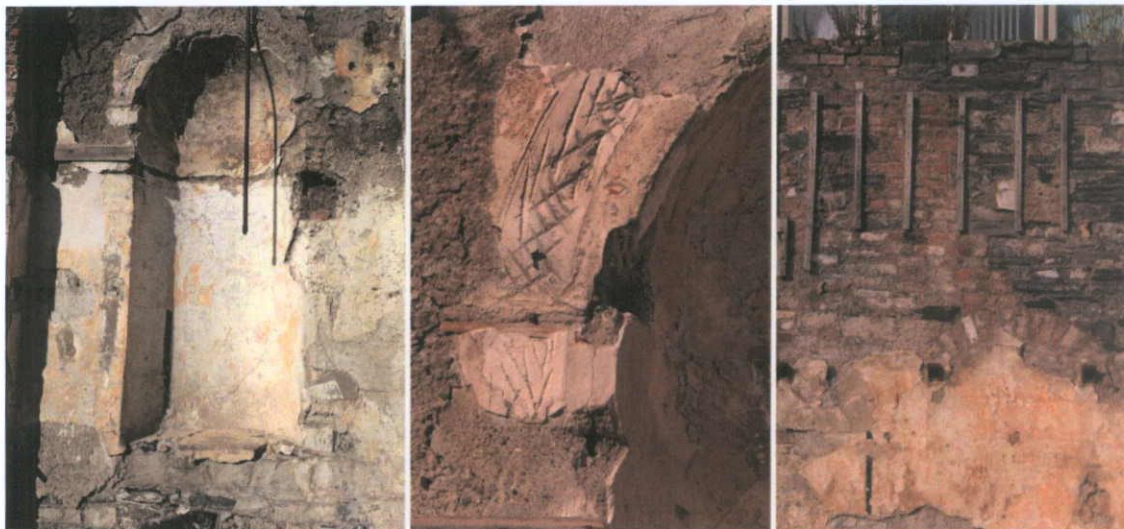
Fig.5.3.13: The western niche retains keying from now-lost embellishment; with timber battens indicating later alteration to the wall surface.
