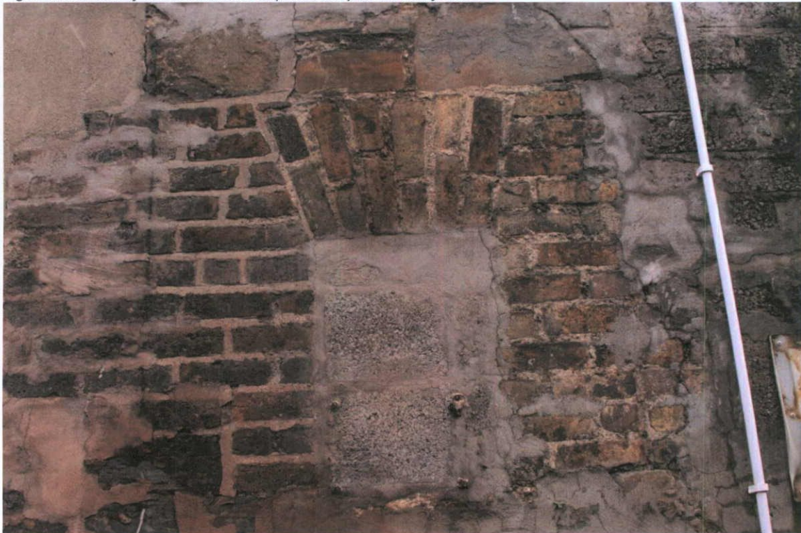
Fig.5.4.4: Detail of the yellow stock brick window.
