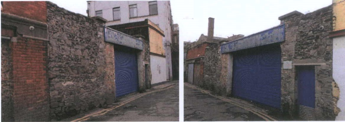
Fig.5.6.1: General view of the Calp limestone masonry wall at the rear of No.59 O'Connell St.
