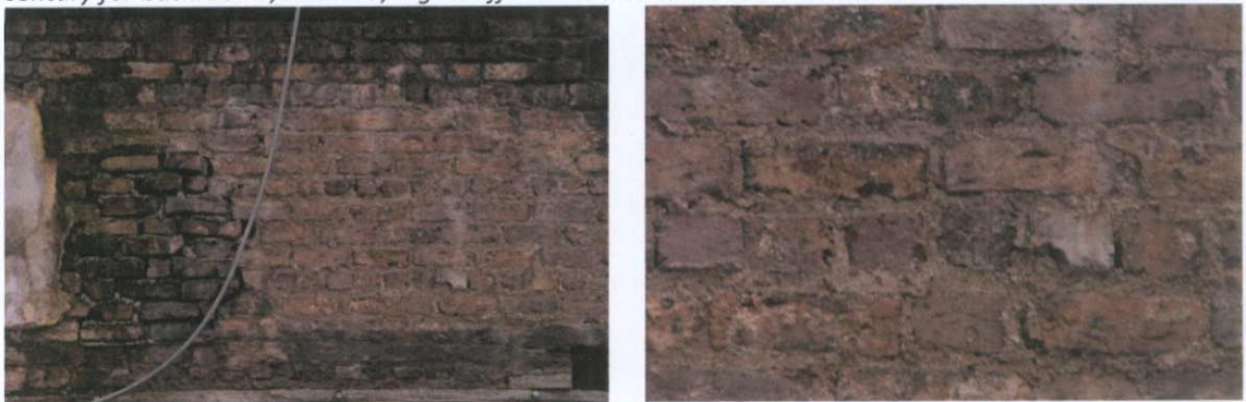
Fig.5.3.25: Yellow stock brick in lime bedding mortar.
