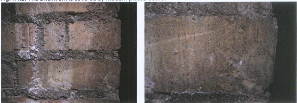
Fig.4.4.3: Yellow machine-cut yellow-stock brick in a lime bedding mortar.
