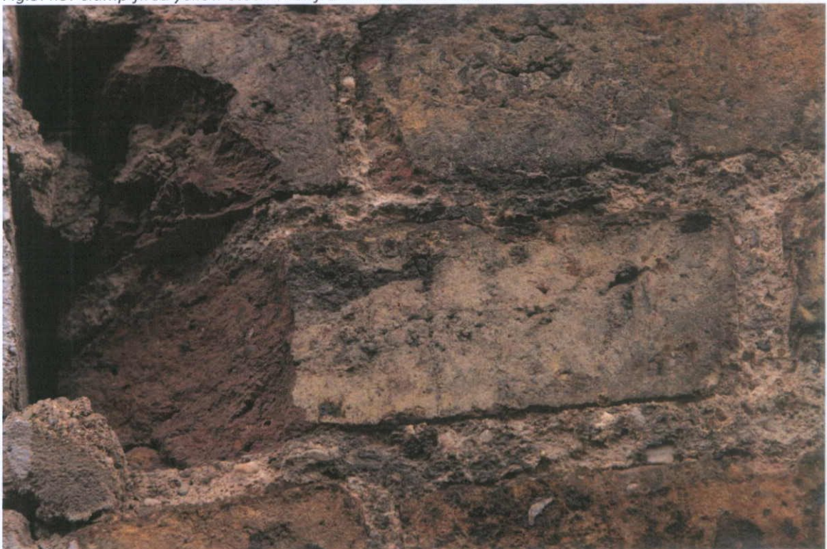
Fig.5.4.6: The yellow colour is confined to the surface, with a spall revealing the red brick core.
