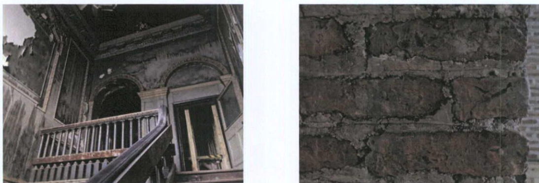
Fig.4.3.8 (left): The internal wall surfaces of the staircase retains decorative plasterwork finishes and enrichment. These were not sampled, but analysis of Georgian plasterwork elsewhere in north Dublin City indicates that the flatwork and the enrichment are composed of different materials – each of which uses very high-grade components and required a great deal of craftsmanship in successful execution.
