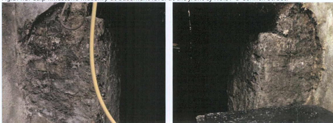
Fig.5.4.9: Detail of Calp limestone bedded in lime mortar at the front of No.57 O'Connell Street.
