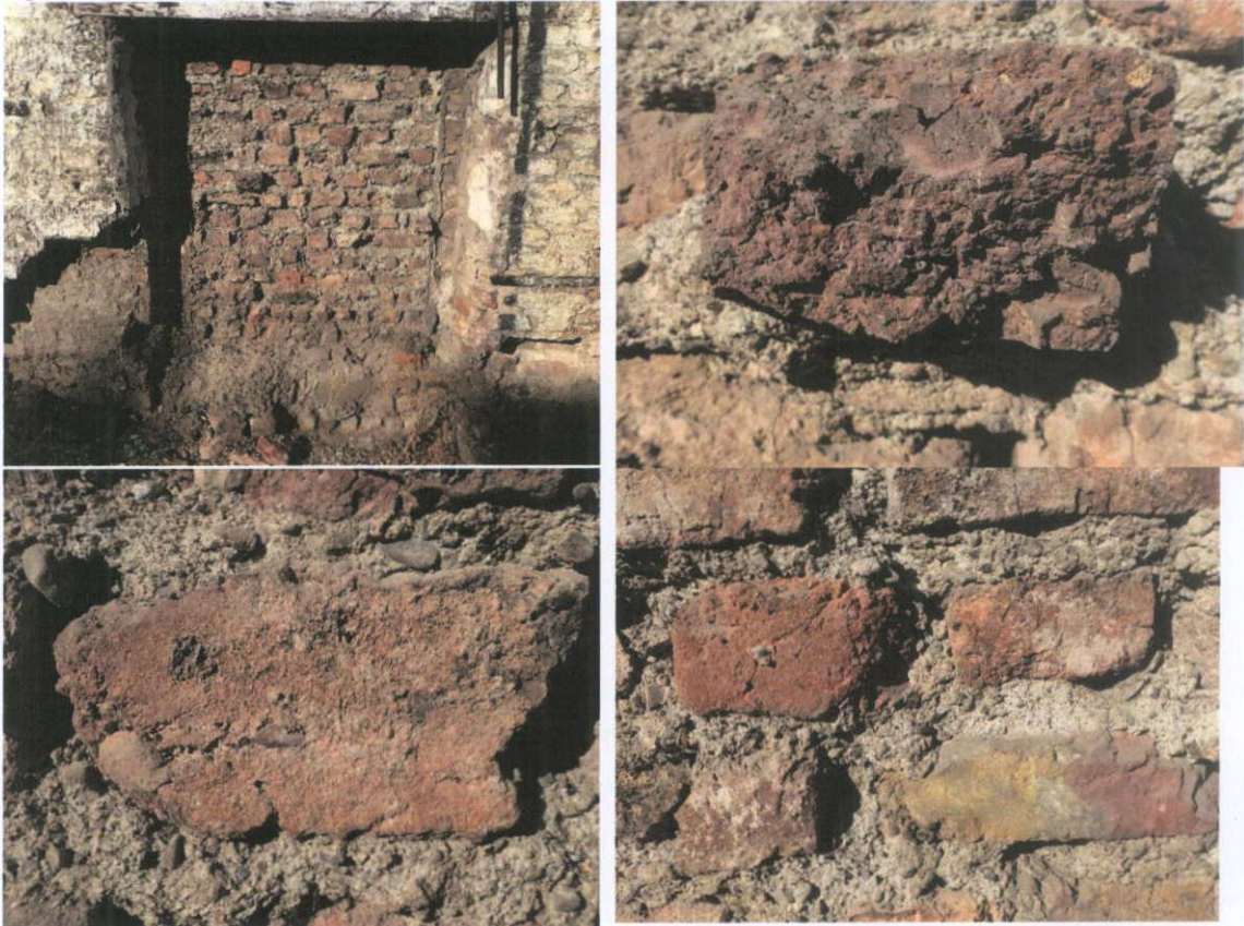
Fig.5.3.20: Irregular clamp fired brick in lime bedding joints infilling a door opening.
