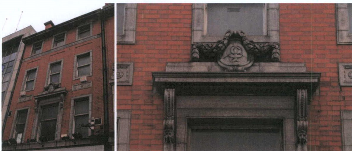
Fig.5.5.1: Granite and brick at the façade.
