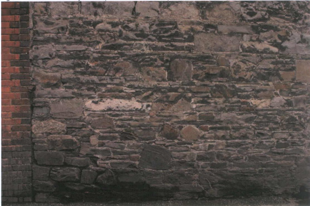
Fig.5.6.2: View of the wall showing flaggy Calp.
