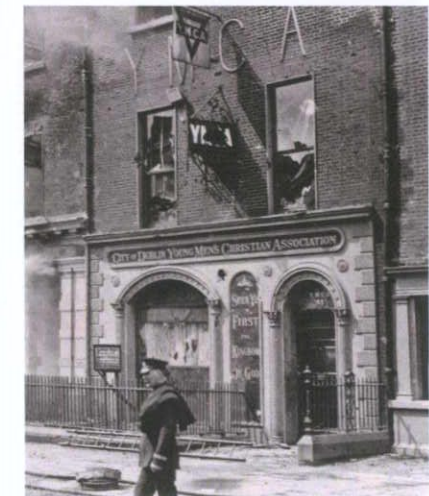
Figure 3: Damage to 43 Sackville Street Upper from fighting in July 1922 (National Library of Ireland)
