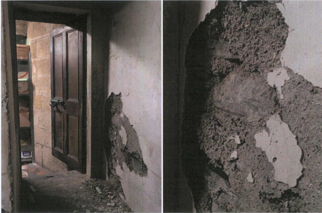
Fig.5.7.8: Detail of the entrance to the granite-lined strongroom at the rear of the building, and the Calp limestone masonry forming the north wall at basement level (right).
