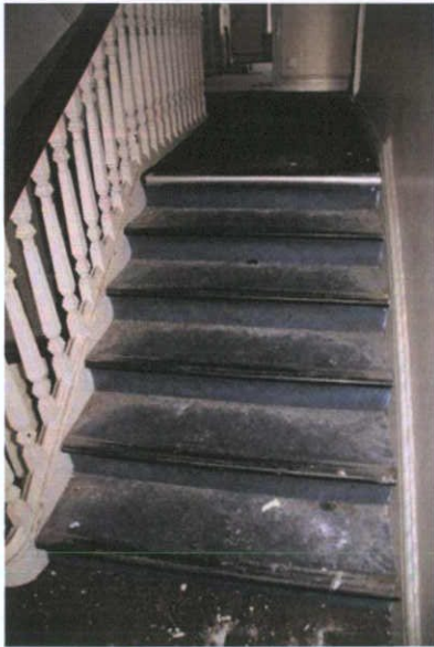
Plate 114: T-1 – View to east
