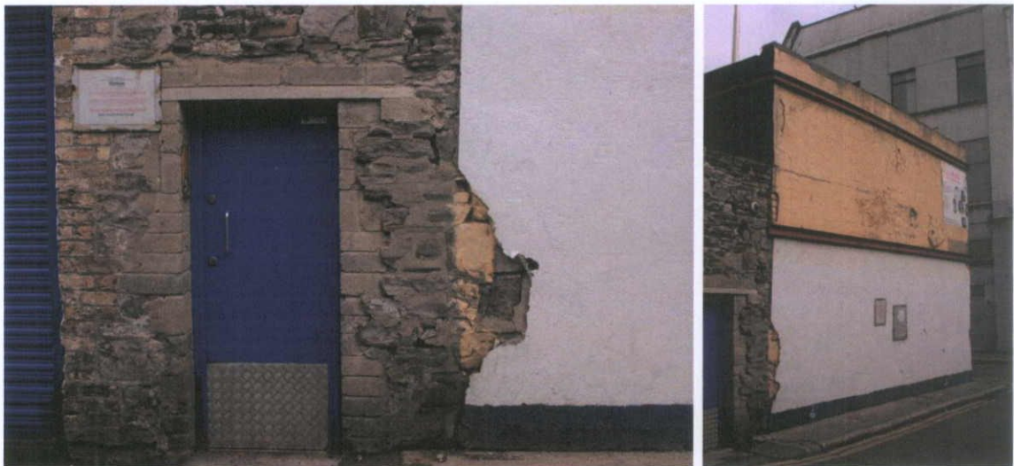
Fig.5.8.1: The rear boundary Calp limestone wall (60a O’Connell Street) is set in a pozzolanic lime mortar similar to others seen along the lane, and is probably eighteenth century Georgian fabric.
