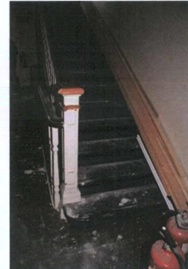
Plate 89: F-5 – First floor landing
