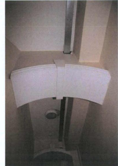
Plate 69: F-4 – Archway over entry hall
