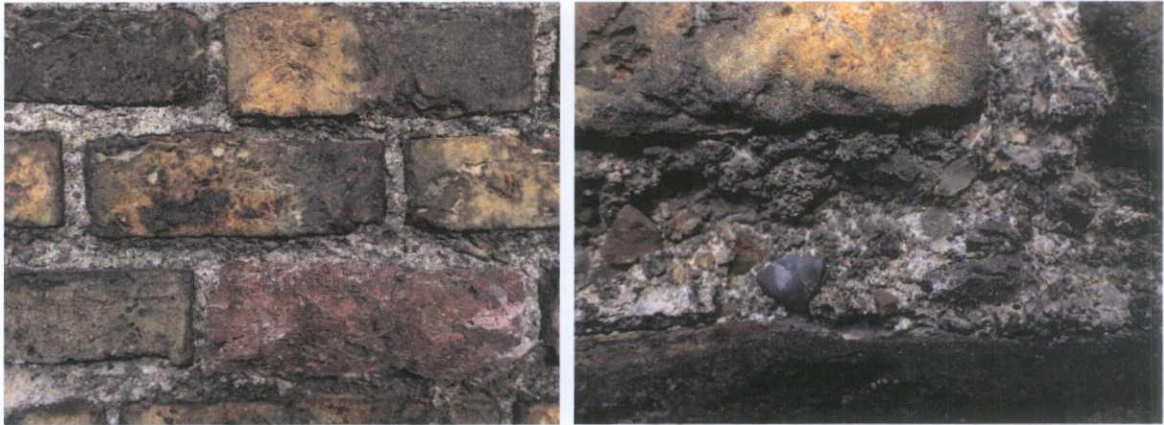
Fig.5.7.16: The soiled party wall is composed of hand-made clamp-fired yellow stock brick bedded in deep coarse-grained lime mortars with scarce crushed brick. This brick is very similar to that transported to Dublin City along the canal networks, and probably mid-nineteenth century.
