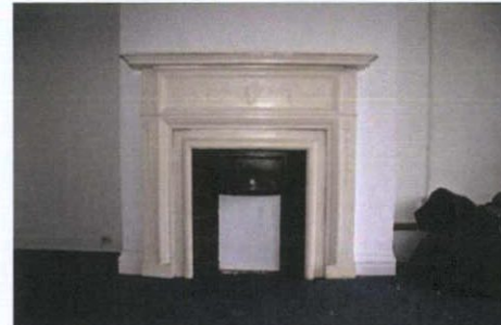
Plate 100: S-3 – Original cast-iron chimney piece to north
