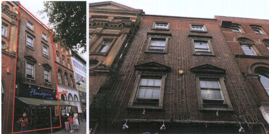
Fig.5.9.1: General view showing the altered upper floor level.
