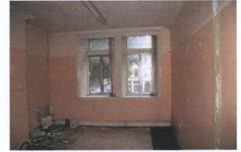
Plate 85: F-9 – View to east
