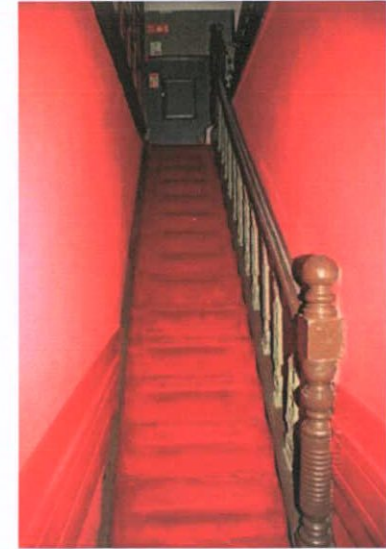
Plate 57: G-7 – View to south; original staircase to first floor
