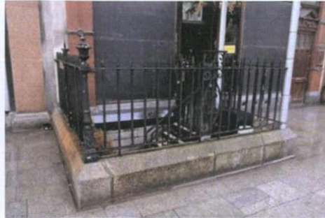
Plate 11: Railings to basement well
