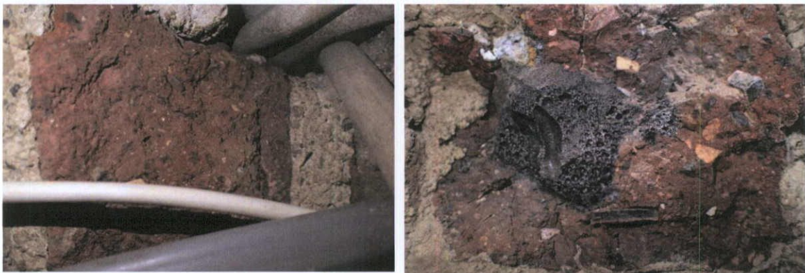
Fig.9.1.1: Brick with coarse angular limestone inclusions from the basement of No.43 O’Connell Street (left), and seen in the internal walls of No.71 Parnell Street (right).
