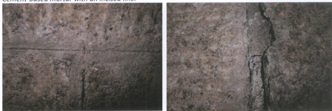
Fig.5.7.11: Detail of the joints of the granite ashlar in the strong room showing the lime bedding mortar beneath the later Portland Cement pointing.
