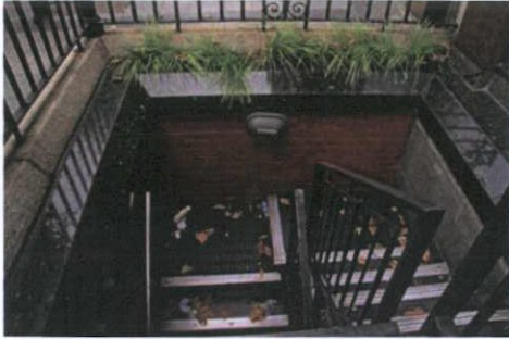
Plate 10: B-1 – View south into basement well
