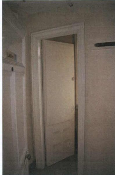
Plate 92: S-2 – View to south-west
