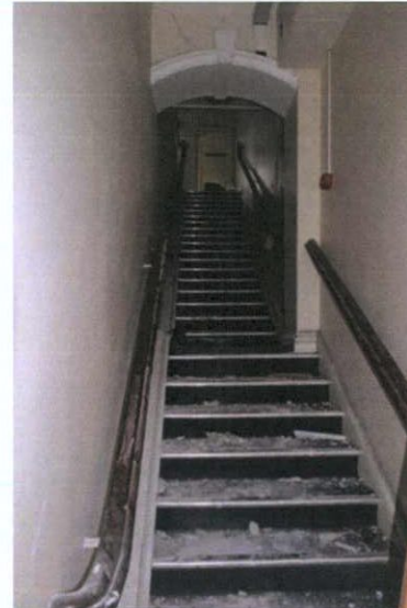
Plate 68: F-4 – View to west
