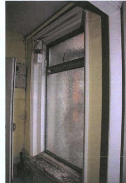
Plate 73: F-6 – View to south
