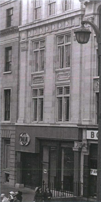
Figure 1: Façade c1960s showing earlier shopfront
