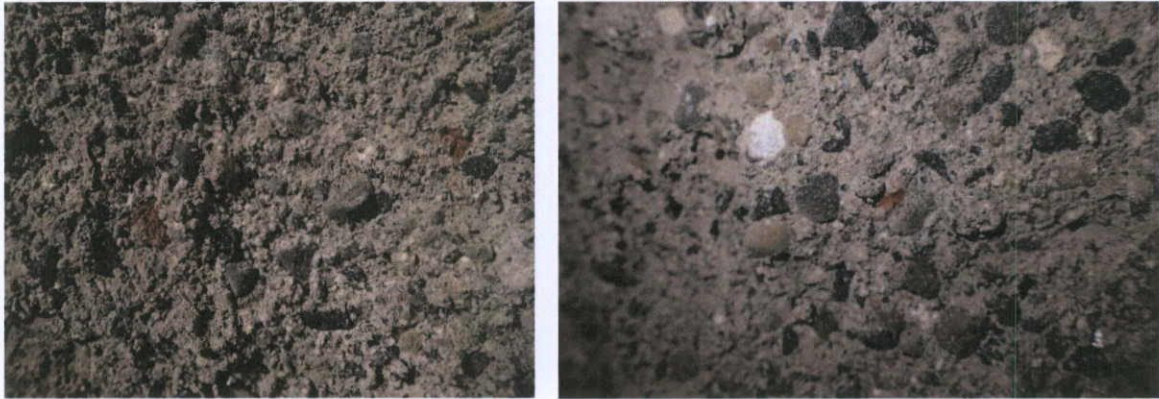
Fig.5.7.9: The render on the north wall of the building is reasonably similar in texture and composition to that found on the south wall. These may be Georgian period building.
