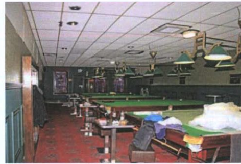
Plate 63: F-3 – View to north-west
