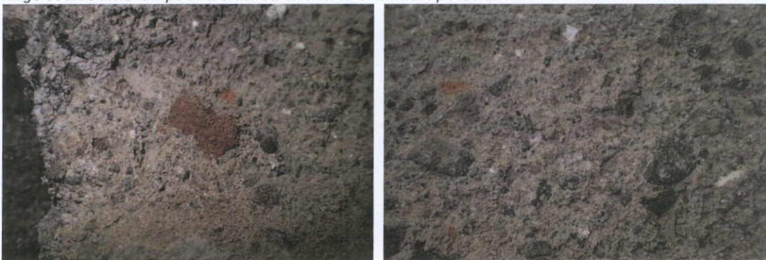
Fig.5.7.7: Limestone aggregate with large coarse lime lumps and crushed brick and brick dust pozzolan on the lime render over the southern basement Calp limestone wall at the front of the building.
