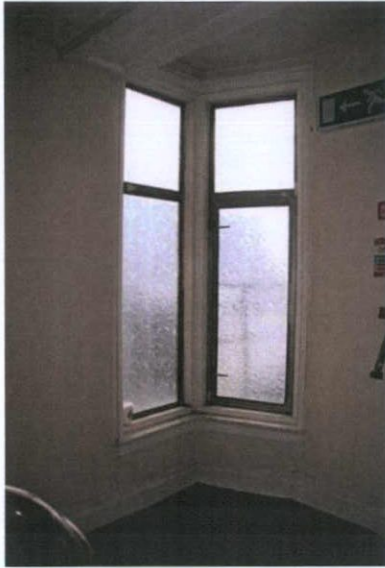
Plate 90: S-1 – Second floor landing
