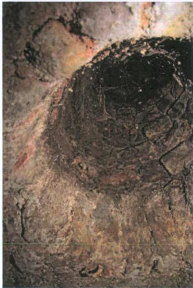
Plate 37: B-9 – Coal hole access to ceiling
