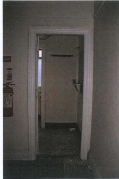
Plate 91: S-1 – View to west towards Room S-2
