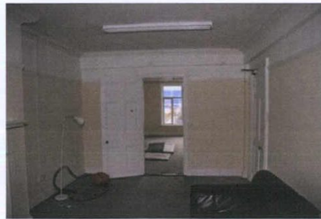
Plate 103: S-4 – View to west
