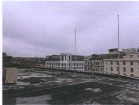
Plate 12: East roof — East 3
