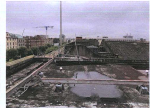
Plate 22: East roof — South 2
