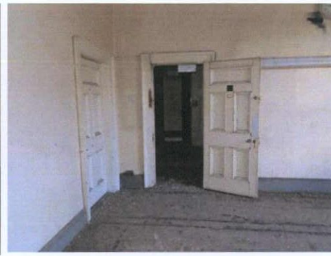
Plate 73: S-3 – View to south
