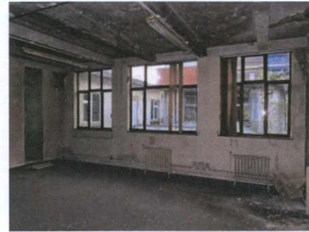
Plate 71: F-9 – View to west
