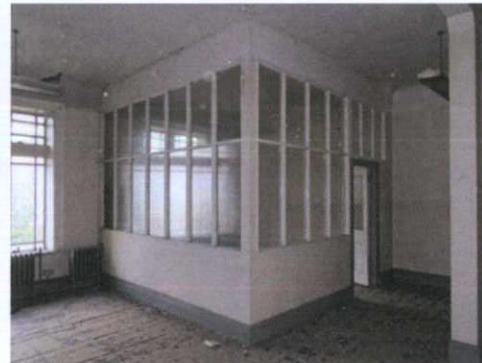
Plate 77: S-4 – View to south-east towards Room S-5; non-original subdivision of room
