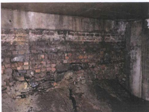
Plate 38: Brick and limestone wall in basement
