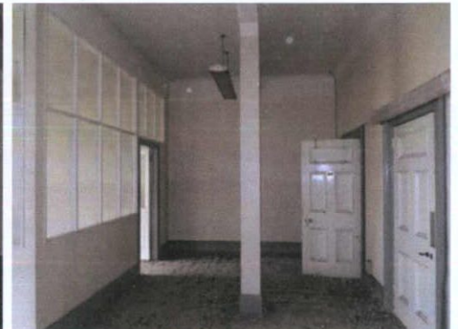
Plate 78: S-4 – View to south
