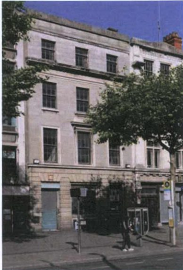
Plate 2: Front (east) elevation
