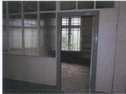
Plate 81: S-5 – Entrance to front room; non-original partition
