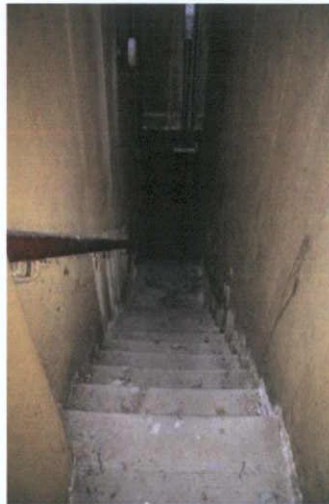
Plate 39: G-7 – View to east towards Room B-1
