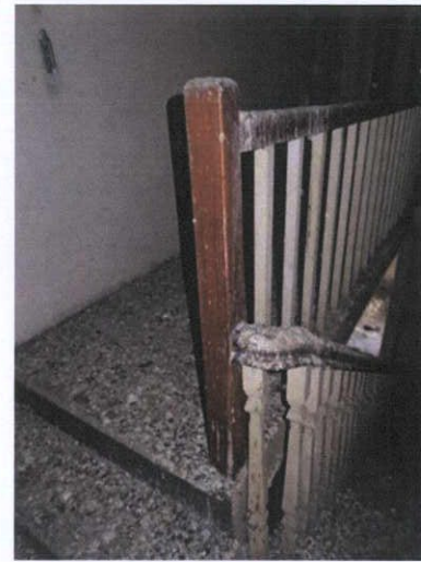
Plate 87: T-1 – View to south-west from third floor landing
