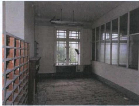
Plate 76: S-4 – View to east
