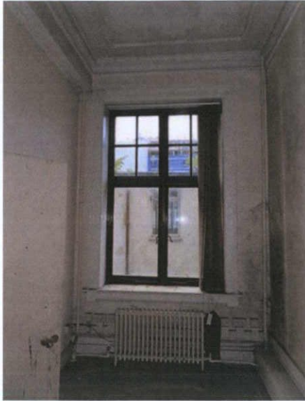
Plate 61: F-4 – View to west
