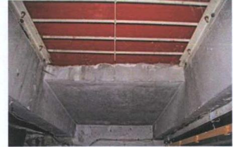
Plate 21: B-8 – View to ceiling
