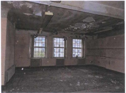
Plate 97: T-4 – View to east
