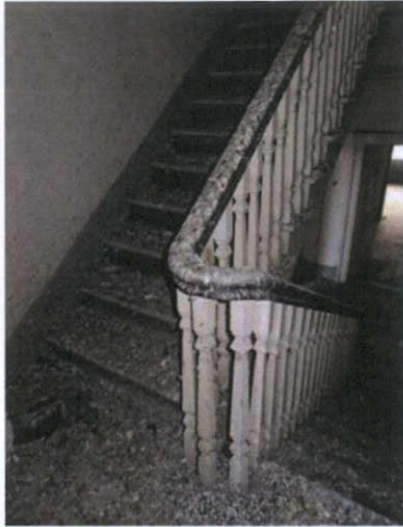
Plate 63: S-1 – View to east from half-landing
