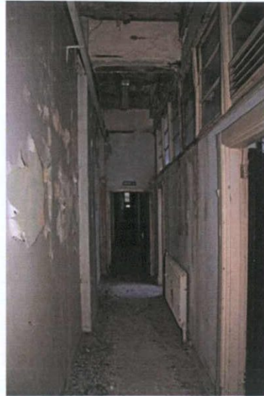
Plate 46: G-11 – View to west
