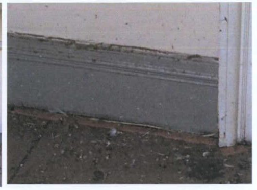
Plate 74: S-3 – Original skirting boards
