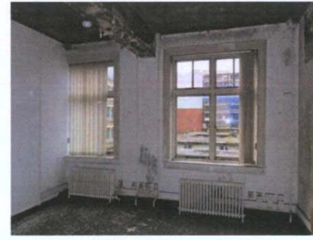
Plate 81: S-3 – View to west; non-original partition to south (left)
