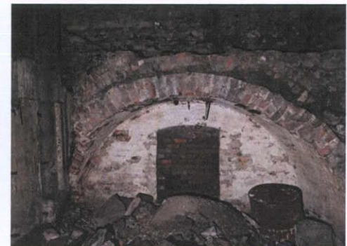
Plate 33: Broken end of brick vault
