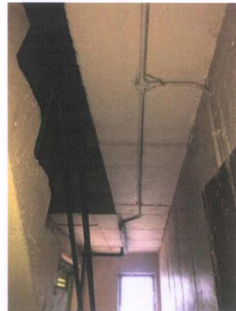
Plate 15: Ceiling of hallway
