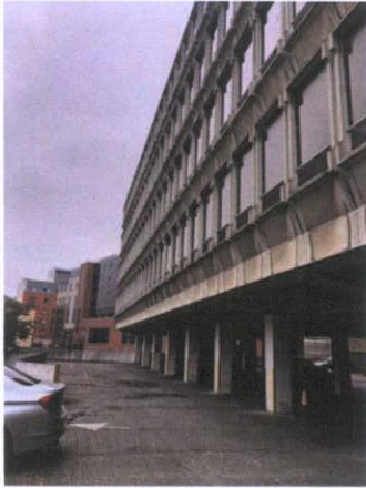
Plate 10: View from car park — View to west
