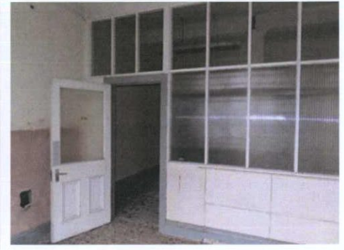
Plate 82: S-5 – View to south-west
