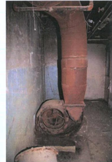
Plate 25: B-10 – View to west
