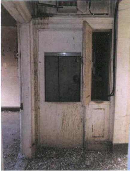
Plate 94: T-4 – View to north; dumbwaiter
