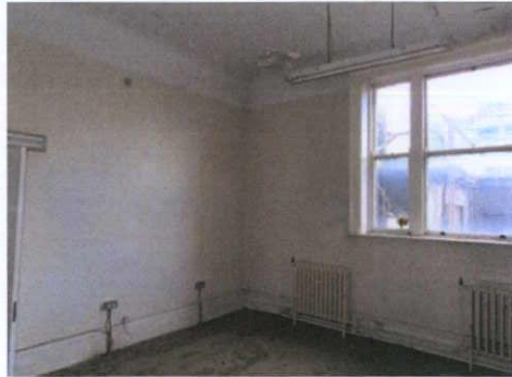
Plate 54: F-5 – View to south-west; Wyatt window
