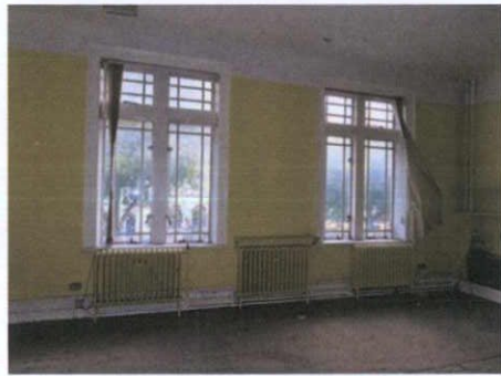
Plate 58: F-6 – View to east
