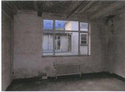
Plate 69: F-8 – View to west
