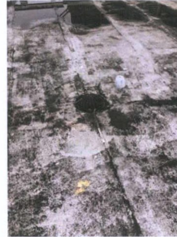
Plate 12: East roof — Drain
