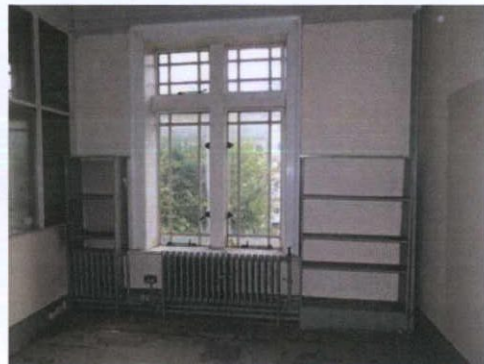
Plate 84: S-5 – View to east
