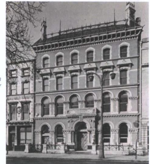
Figure 2: Numbers 46 to 48 O'Connell Street Upper
