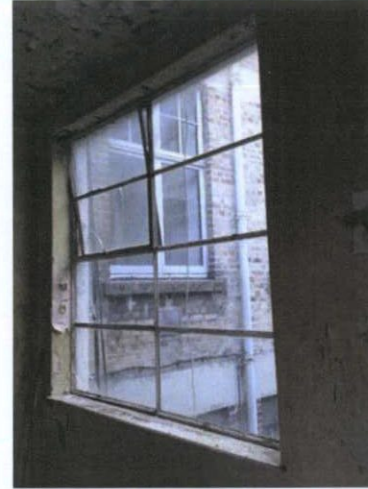
Plate 48: F-1 - View to north-east; steel pivot window
