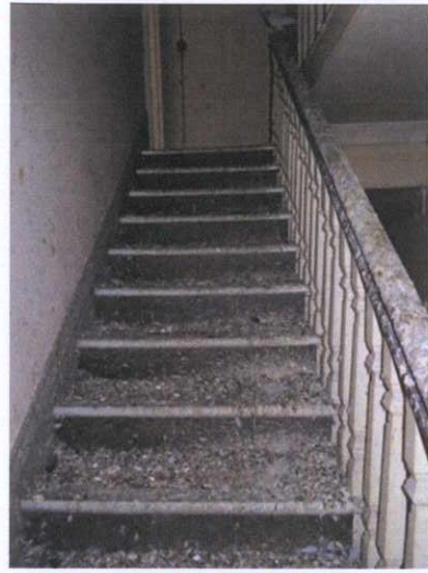
Plate 86: T-1 – View to east
