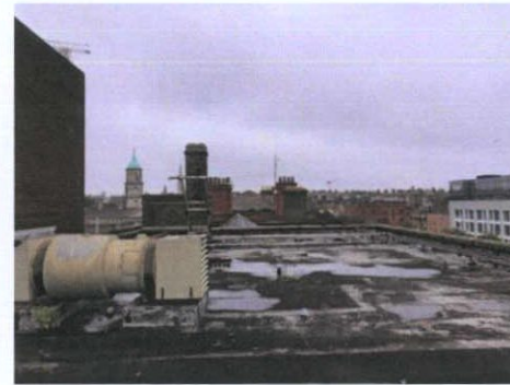
Plate 12: East roof — North
