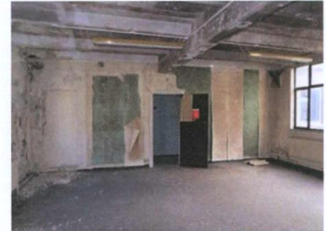
Plate 72: F-9 – View to south
