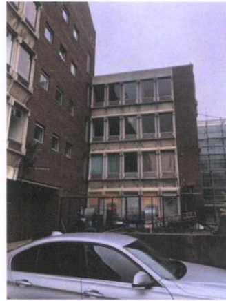
Plate 11: Rear of building view from car park — View to east
