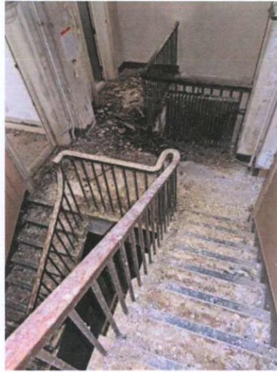
Plate 54: F-1 – View to south
