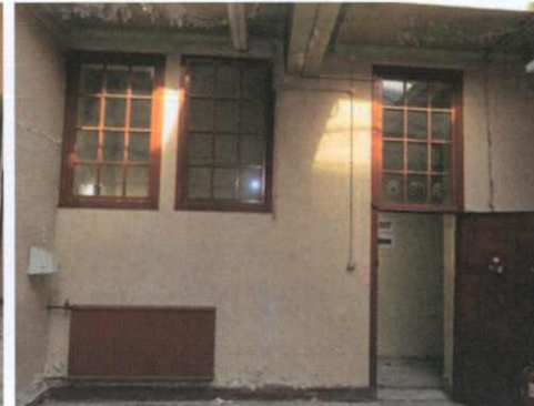
Plate 44: G-9 – View to north
