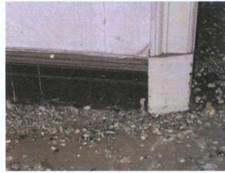
Plate 80: S-2 – Original skirting board
