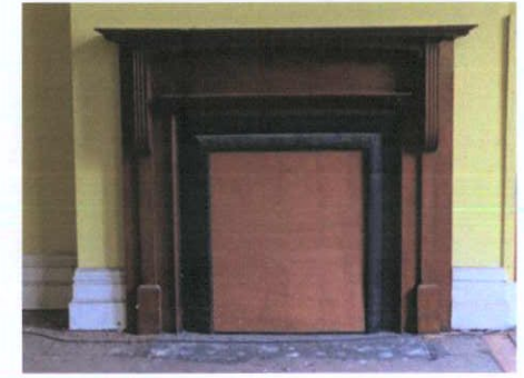
Plate 61: F-6 – Timber chimneypiece with cast-iron insert
