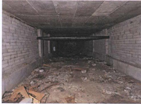
Plate 30: Concrete rising walls in basement
