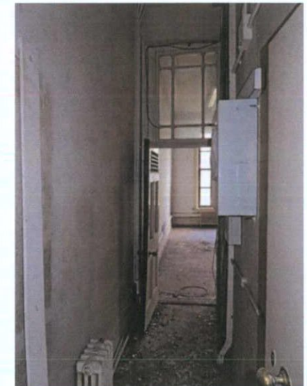
Plate 60: F-3 – View to east
