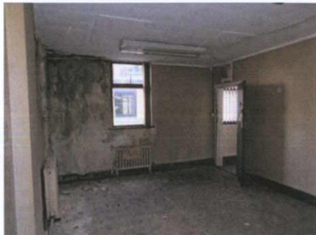
Plate 73: F-10 – View to east
