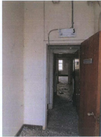
Plate 85: S-4 – View to east
