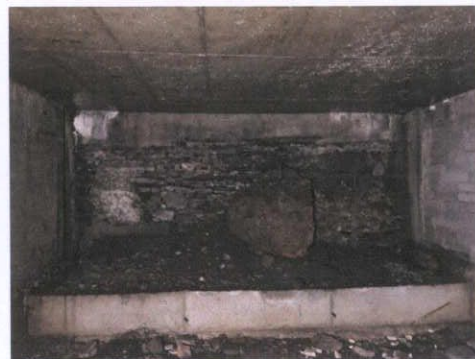
Plate 39: Limestone wall in basement
