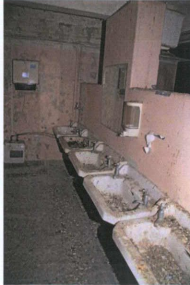
Plate 27: B-12 – View to west
