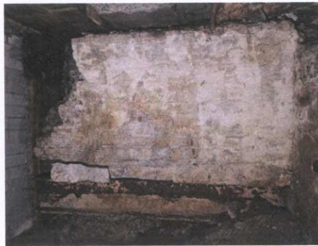
Plate 40: Limewashed wall in basement
