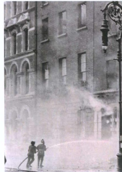
Figure 3: 45 O'Connell Street Upper gutted by fire
