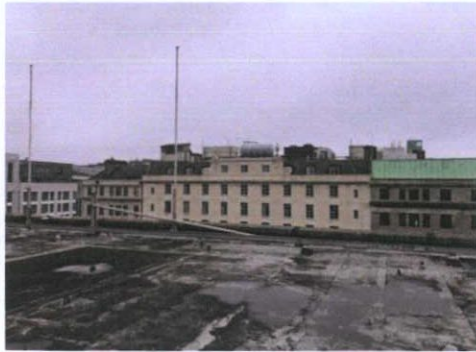
Plate 11: East roof — East 2
