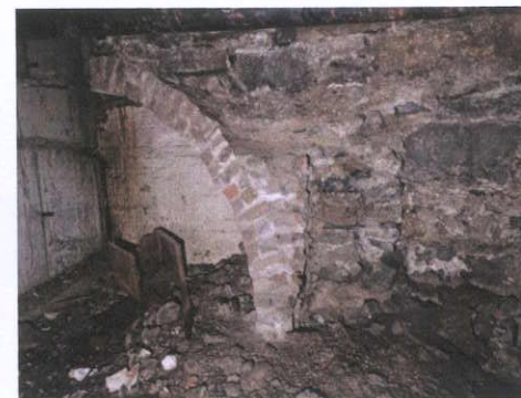
Plate 41: Vault and masonry in basement
