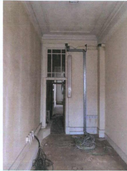
Plate 62: F-4 – View to east
