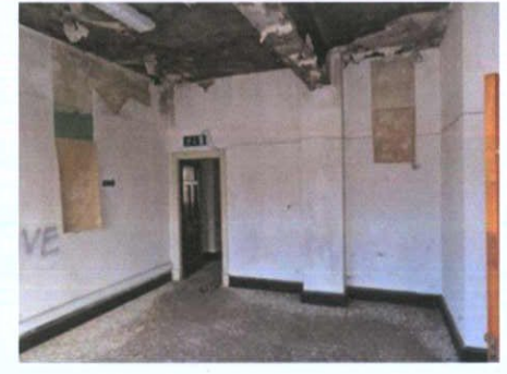
Plate 82: S-3 – View to east
