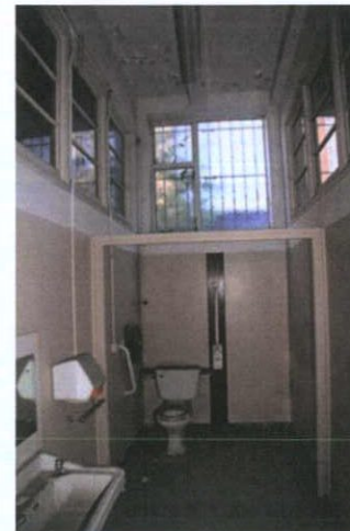
Plate 51: G-14 – View to west
