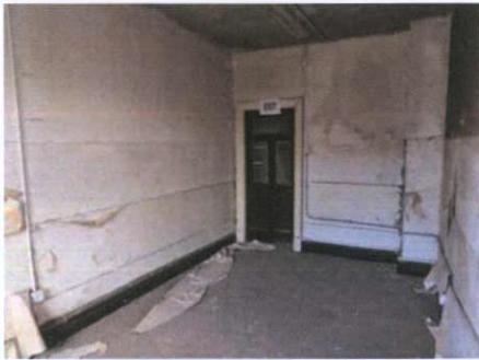
Plate 98: T-7 – View to east
