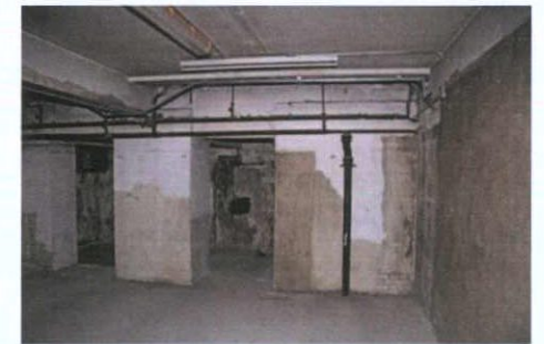
Plate 17: B-5 – View to east
