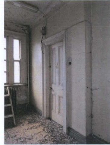
Plate 65: S-1 – Entrance to Room S-2
