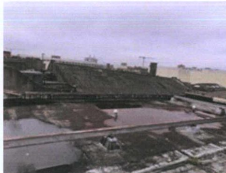
Plate 21: East roof — South 1
