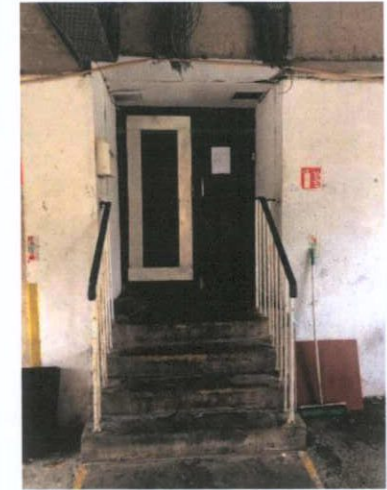
Plate 161: Emergency exit from Level 1 'Fortune Terrace
