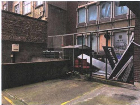
Plate 170: North east area of car park
