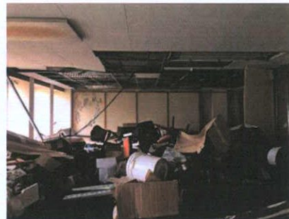
Plate 331: Main room - South wall
