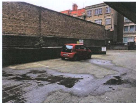
Plate 155: North boundary wall and entrance ramp
