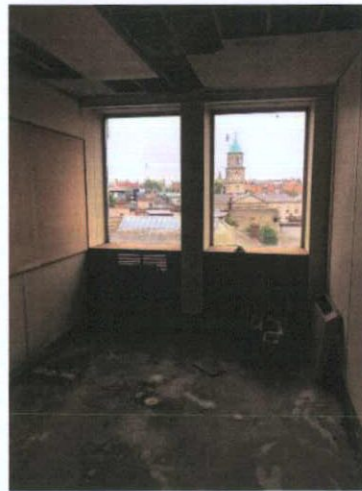
Plate 440: Room 10 — North wall
