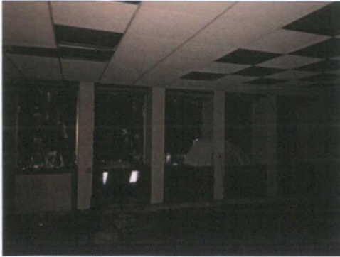
Plate 226: Room 1 — South wall
