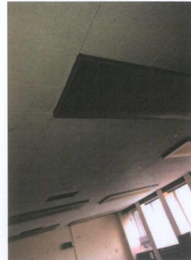
Plate 280: Room 14 — suspended ceiling
