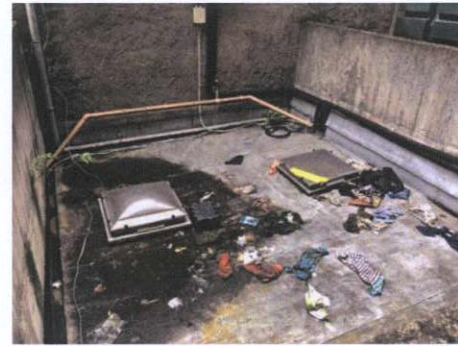
Plate 168: South East area of car park
