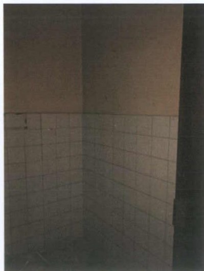
Plate 294: East wall of cleaning closet
