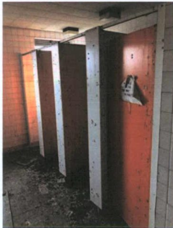
Plate 384: Women's WC cubicles
