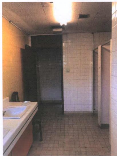
Plate 185: Exit from men's WC
