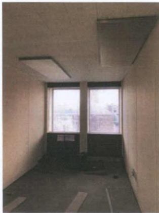
Plate 246: Room 7 — North wall
