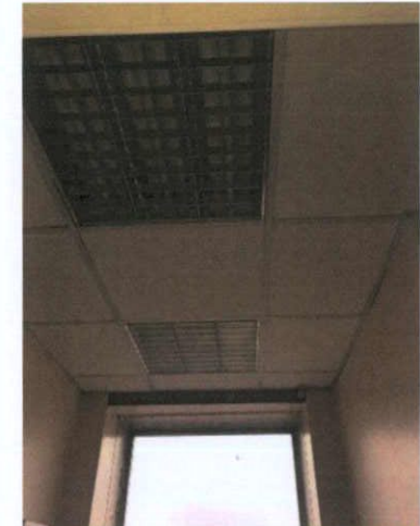
Plate 406: Room 1 — Suspended ceiling
