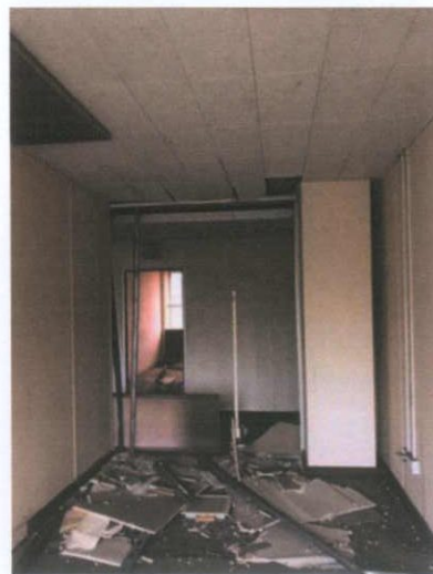
Plate 262: Room 10 — South wall
