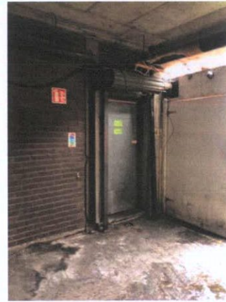
Plate 97: Exit from Pick & Pay shop in south east corner
