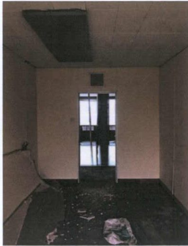
Plate 266: Room 11 — South wall
