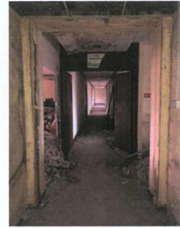
Plate 301: Main corridor facing west
