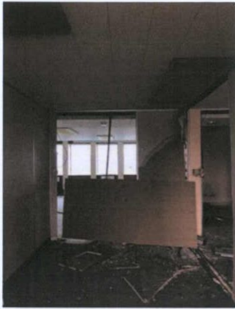
Plate 364: Room 7 — North wall
