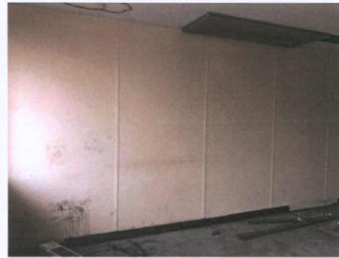
Plate 243: Room 6 — West wall
