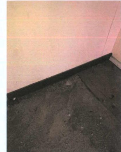
Plate 305: Carpet visible underneath metal stud partitions
