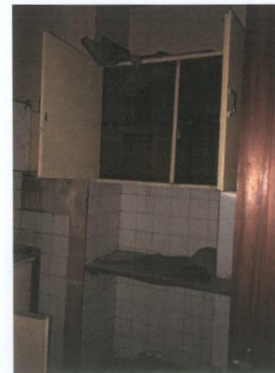
Plate 297: East wall of kitchenette
