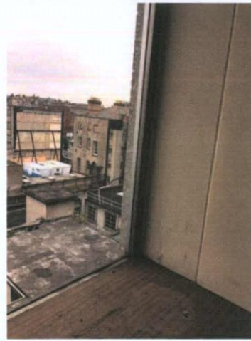
Plate 424: Room 7 — Window detail
