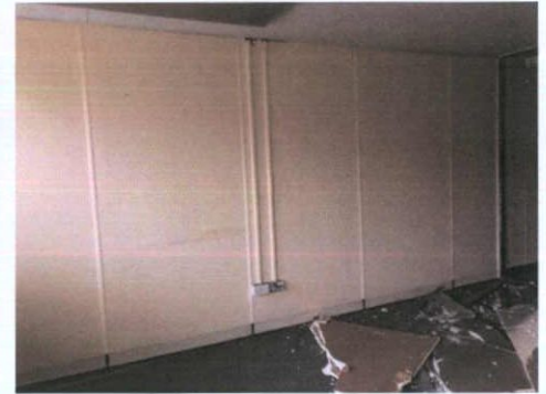
Plate 241: Room 5 — West wall
