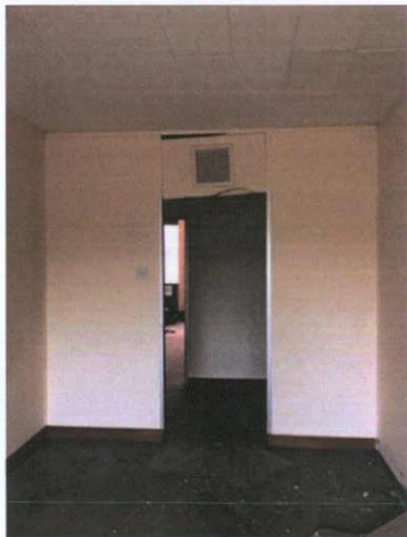
Plate 254: Room 8 — South wall
