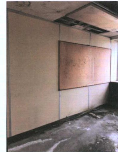
Plate 438: Room 9 — Suspended ceiling damage
