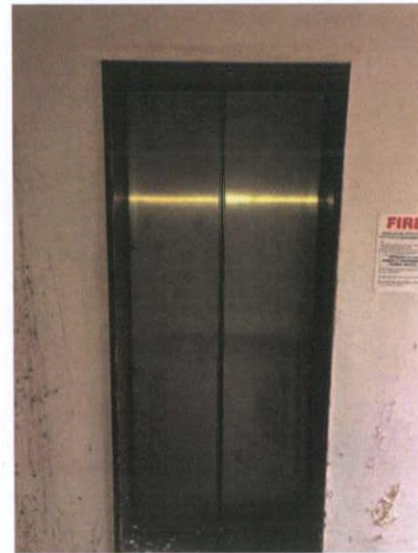
Plate 492: Lift lobby — Door 1
