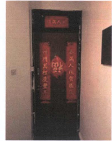
Plate 175: Entrance to floor from stair core
