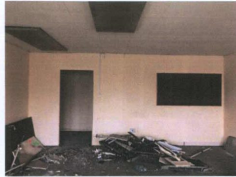
Plate 235: Room 2 — North wall
