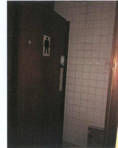
Plate 285: Male WC entrance from main hallway
