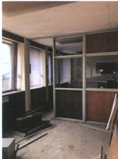
Plate 219: Office behind reception area
