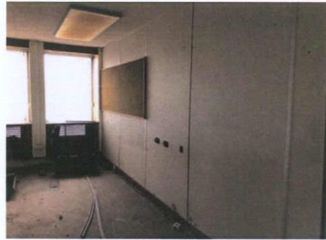
Plate 365: Room 7 — West wall
