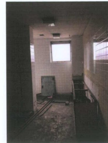
Plate 379: Men's WC wash area
