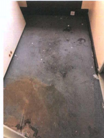
Plate 405: Room 1 — Concrete floor
