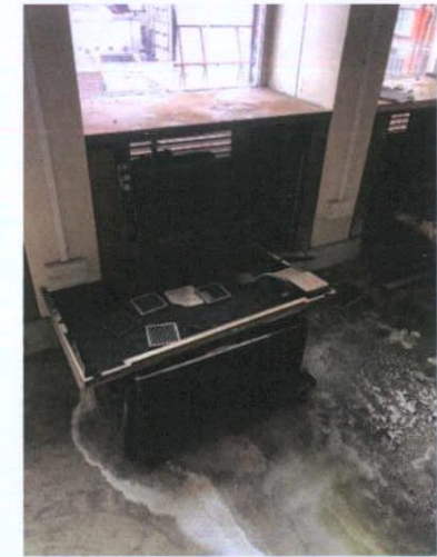
Plate 426: Room 7 — Ventilation units removed
