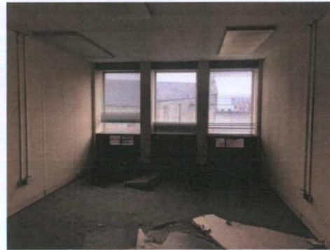
Plate 240: Room 5 — North wall
