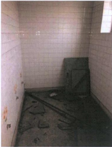
Plate 380: Men's WC urinal area
