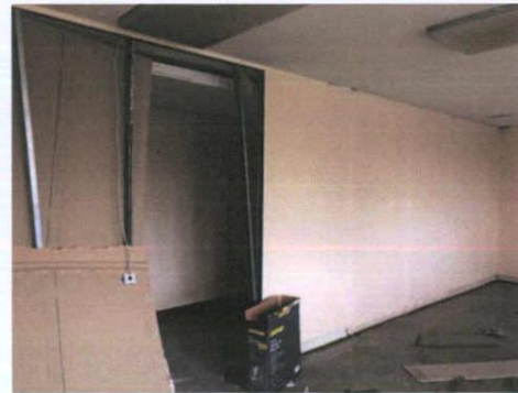
Plate 239: Room 3 — South wall
