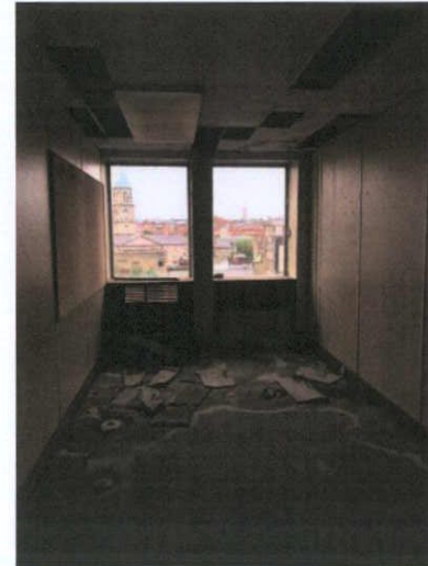
Plate 453: Room 12 — North wall
