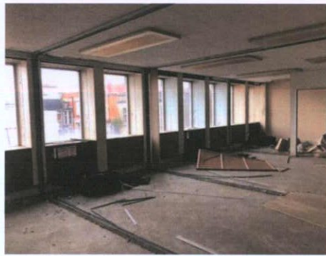
Plate 370: Rooms 13-16 — North wall
