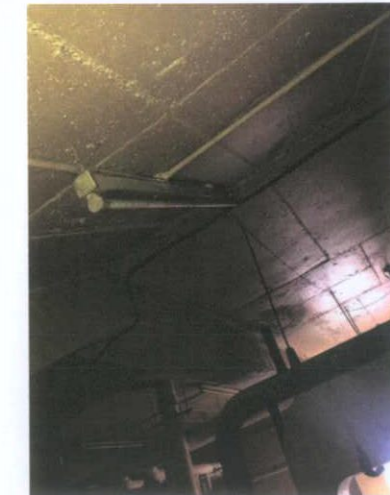
Plate 498: Plant room — Ceiling
