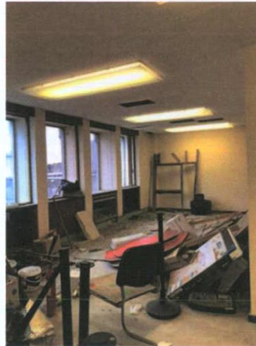
Plate 202: Room partially demolished — West wall
