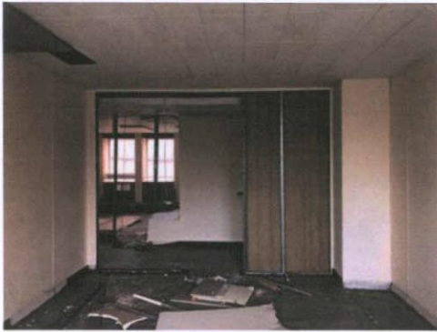
Plate 242: Room 6 — North wall
