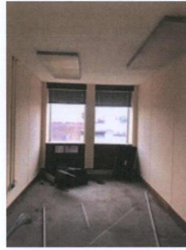
Plate 252: Room 8 — North wall
