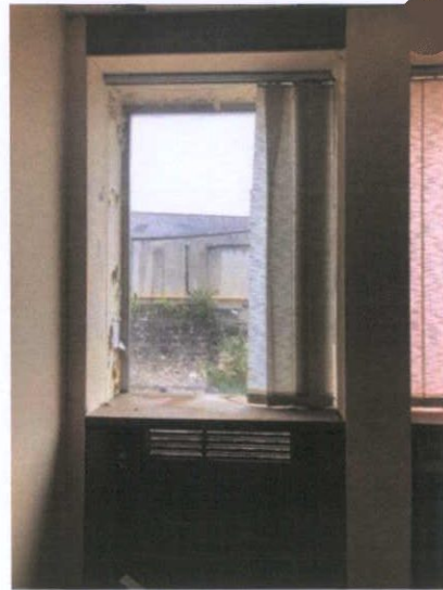
Plate 206: Window in office
