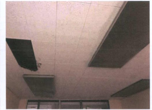
Plate 245: Room 6 — Suspended ceiling
