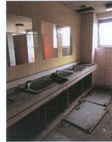
Plate 383: Women's WC wash area
