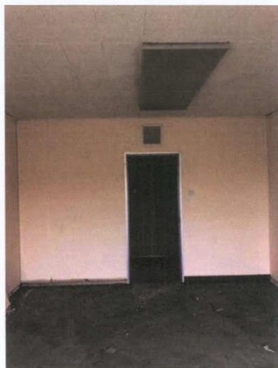
Plate 258: Room 9 — North wall
