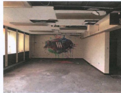
Plate 358: Room 6 — West wall
