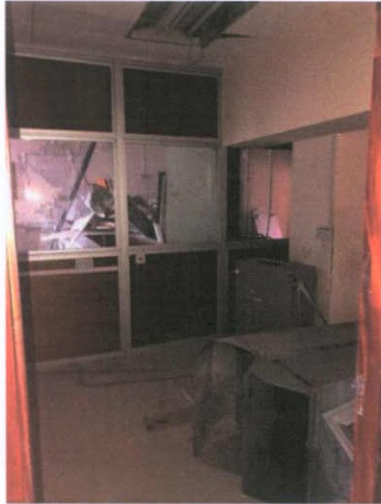
Plate 221: Waiting room next to reception area
