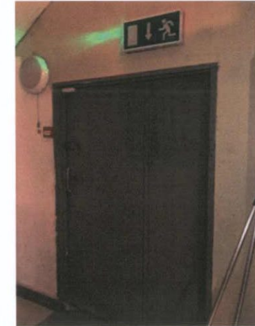
Plate 52: Emergency exit to car park
