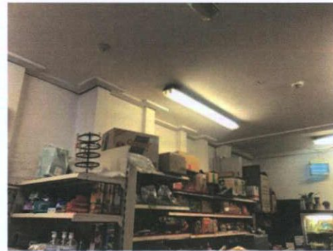
Plate 67: South wall of shop showing door to stock room at the rear; concrete piers around
