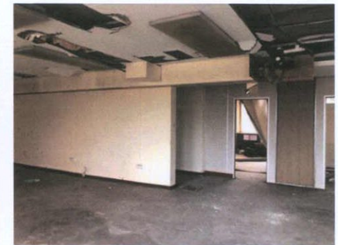
Plate 359: Room 6 — North wall
