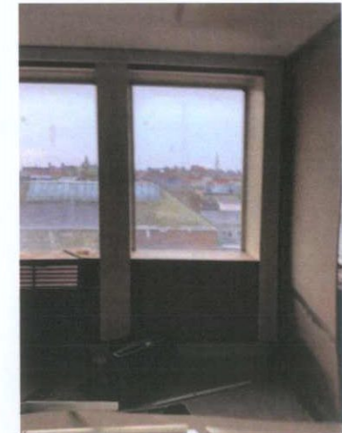
Plate 347: Room 4 — North wall
