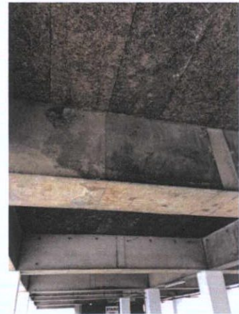
Plate 171: Car park ceiling
