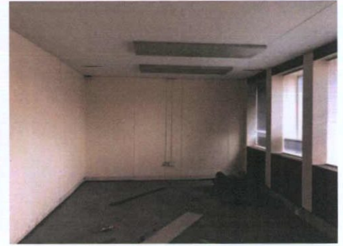
Plate 237: Room 3 — West wall
