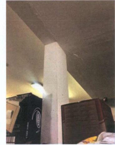
Plate 65: Centrally located concrete column within shop
