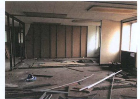
Plate 367: Rooms 8-12 — East wall
