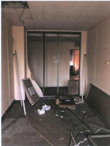
Plate 270: Room 12 — North wall
