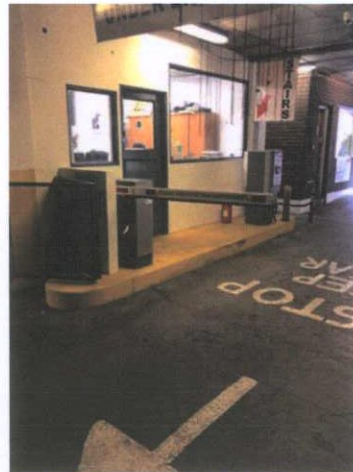
Plate 89: Car entrance barrier and office
