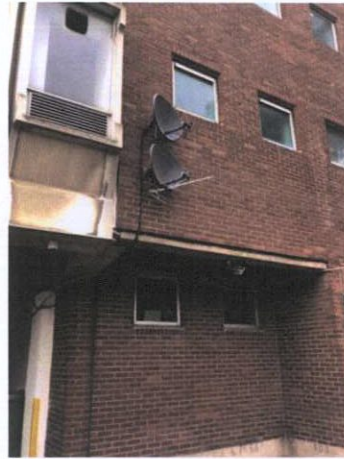
Plate 167: South west wall of west stair core
