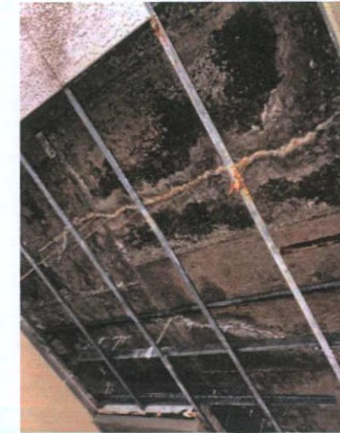
Plate 438: Room 9 — Suspended ceiling damage
