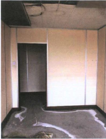
Plate 435: Room 9 — South wall
