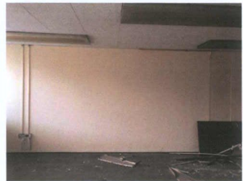
Plate 233: Room 2 — West wall
