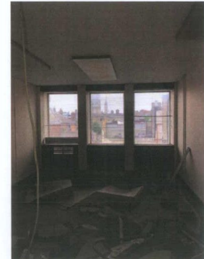
Plate 281: Room 15 — North wall
