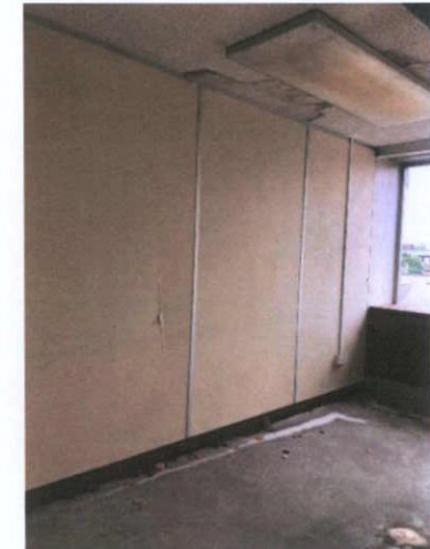
Plate 446: Room 11 — West wall
