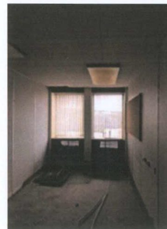
Plate 362: Room 7 — South wall
