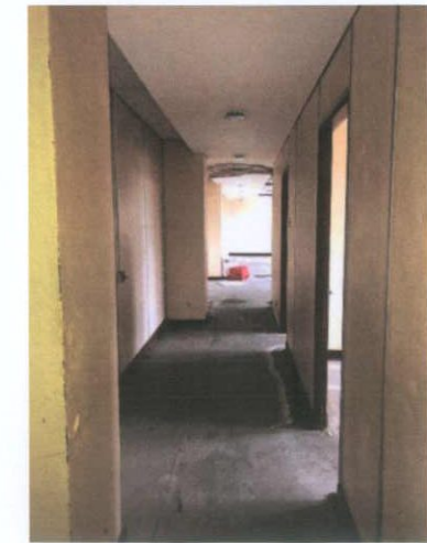
Plate 450: Secondary hallway connecting rooms 7,9,10,11
