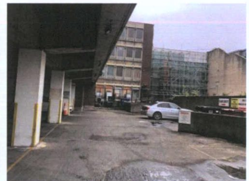
Plate 157: South boundary wall connecting to main building
