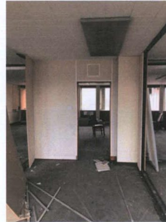
Plate 350: Room 4 — South wall
