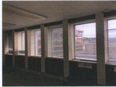
Plate 236: Room 3 — North wall
