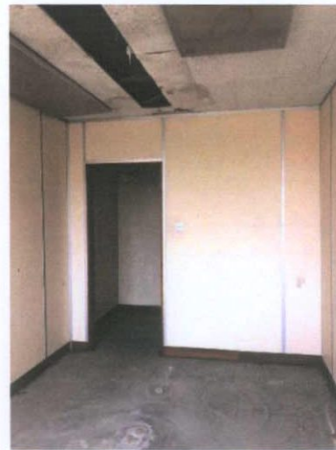
Plate 448: Room 11 — South wall
