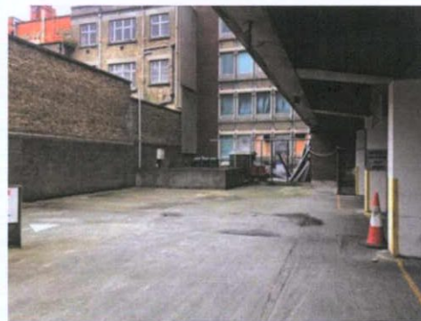
Plate 156: North boundary wall connecting to main building
