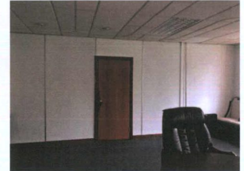
Plate 195: North wall of board room
