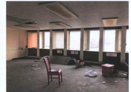
Plate 355: Room 6 — South wall
