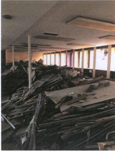
Plate 213: South section of main room used to store materials from demolition
