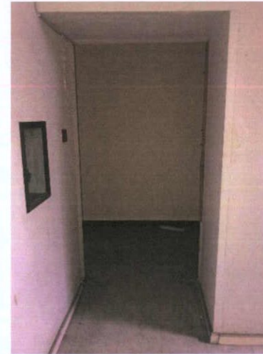
Plate 304: Entrance doorway onto level 3 from west stairwell
