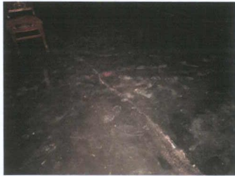
Plate 230: Concrete floor finish
