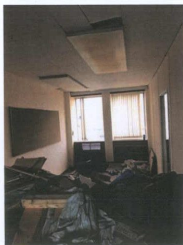
Plate 376: Room 18 — South wall
