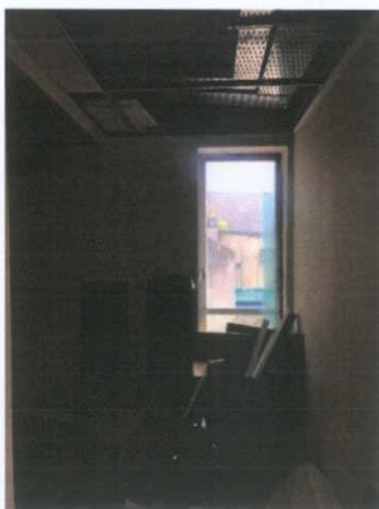
Plate 321: Corridor from lift lobby to main room
