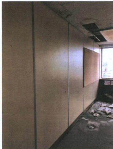
Plate 455: Room 12 — West wall
