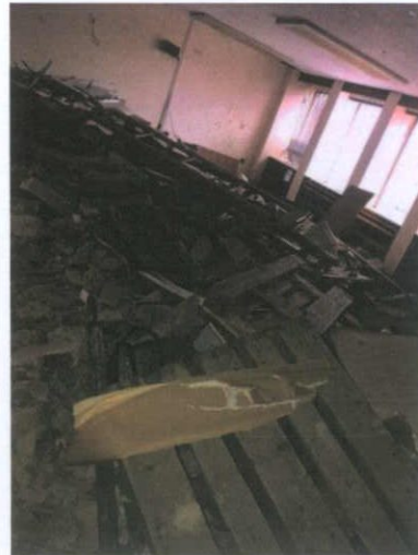
Plate 279: Room 14 — Non accessible due to demolished material
