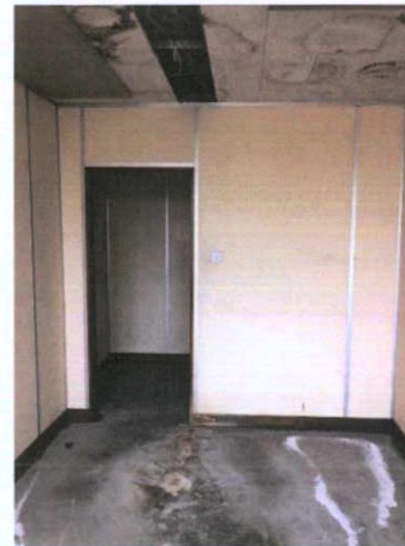
Plate 441: Room 10 — South wall
