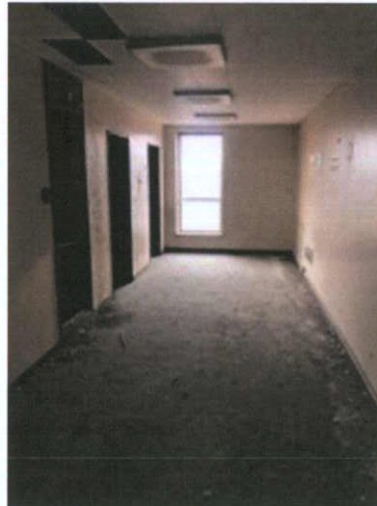
Plate 488: Lift lobby — North wall
