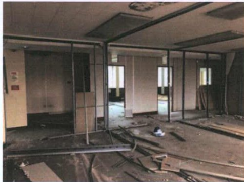
Plate 368: Rooms 8-12 — North wall
