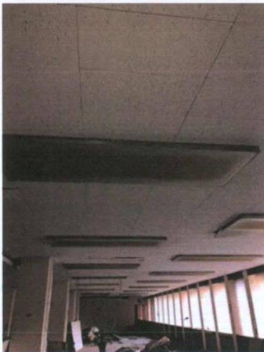
Plate 217: Typical suspended ceiling throughout floor
