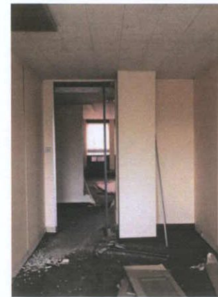
Plate 248: Room 7 — South wall
