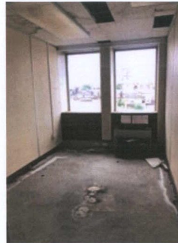
Plate 445: Room 11 — North wall
