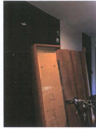
Plate 109: Storage unit in WC hallway
