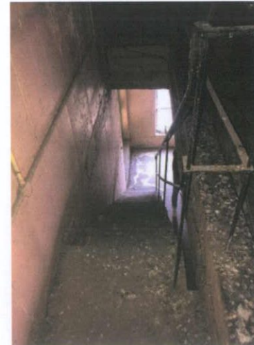
Plate 497: Stairway from level 5 to plant room
