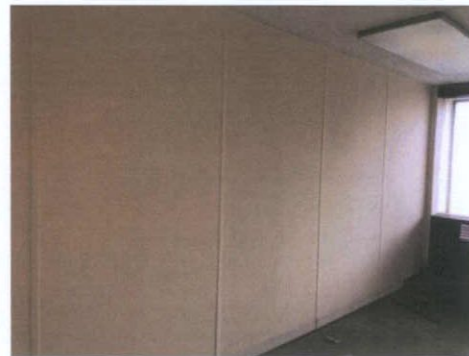
Plate 247: Room 7 — West wall
