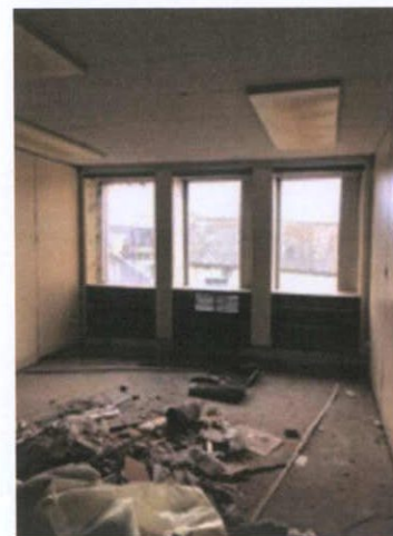
Plate 374: Room 17 — South wall
