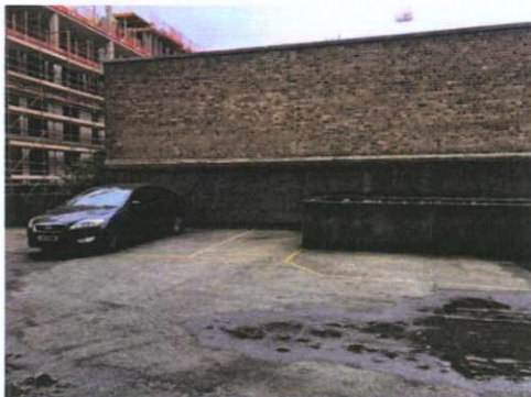
Plate 154: North boundary wall
