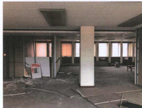
Plate 353: Room 5 — South wall
