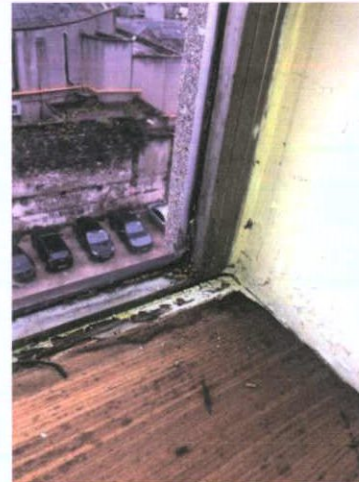
Plate 473: Room 16 — Window detail
