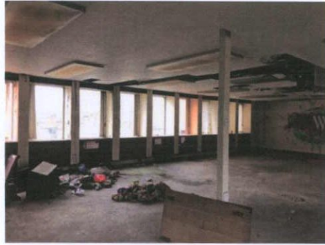
Plate 356: Room 6 — South wall
