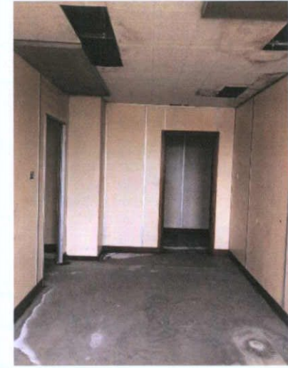
Plate 454: Room 12 — South wall
