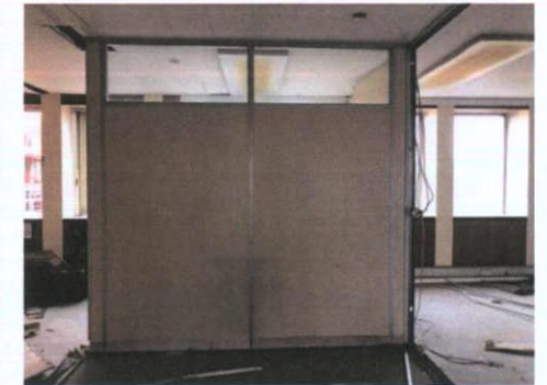
Plate 339: Room 2 — North wall
