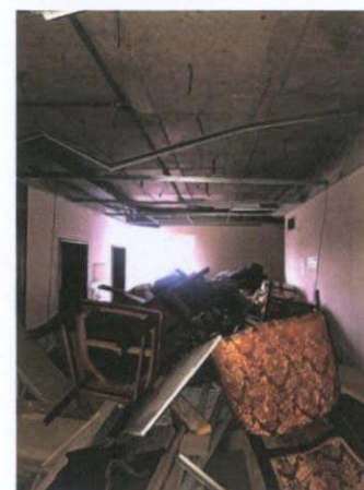
Plate 318: Lift lobby – North wall
