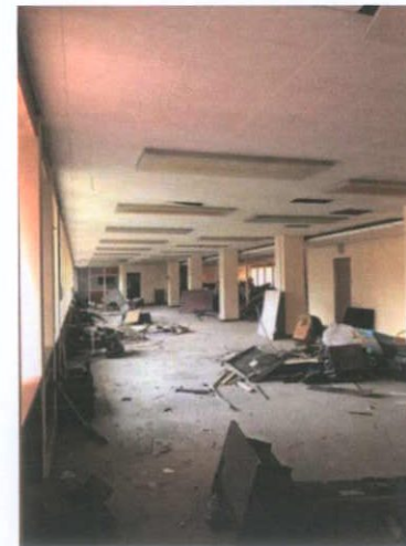
Plate 211: Level 2 main room
