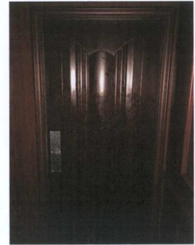
Plate 135: Entrance door to disused fire exit
