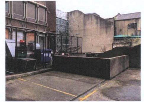
Plate 169: South east area of car park
