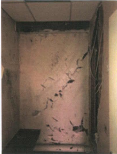
Plate 411: Room 2 — North wall
