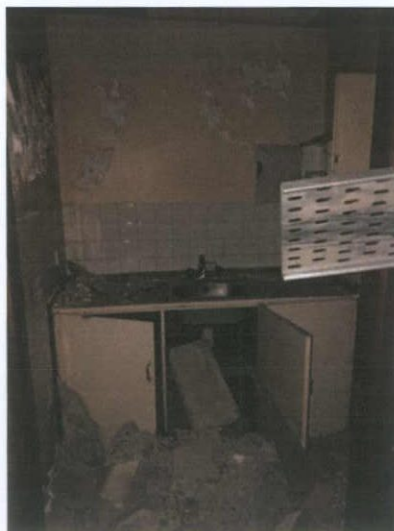
Plate 295: Doorway of kitchenette
