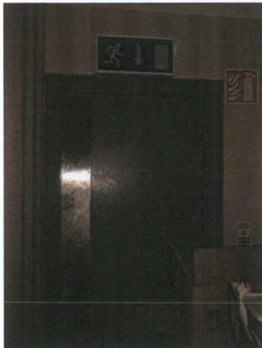
Plate 136: Fire exit door
