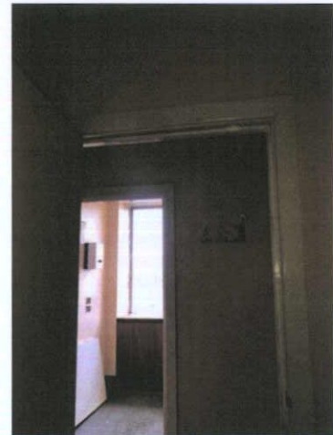
Plate 408: Room 2 — South wall
