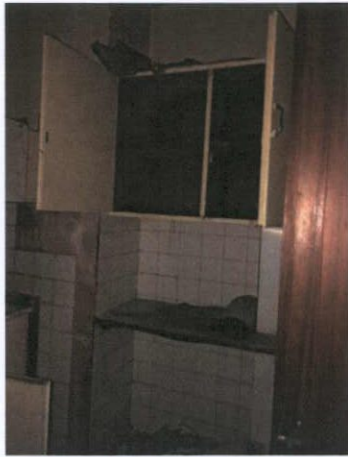
Plate 298: East wall of kitchenette
