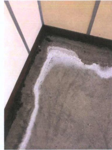
Plate 437: Room 9 — Carpet under partition
