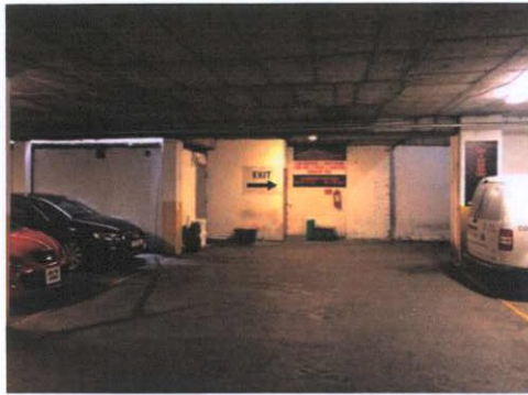
Plate 92: West wall at rear of car park
