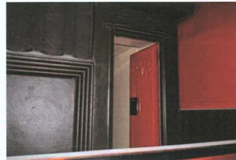
Plate 42: T-2 – Detail to doorway to south-east
