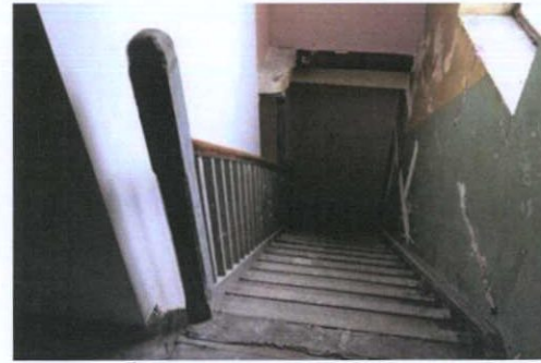
Plate 54: FO-1 – View to west from third floor landing
