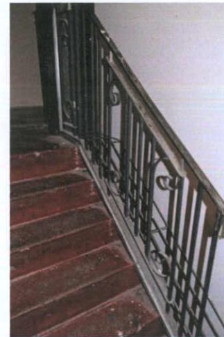
Plate 24: B-4 – View to north-east; original balustrade
