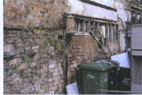
Plate 7: Red brick to north-east
