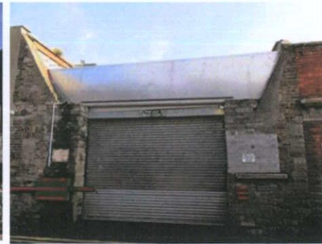
Plate 8: Rear elevation of extension onto Moore Lane
