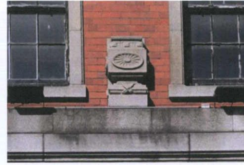
Plate 4: Limestone bracket
