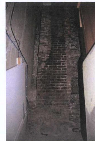
Plate 28: B-8 – View to south towards party wall
