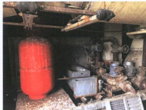
Plate 501: Plant room — North wall 1
