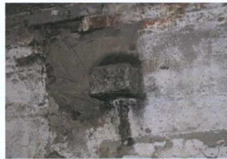
Plate 39: G-3: Granite corbel in southern wall
