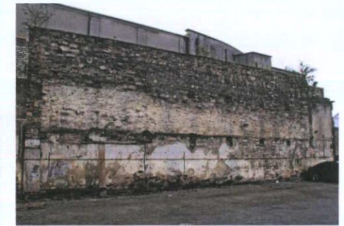
Plate 9: View to west; Calp limestone boundary wall
