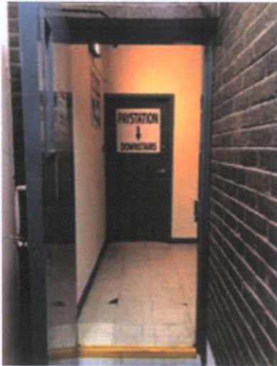
Plate 515: Access to stair at ground level
