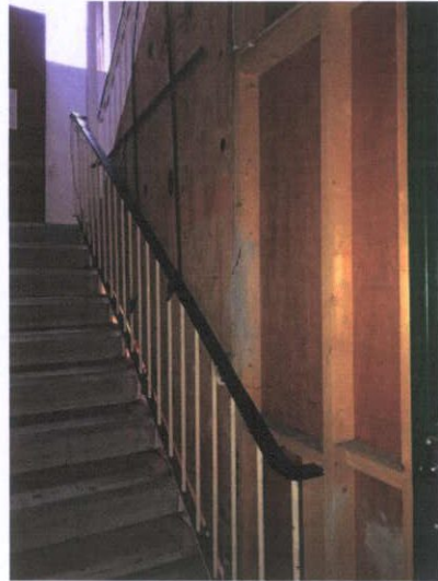
Plate 516: Stair wall to block upper levels
