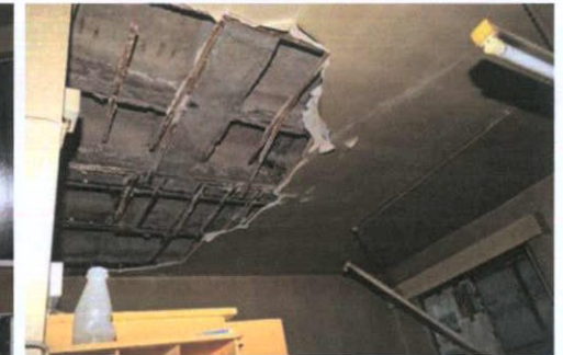
Plate 51: T-6 - View to ceiling; concrete structural substrate
