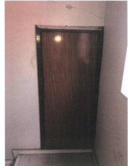
Plate 518: Access door to service riser
