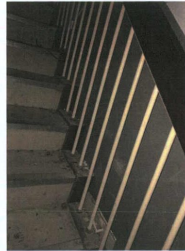
Plate 511: Stair baluster detail
