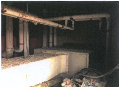
Plate 499: Plant room — South wall 1
