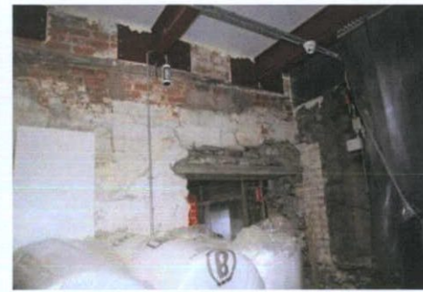
Plate 40: G-3 - Entry to rear of 44 O'Connell Street Upper
