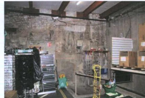
Plate 36 - G-3 - View north
