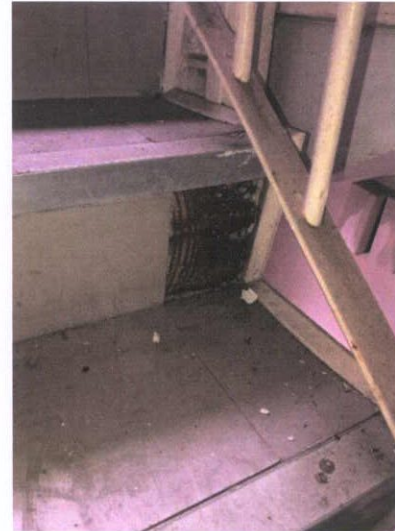
Plate 517: Typical stair tread, riser and handrail detail
