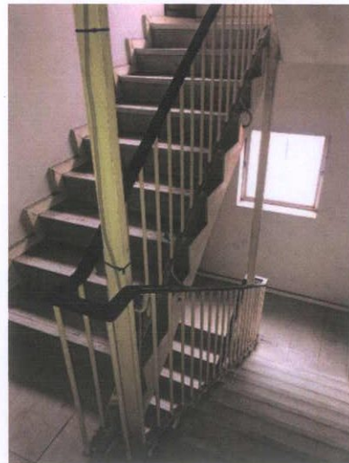
Plate 520: Typical stair flights and landings
