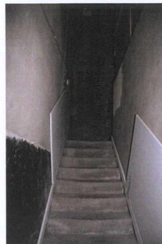
Plate 27: B-8 – View to south
