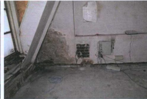
Plate 58: FO-2 – View to south
