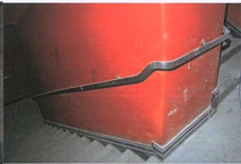
Plate 49: T-5 – Handrail on staircase
