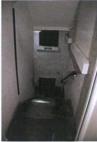
Plate 30: G-1 - View down stairway
