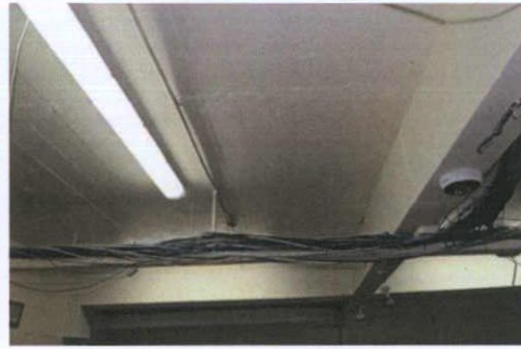
Plate 19: B-3 – Concrete structural bressummers and cast concrete floor
