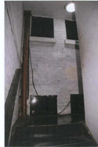
Plate 32: G-1 - Blocked windows to east of stairway
