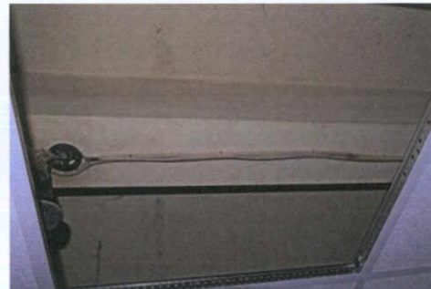
Plate 15: B-2 – Bressummers above false ceiling
