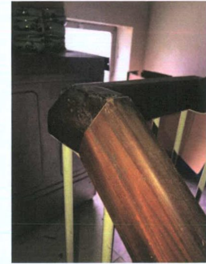
Plate 512: Stair handrail turn detail
