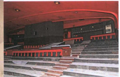
Plate 35: T-2 – View to east; former gallery / balcony; projection room to centre
