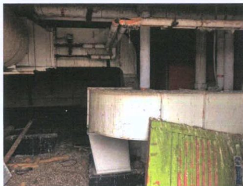
Plate 504: Plant room — East wall
