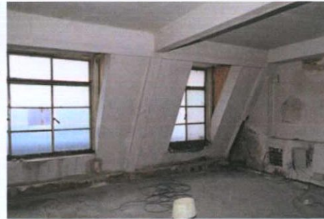
Plate 57: FO-2 – View to south-east
