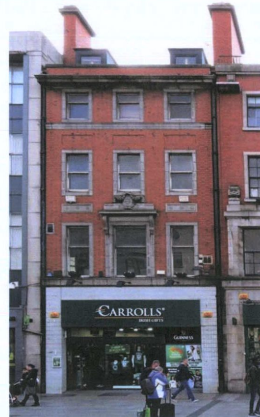
Plate 1: Front façade, 58 O'Connell Street Upper
