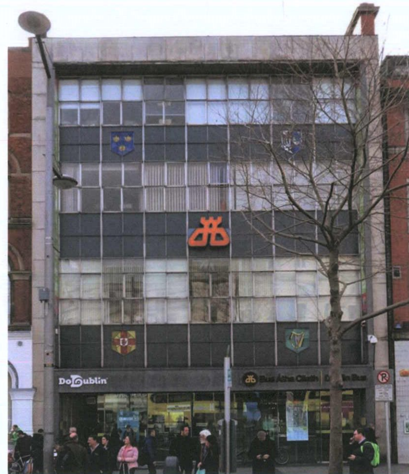
Plate 1: Front façade, 59 O'Connell Street Upper
