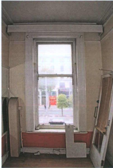
Plate 54: F-3 – View to east
