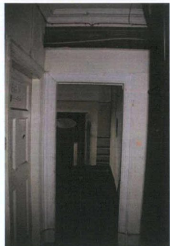
Plate 91: View into Room S-8 to north
