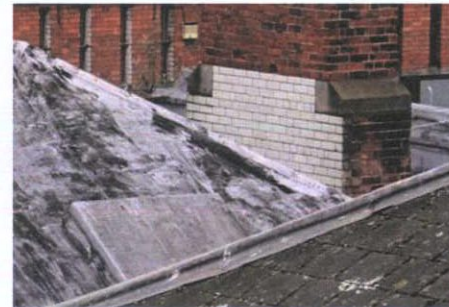
Plate 24: Glazed brick to base of chimney stack to north of Reading Room to reflect light into north-facing rooflight
