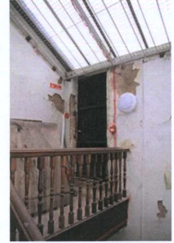
Plate 102: View to south-west
