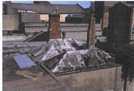
Plate 23: View to extension from south-west
