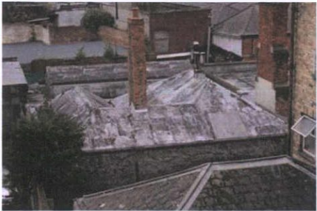
Plate 22: View to Reading Room from south-east
