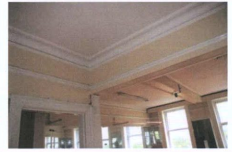
Plate 73: S-3 – View to ceiling
