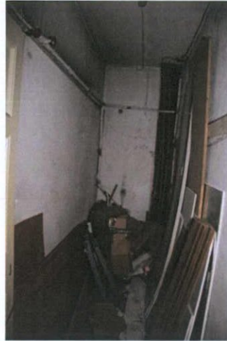
Plate 124: T-8 – View to north
