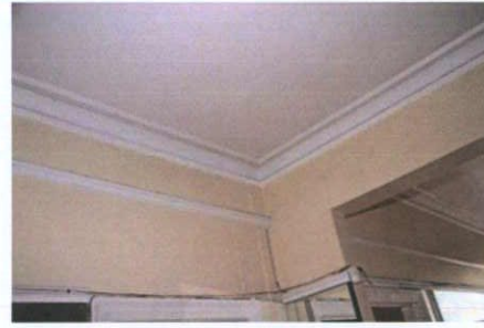
Plate 52: F-2 – View to ceiling
