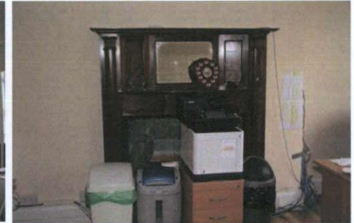
Plate 60: F-7 – Detail to chimney piece
