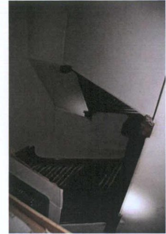
Plate 68: F-9 – Stairwell; view to upper floors
