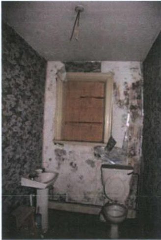
Plate 119: T-6 – View to west
