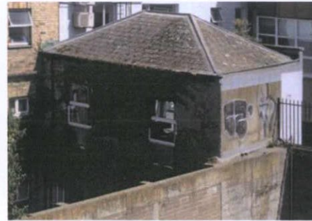
Plate 12: View of extension from south-west
