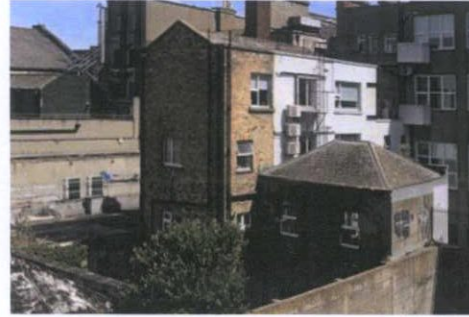
Plate 11: View of return and extension from south-west
