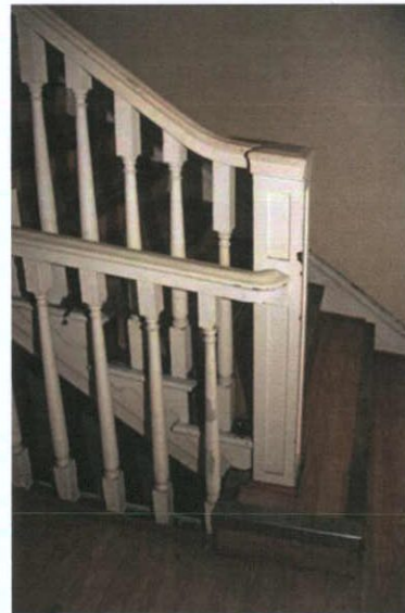
Plate 47: F-1 – Detail to balustrade
