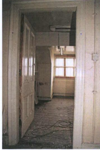
Plate 99: FO-1 – View to east into Room FO-5
