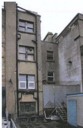
Plate 8: Rear elevation of main building
