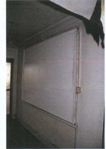
Plate 106: T-2 – Blocked-up window opening to south wall
