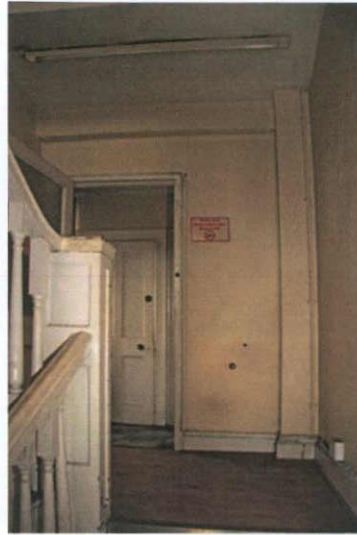
Plate 59: S-1 – View to west towards Room S-2
