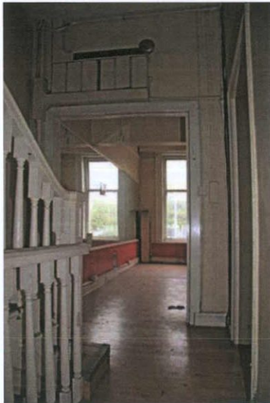
Plate 46: F-1 – View to east
