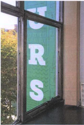
Plate 133: S-4 – View of steel window to east
