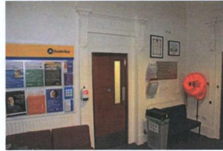
Plate 98: F-1 – View to north-east at first floor landing; entry to Room F-2
