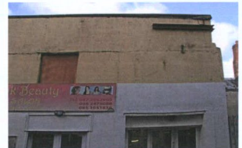
Plate 9: Former slit window, now blocked-up, noted to first floor to south elevation
