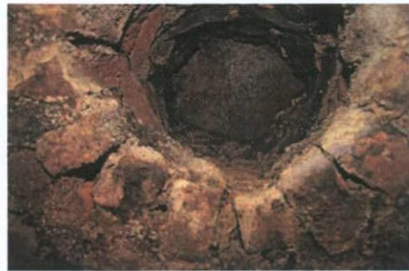
Plate 12: B-2 - Coal hole to soffit of vault
