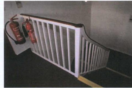
Plate 171: T-9 – Detail to balustrade
