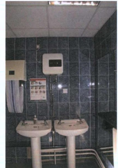
Plate 144: S-9 – View to west
