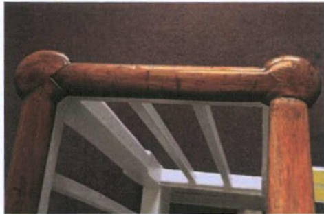
Plate 169: T-9 – Detail to balustrade
