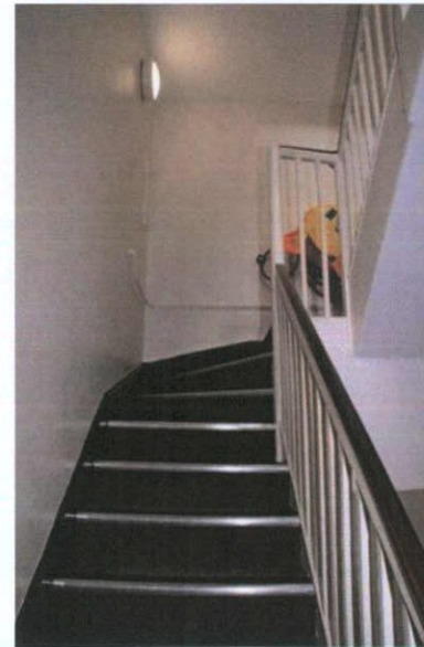
Plate 119: F-9 – View to north
