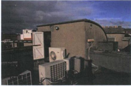
Plate 177: FO-1 – View to north-west
