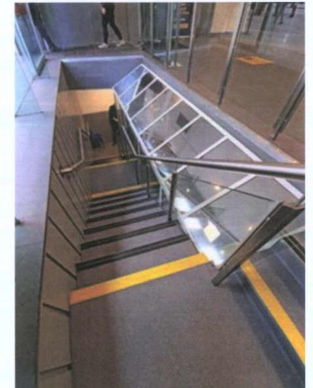
Plate 73: G-1 – View to staircase leading to basement level
