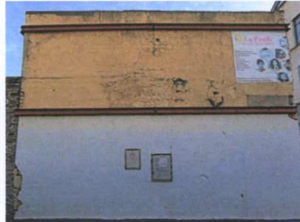
Plate 3: West elevation; former cruciform ventilation opening to high level
