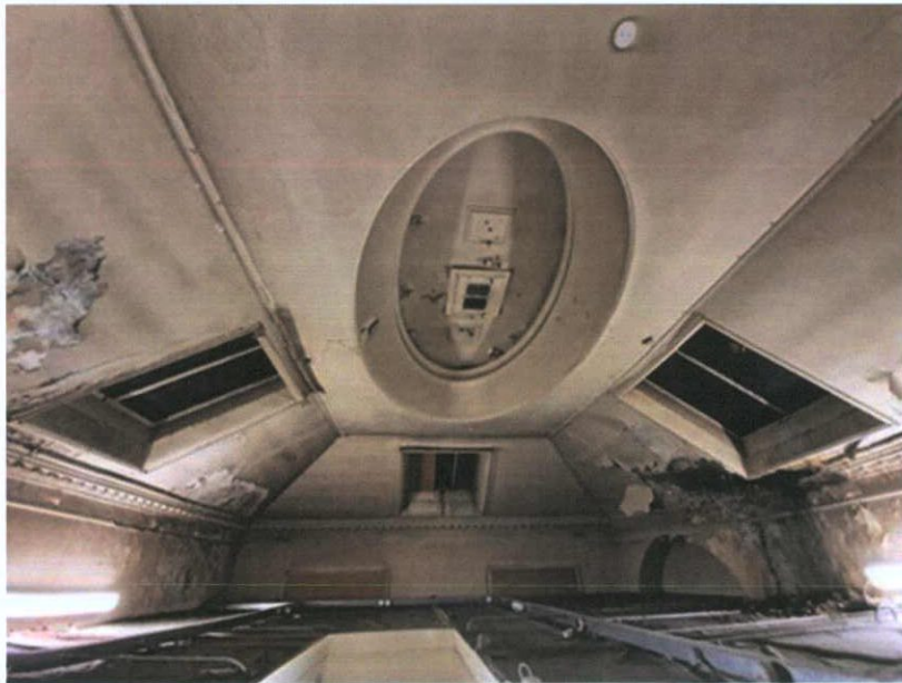
Plate 94: G-13 – Original ceiling over suspended ceiling in Reading Room
