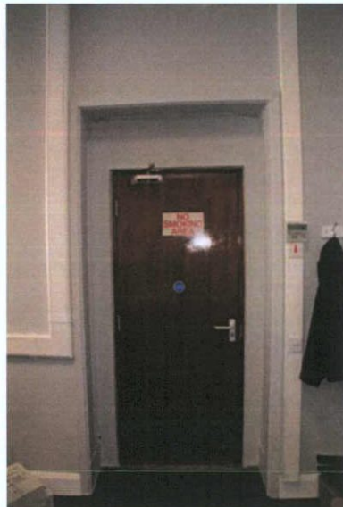
Plate 109: F-4 – View to north towards entry to Room F-1
