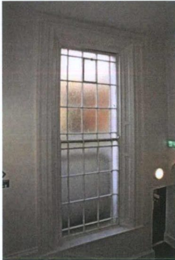
Plate 125: S-1 – View to west
