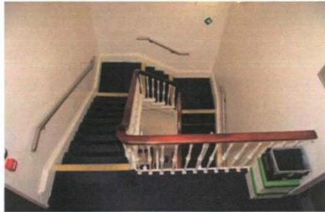
Plate 153: T-1 – View to north
