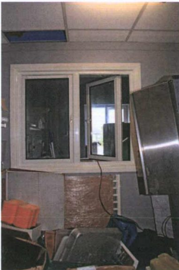
Plate 53: S-3 – View to west
