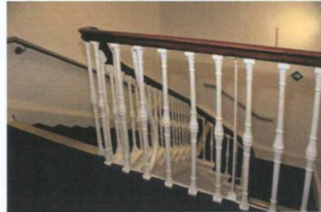
Plate 154: T-1 – Detail to balustrade at third floor landing
