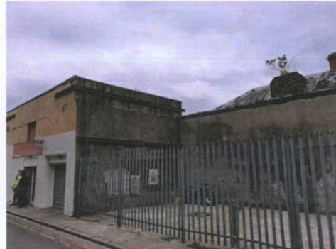
Plate 27: Site of 61a O'Connell Street Upper
