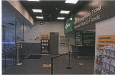
Plate 66: G-1 – View to south
