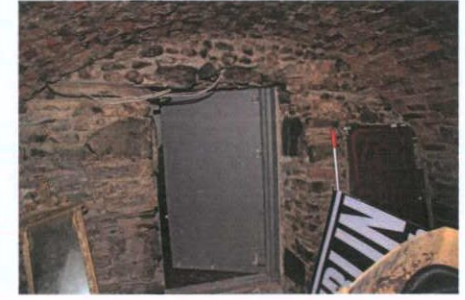
Plate 15: B-3 - View to west
