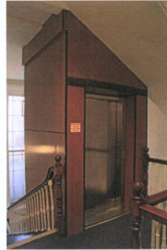
Plate 123: S-1 – View to lift shaft within open-well staircase
