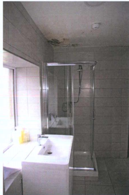
Plate 81: T-4 – View to north
