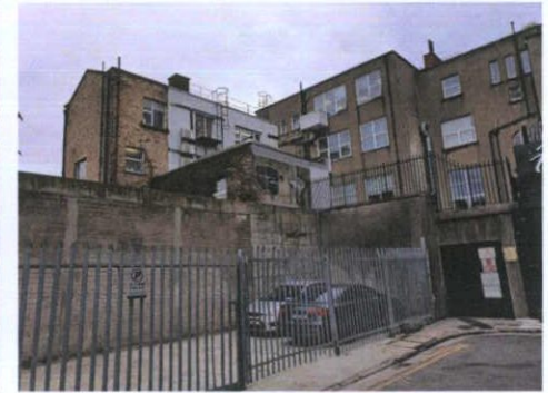
Plate 29: Site of 62a O'Connell Street Upper
