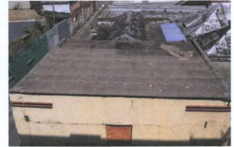
Plate 5: Flat roof as viewed from south
