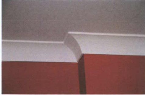
Plate 76: T-2 – Detail to coving to chimney breast
