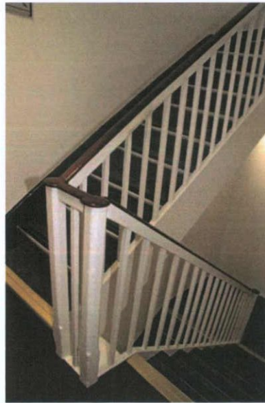
Plate 118: F-9 – View to north-west
