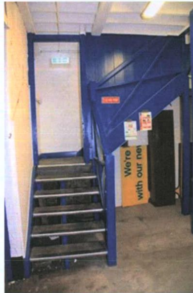
Plate 63: B-16 – View to west
