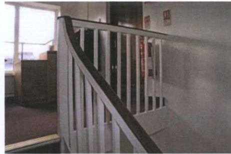
Plate 170: T-9 – View to south-west
