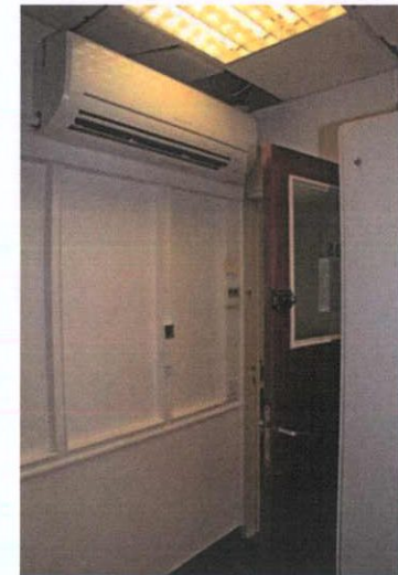
Plate 136: S-6 – View to north-west
