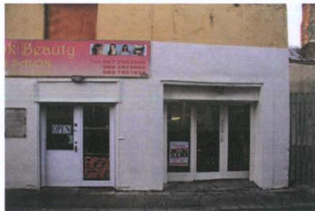
Plate 6: Possible former carriage opening to east (right)
