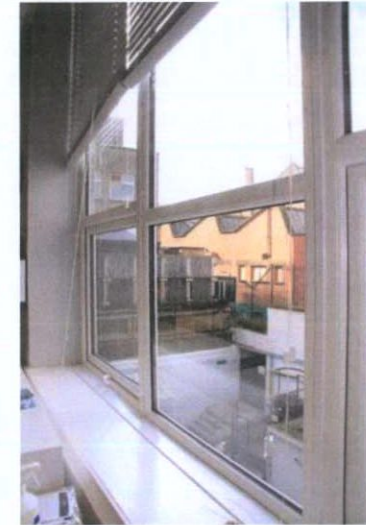
Plate 108: F-4 – View to south-west
