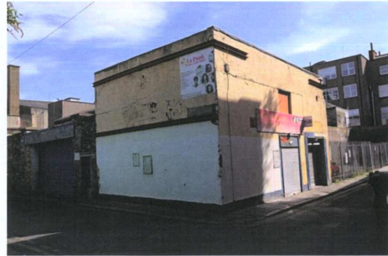
Plate 1: Exterior of 60A O'Connell Street Upper
