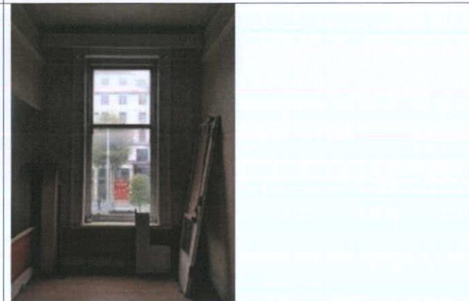
Fig. 52 Timber sash windows with moulded architraves internally and without shutters.
