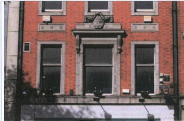
Fig. 47 Decorative plaque with swags over corniced hood moulding set to central, first floor window.
