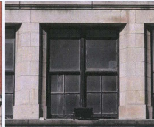
Fig. 41 One-over-four paired timber windows at first floor.
