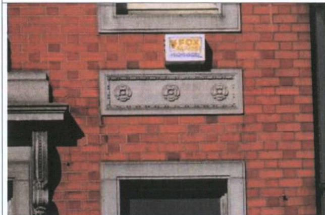
Fig. 50 Panelled granite window aprons to second floor, with decorative rosettes.
