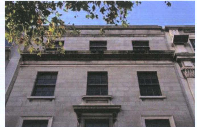
Fig. 28 Coursed, ashlar granite parapet to be cleaned and repointed as required.
