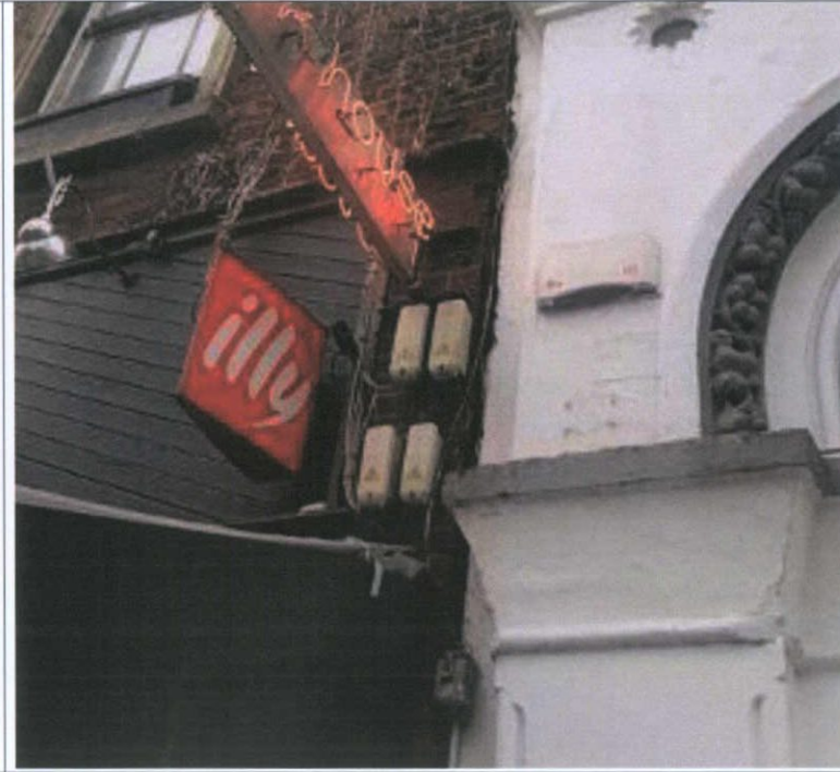
Fig. 62 Detail of contemporary brick positioned in front of the fascia and shopfront. Underlying fabric to be inspected for surviving historic fabric. It is clear from examination of historic photographs that the early 20 th century shopfront has either been significantly altered or previously altered.
