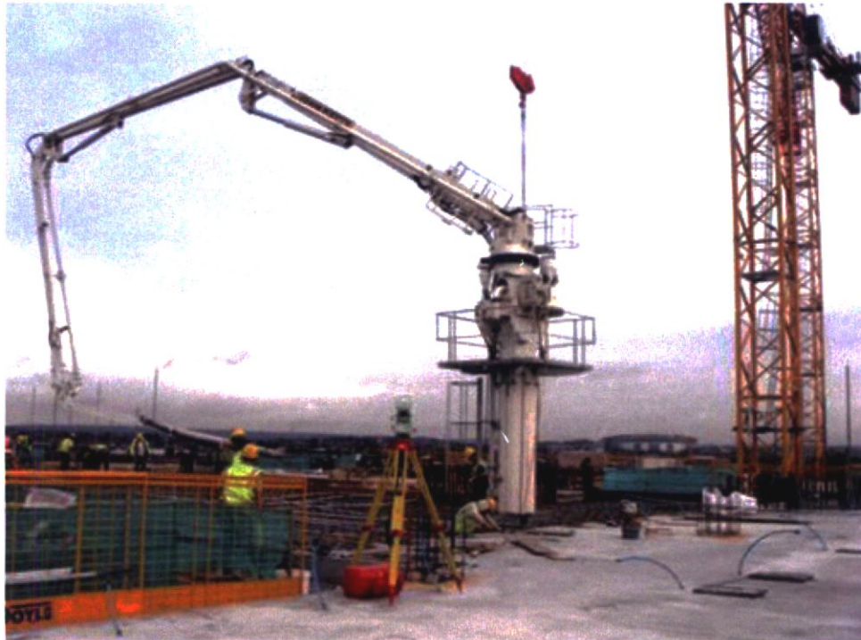
Figure 21 - Typical Concrete Placement
