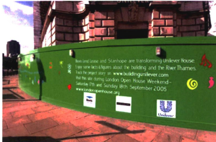
Figure 28. Typical Pavement Hoarding with Street Lighting
