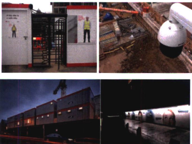
Figure 32. Typical Site Security Measures
