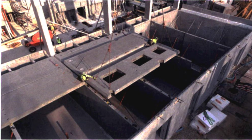
Figure 24. Typical Precast Concrete Construction
