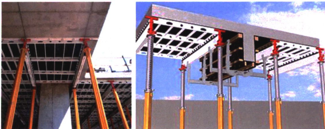
Figure 20 - Typical RC Formwork (Skydeck)
