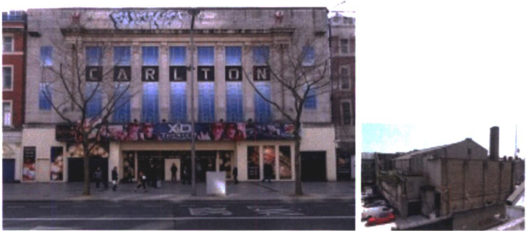
Plate 15.3.6 Front elevation of No.52-54 O'Connell Street Upper, the former Carlton Cinema and rear (upper) elevation on Moore Lane
