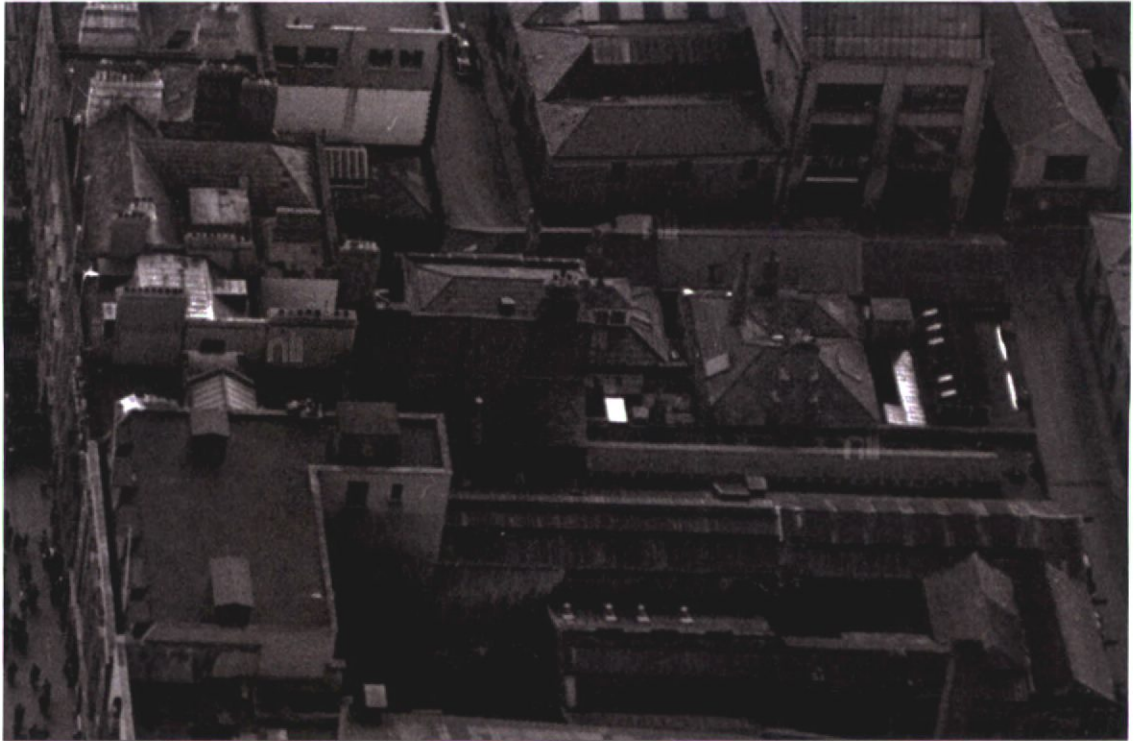
Figure 15.3.8: An aerial photograph of Site 2AB (in part), 1955 provides an interesting overview of the complex at the rear of No.59. The roof of reading room and the 'regency annex' is visible, with a lantern-roofed structure (since demolished) in the interstitial space. Source 'The Morgan Collection', National Library of Ireland.
