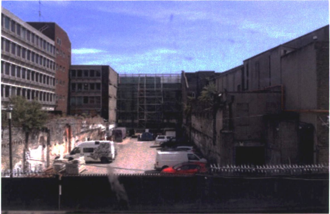
Plate 15.3.5 Overview of vacant plot at Nos.50-51 O'Connell Street Upper due east from Moore Lane
