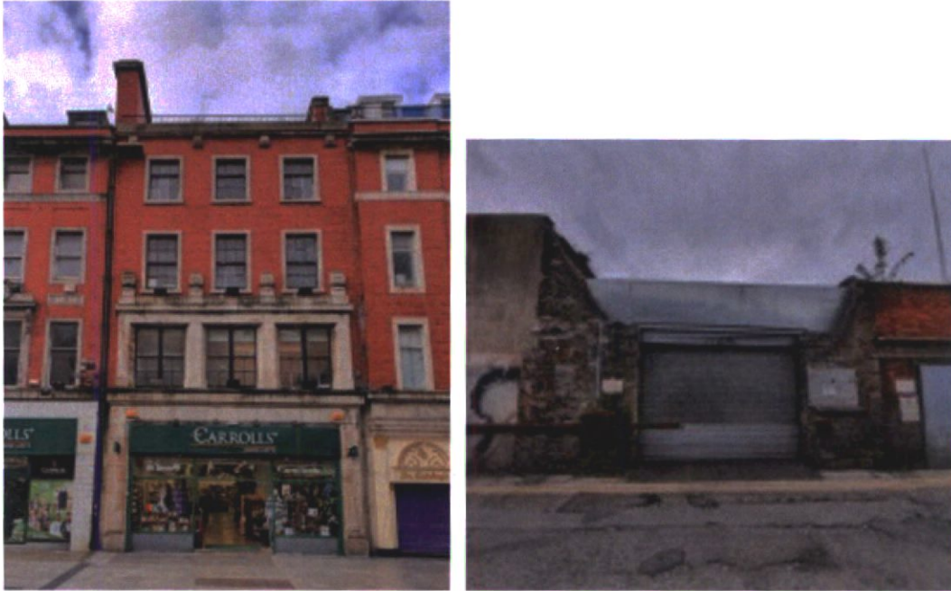
Plate 15.3.8 Front of No.57 O'Connell Street Upper and rear elevation to Moore Lane
