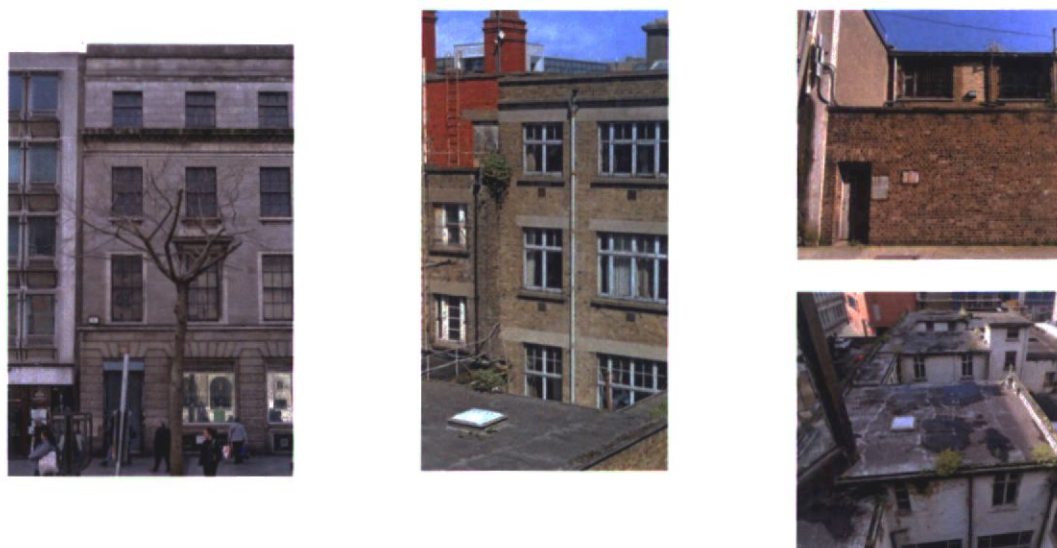
Plate 15.3.3 Front and rear elevations of No.45 O'Connell Street Upper together with Moore Lane elevation and a cameo of the rear building's roof composition
