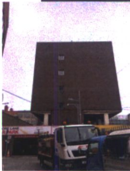
Plate 15.3.4 Front of No.46-49 O'Connell Street Upper and rear elevation on Moore Lane
