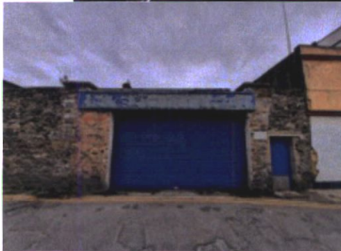
Plate 15.3.11 Interior and exterior of the car port
