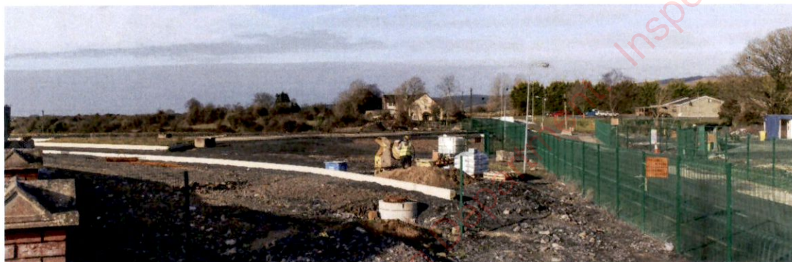
Figure 16.4 View from Old Cratloe Road at Shannonvale to the west. Subject lands are visible in the background beyond the road construction works
