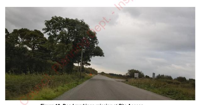
Figure 16: Road markings missing at Site Access
