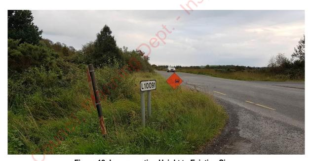
Figure 18: Low mounting Height to Existing Signs
