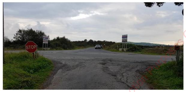
Figure 10: Poor carriageway condition on minor road opposite site
