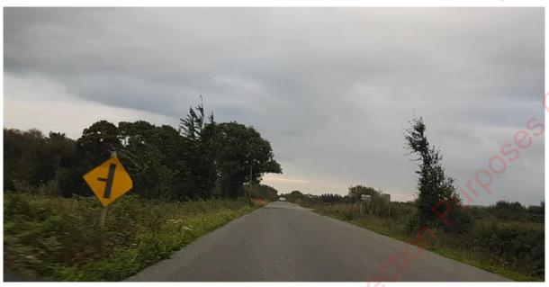
Figure 17: Low mounting Height and Limited Offset to Existing Signs
