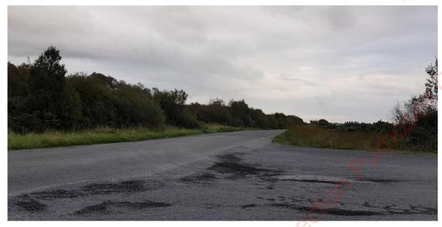
Figure 12: Poor carriageway condition and loose debris at Site Access
