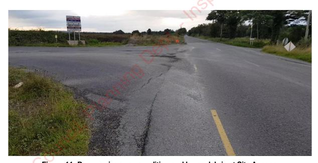
Figure 11: Poor carriageway condition and loose debris at Site Access
