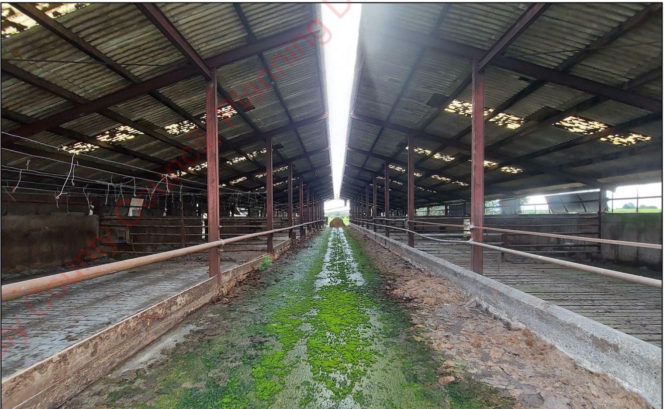
Figure 15-10: Portal frame shed with concrete slatted floor, underground slurry storage tanks
