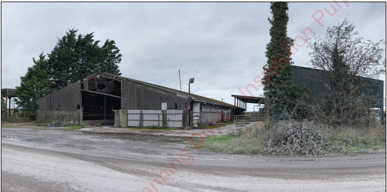
Figure 15-8: View of the site from the private access road to its south
