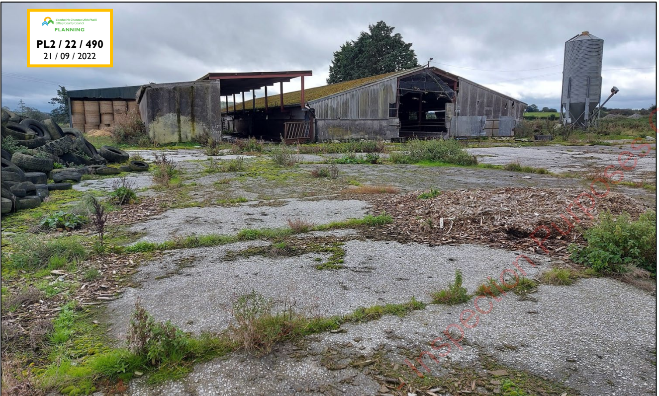
Figure 15-9: Large concrete yard to the rear of the sheds
