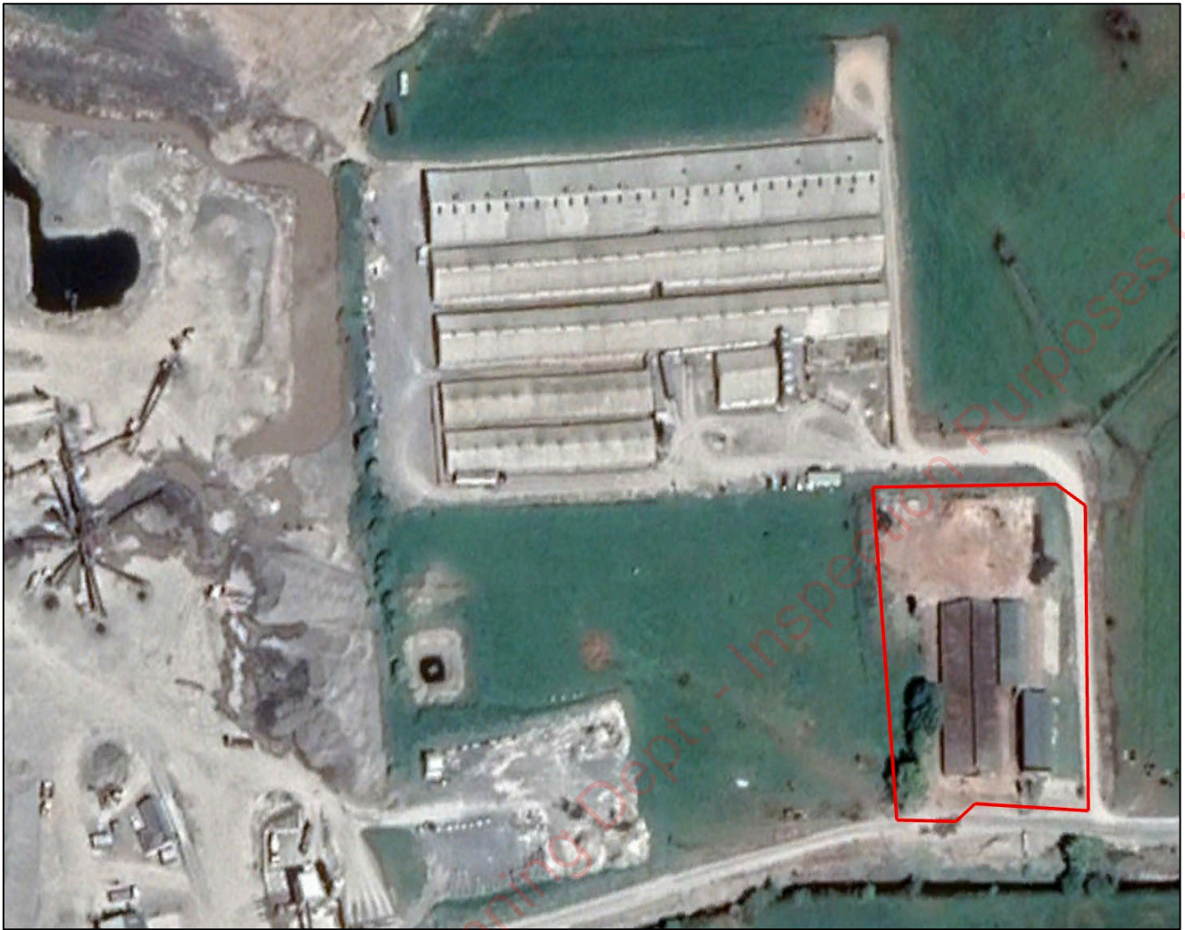
Figure 15-5: Aerial view of site, adjoined by a sand & gravel pit and Derryarkin Pig Farm
