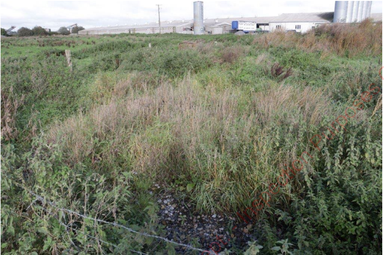
Plate 10-1: Overgrown Open Stone Soakaway Pit
