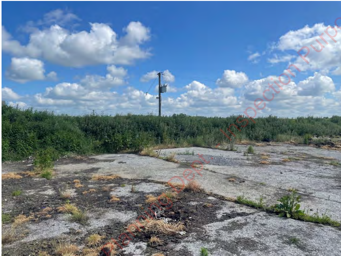
Plate 8-4: Earth Bank (BL2). Northern earth bank.
