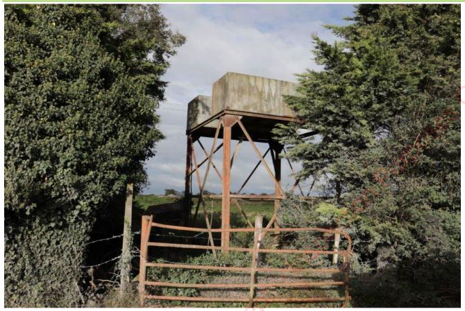
Plate 4-14: Above Ground Raised Water Storage Tank
