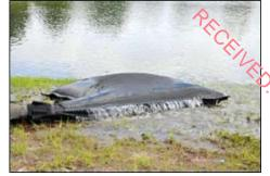
Plate 2-1 Silt Bag under inspection
