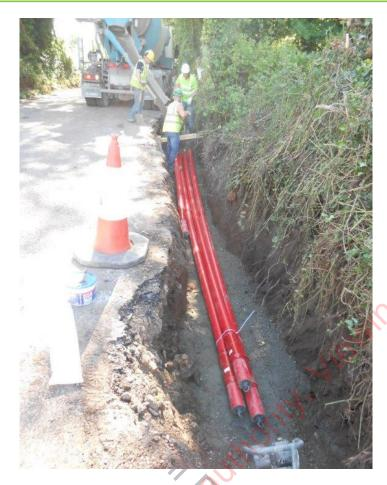
Plate 3-4: Cable Duct Laying in Trefoil Configuration
