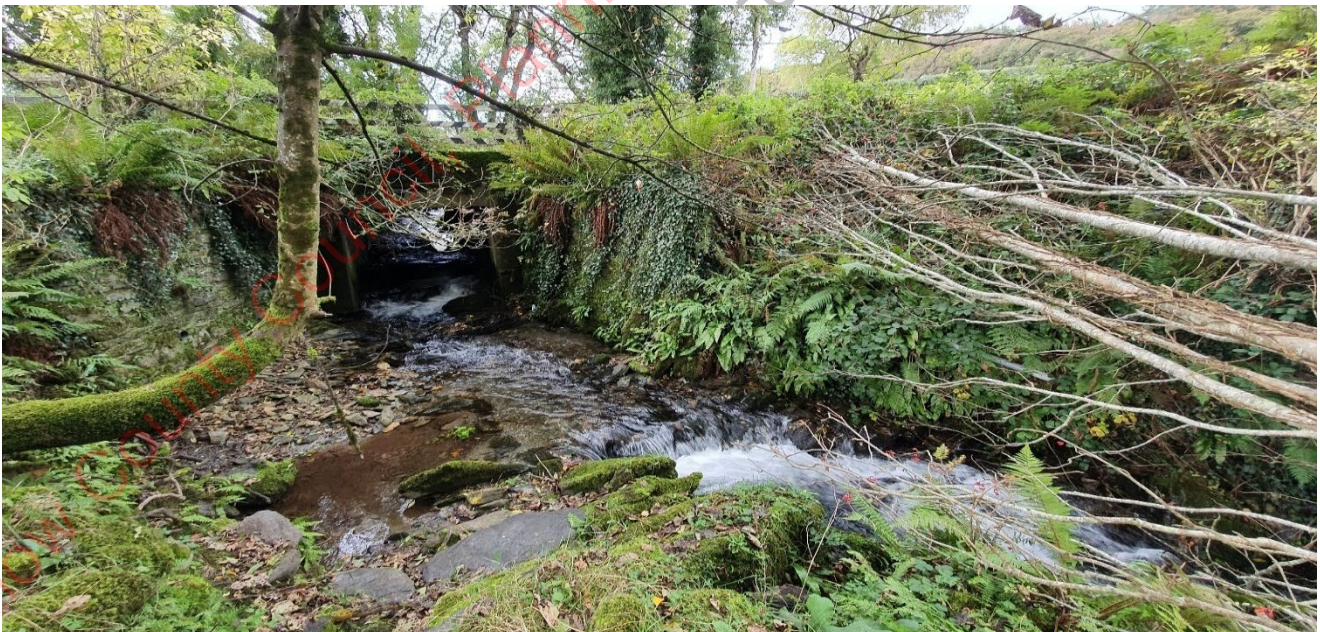
Plate 8-39: Turbine delivery work location no. 43 – Temporary Bridge Crossing Location
