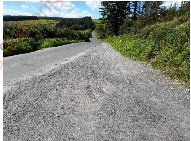
Plate 13-3: Existing Visibility to Right from Proposed Site Entrance at X=3m
