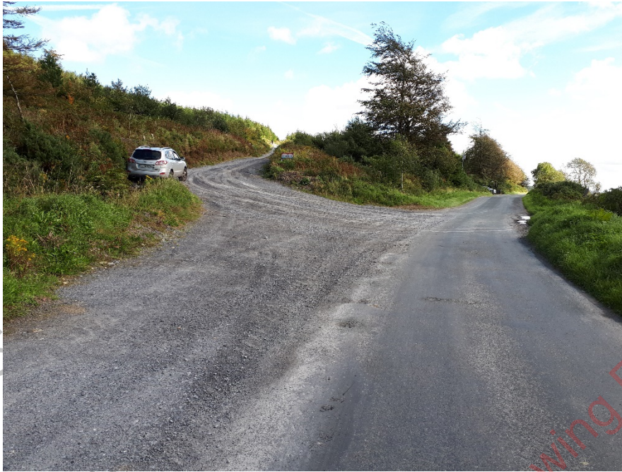
Plate 13-1: Existing Forestry Access and Proposed Site Entrance
