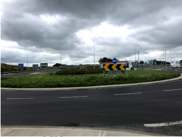
Plate 8-32: Turbine delivery work location no. 18. N80 roundabout
