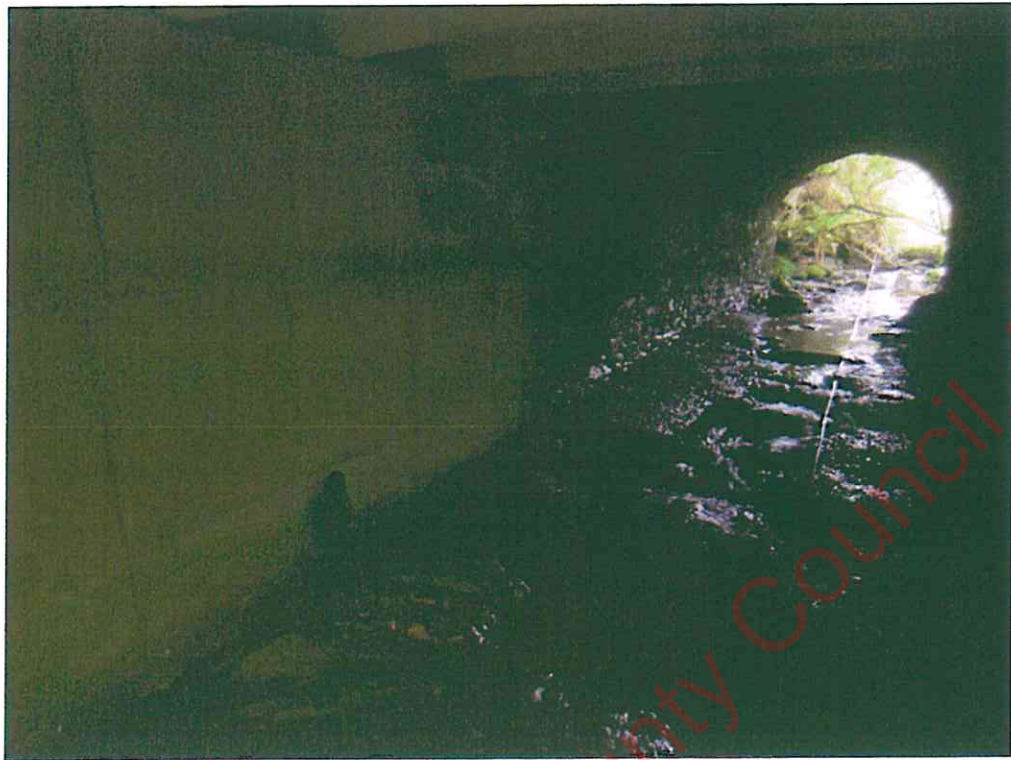
Precast Ribs and Concrete abutment downstream, Stone Arch Upstream half
