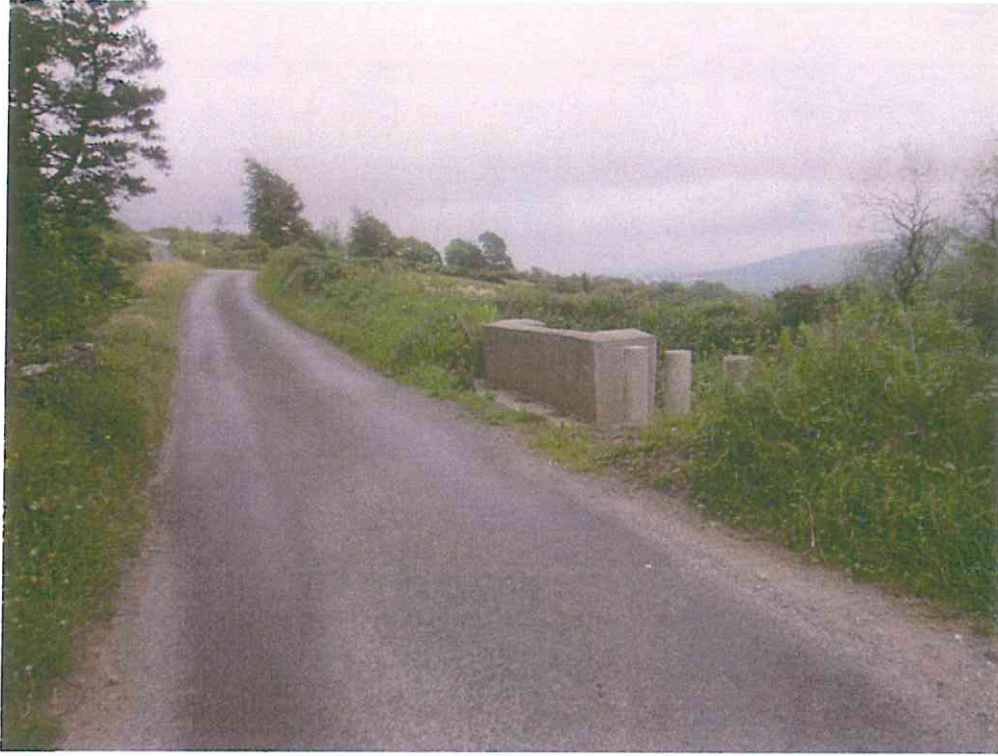
Road Surface and Parapet Wall with 215 wide block
