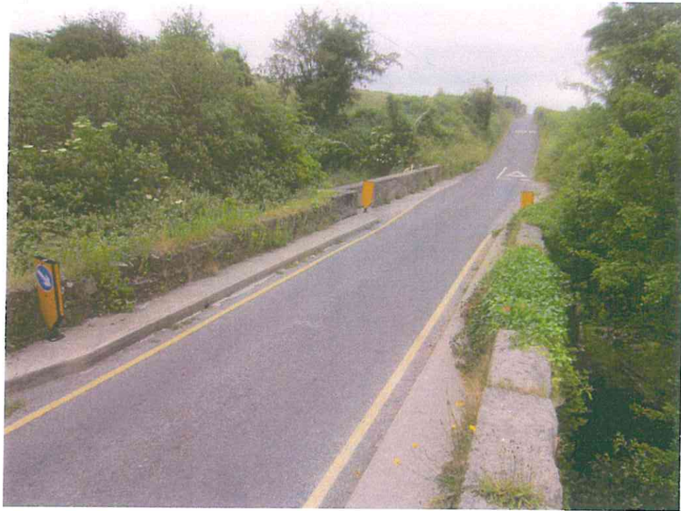
Parapet Walls Road Width 3.4m
