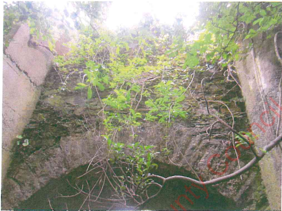
Concrete Buttresses Upstream Side
