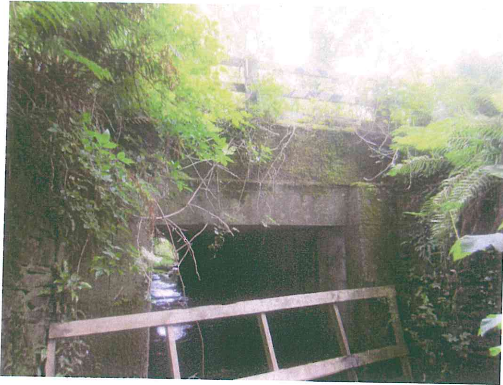
Downstream View – Outside rib and concrete Buttress
