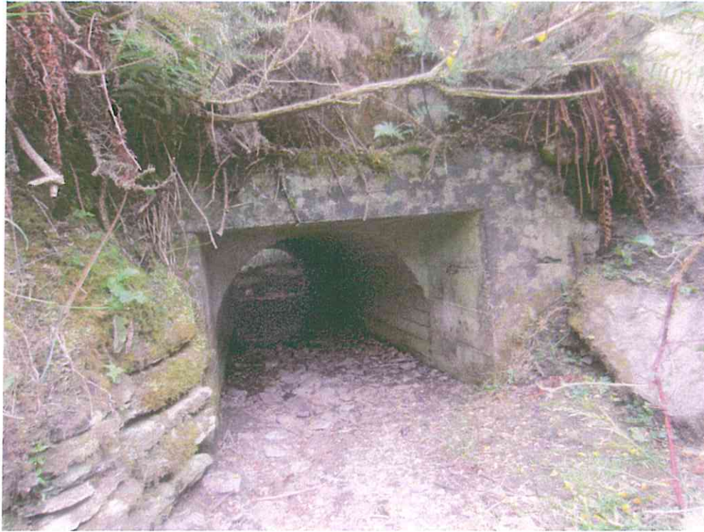
Upstream View of dry Culvert
