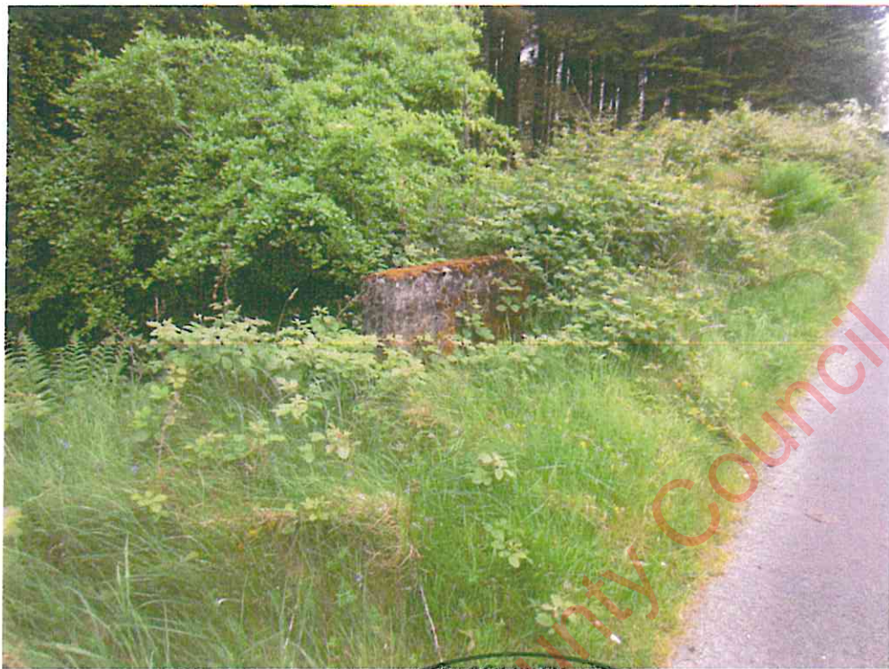
Parapet wall downstream side
