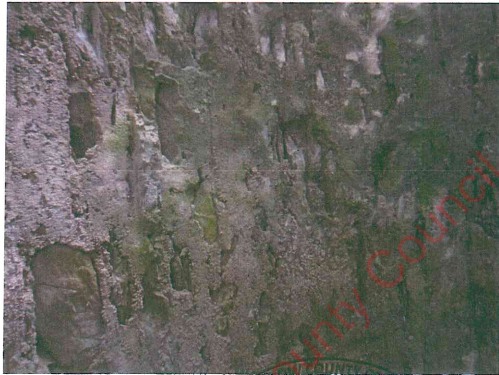
Underside of Arch
