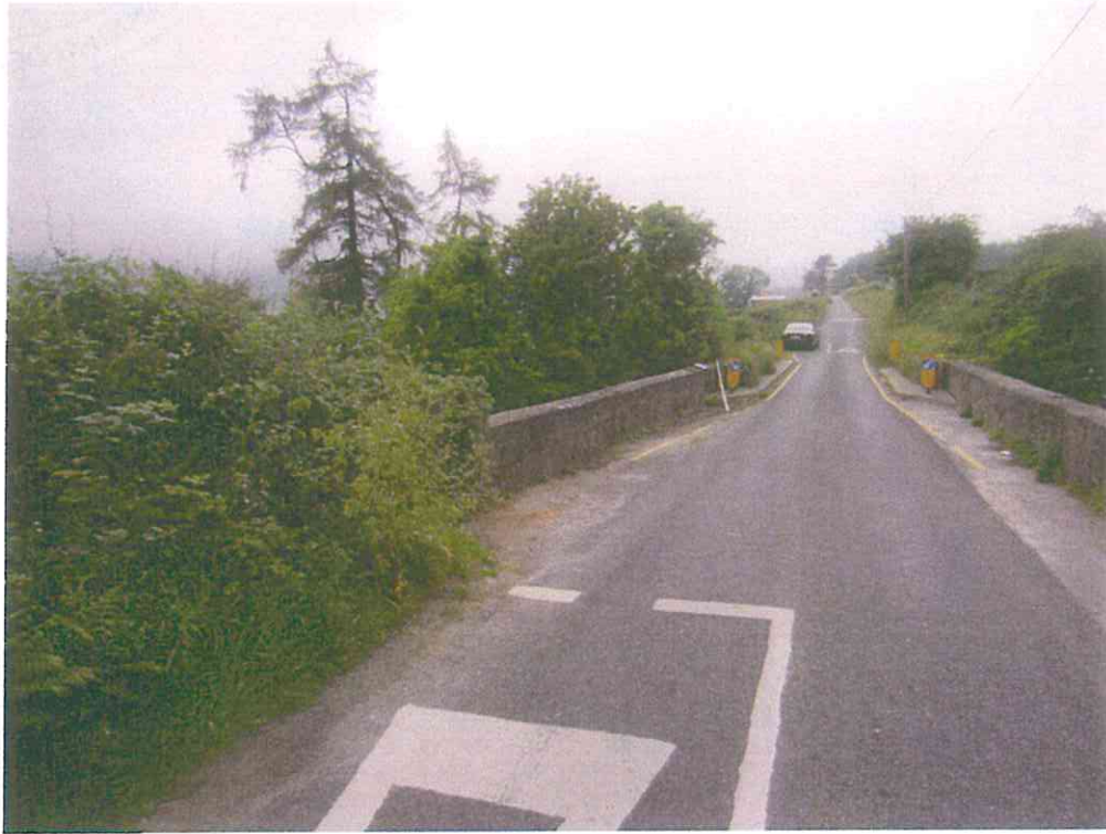
Concrete Wing Walls and Road Surface
