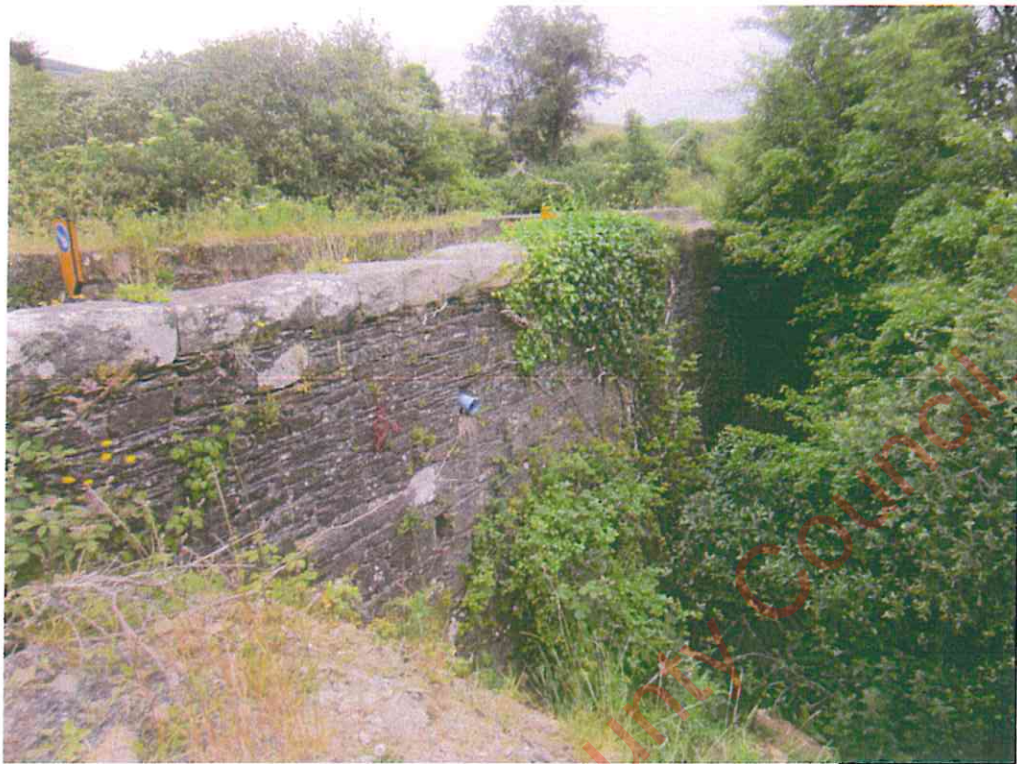
Stone Wing Wall on Bridge
