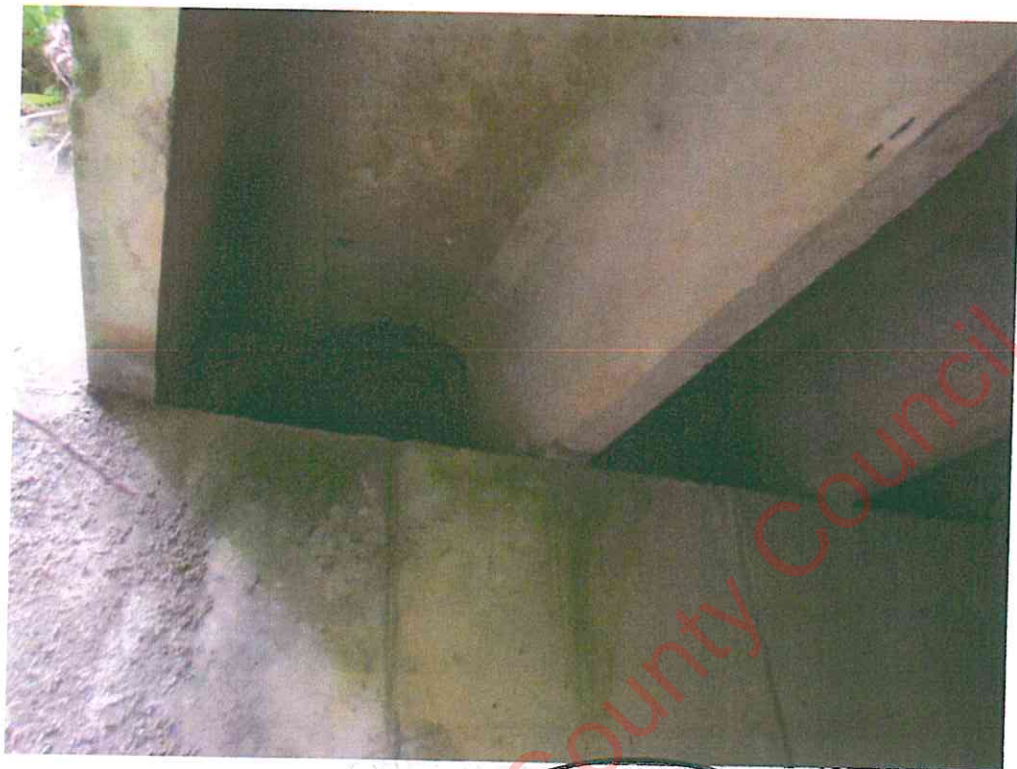
Pre Cast Concrete Ribs on downstream span
