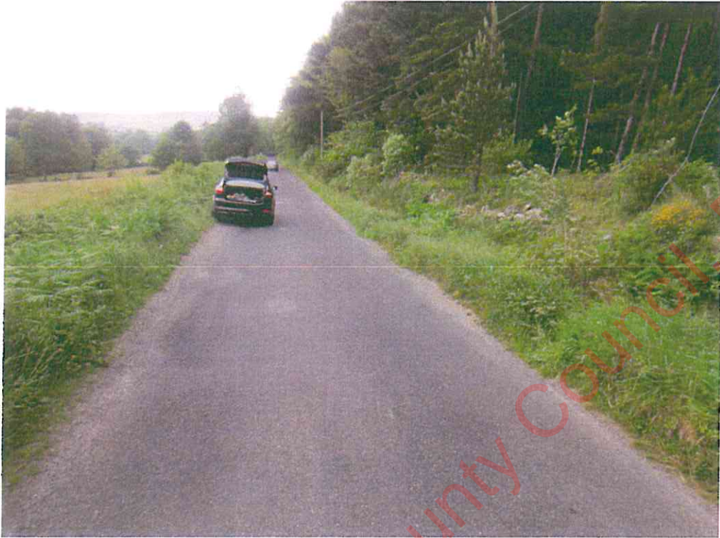
Road Surface at Slieve Stone Culvert
