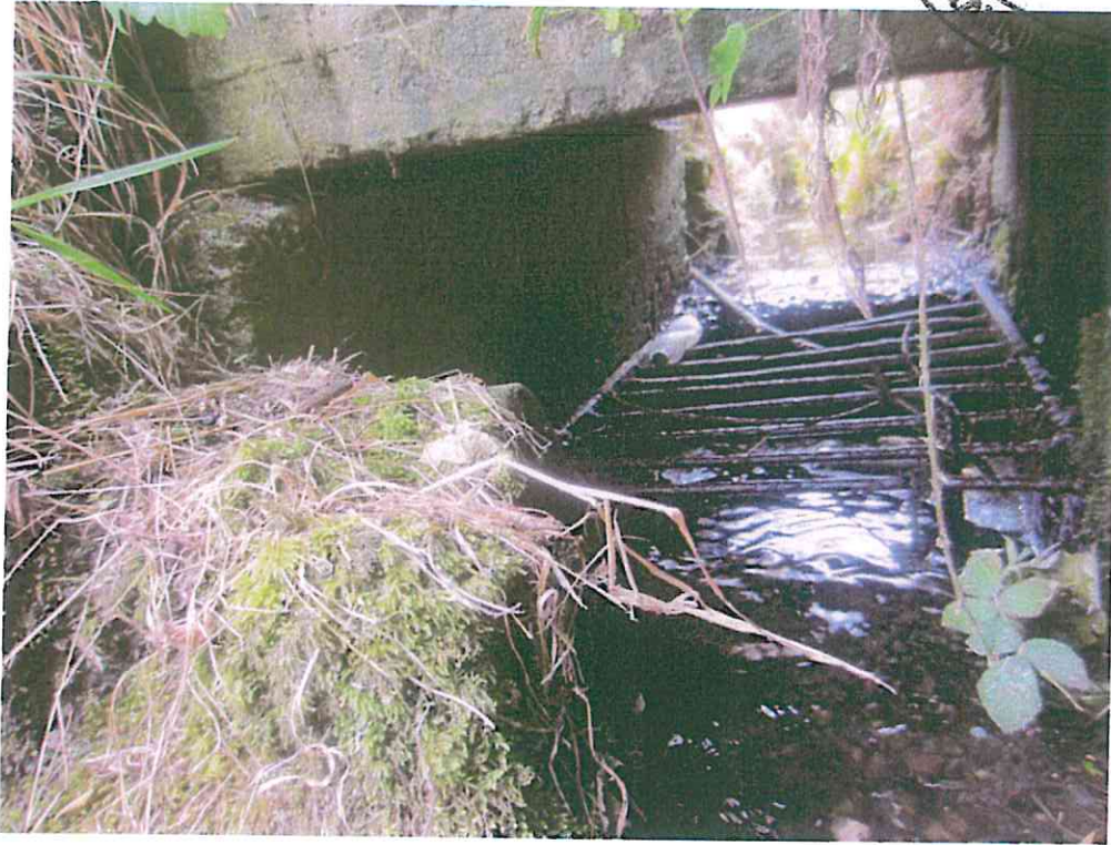
Culvert road crossing at Car on next photo
