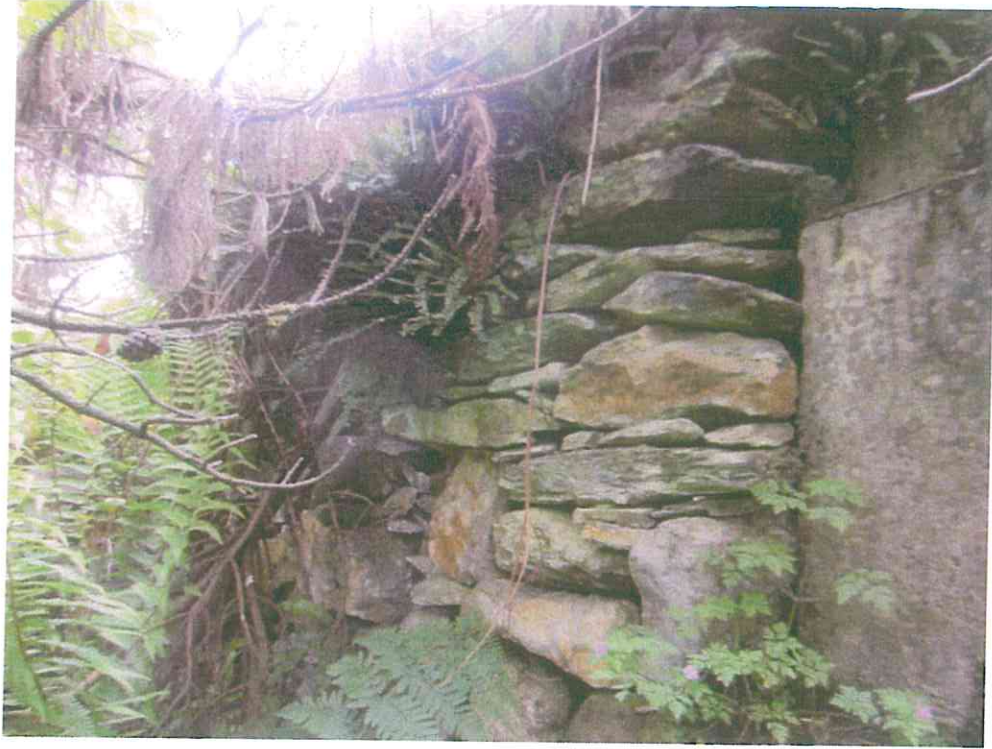
Loose stone wing wall upstream side
