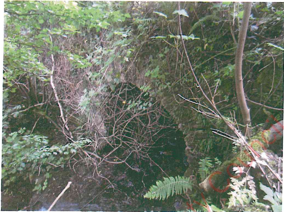
Upstream View of Stone Arch
