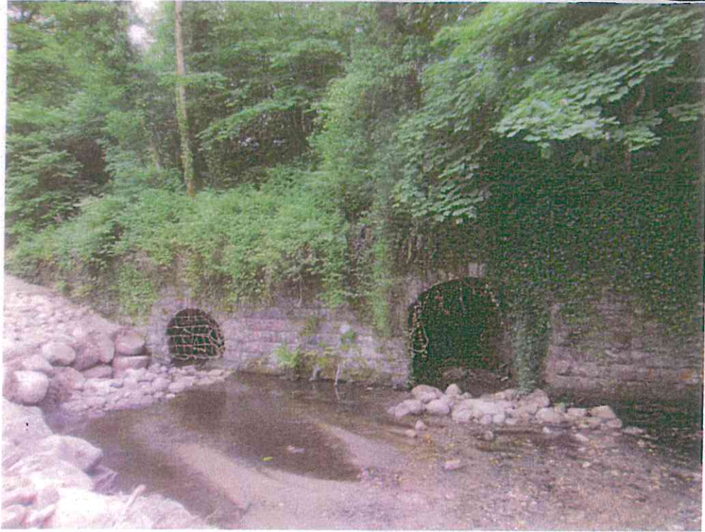
Upstream View of Arches
