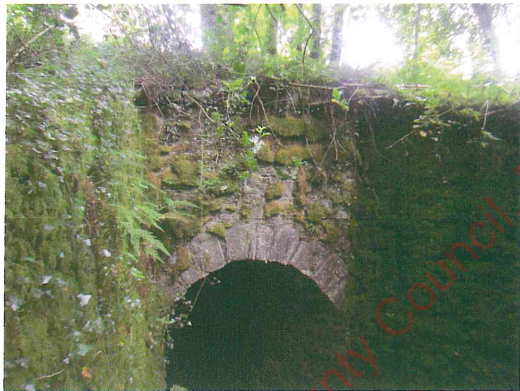
Small Arch Downstream Side
