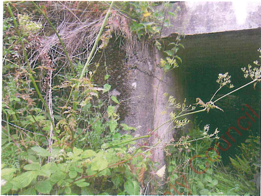
Concrete abutment downstream side
