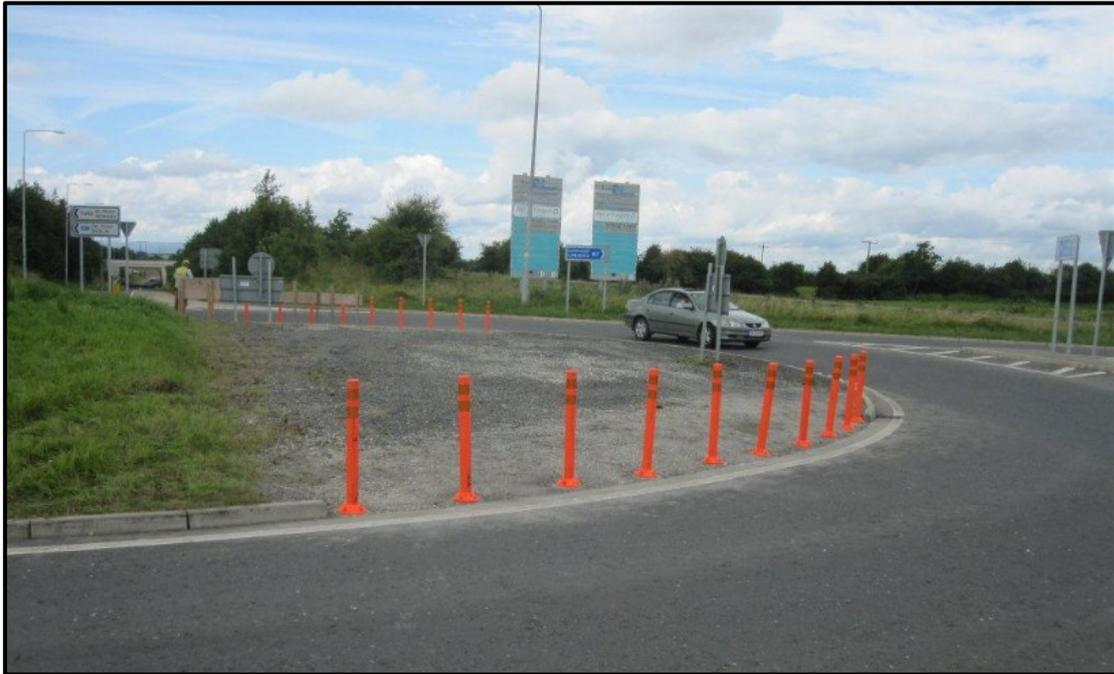
Figure 16: Example of a temporary stone road on central island of roundabout
