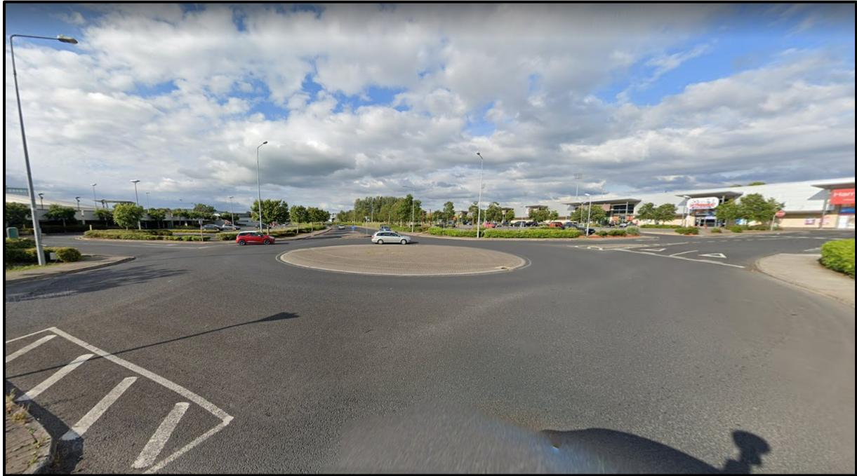
Figure 45: Example of flat central island at nearby roundabout serving the Jetland Shopping Centre
