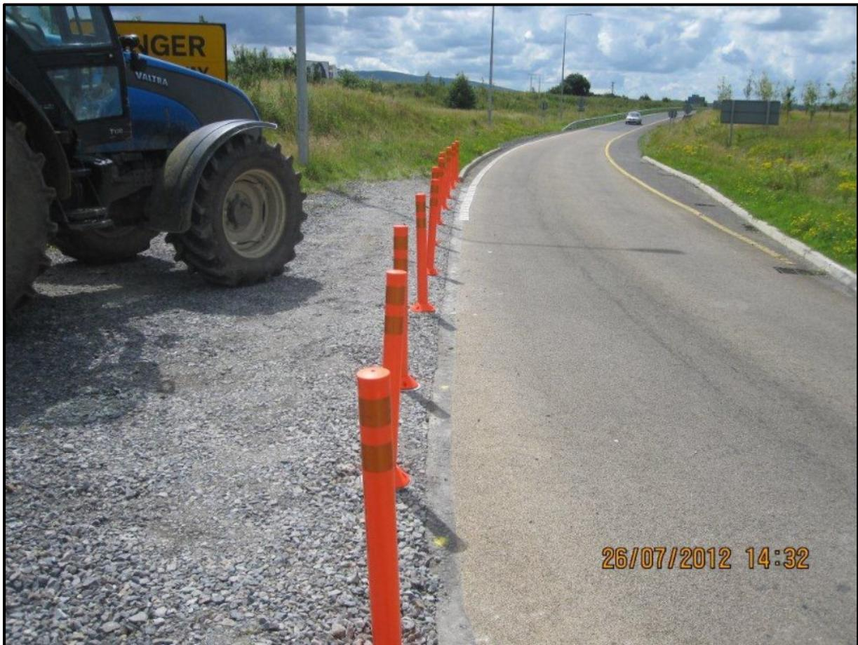
Figure 22: Example of temporary road widening along an off-ramp.
