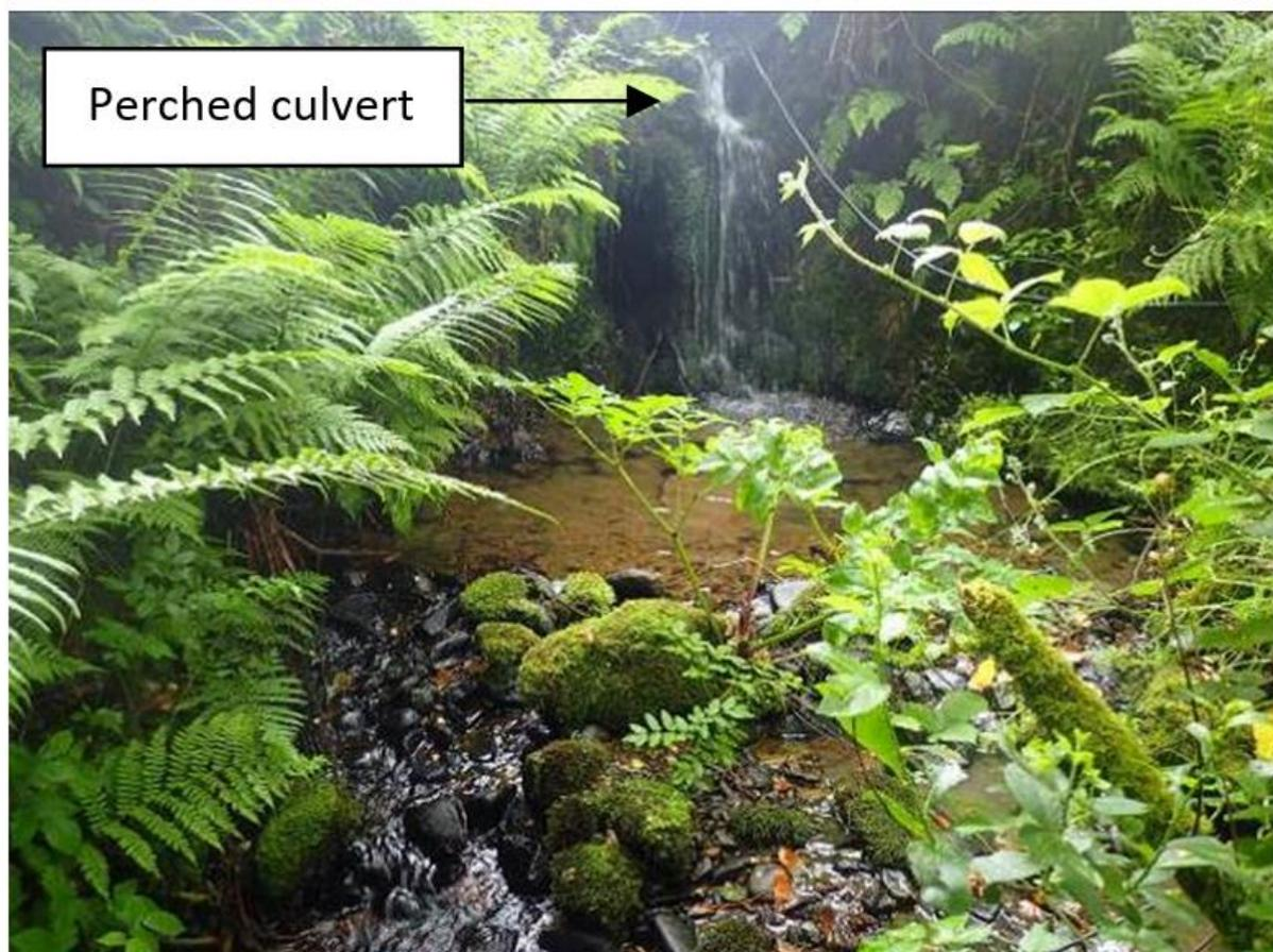
**Plate 8. A perched culvert that likely limits the upstream passage of trout located at Site 2 on the 1<sup>st</sup> Order Glennagross Stream, a tributary of the Crompaun Stream.**
