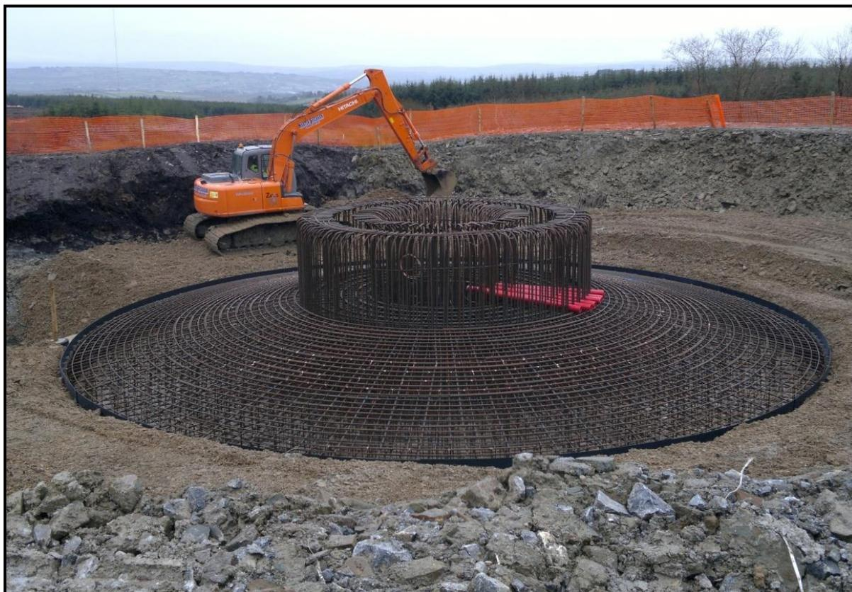
Plate 9. Typical construction of a wind turbine base.
